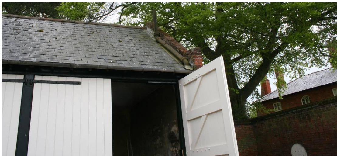
A stink pipe is laid on the roof.
