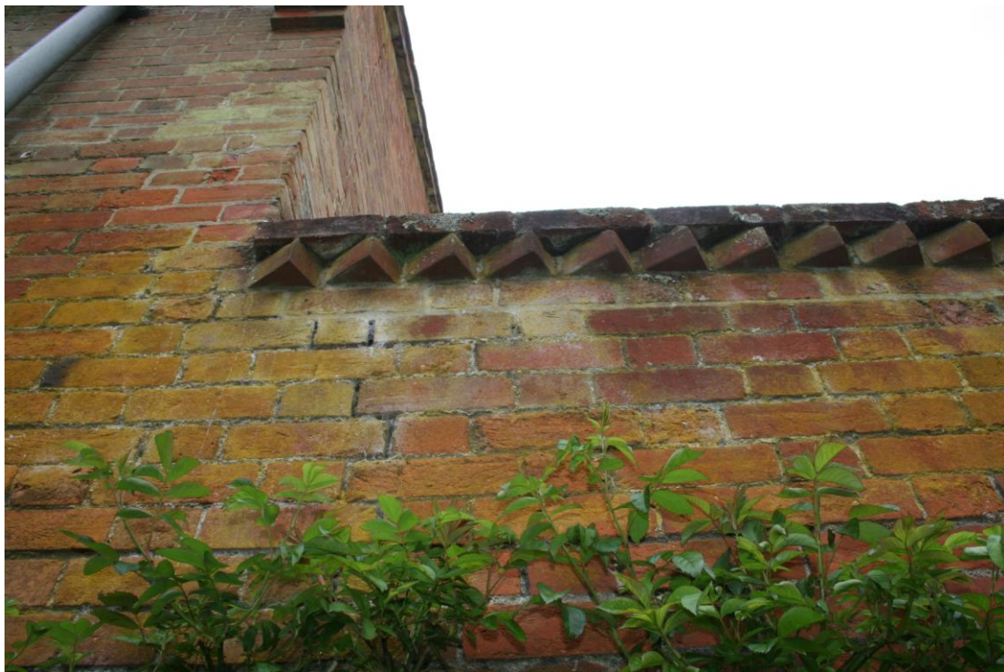
Detail of the of the herringbone dentillation.
