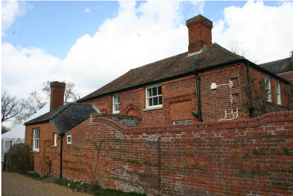
The SW elevation has a number of added 'offices'.
