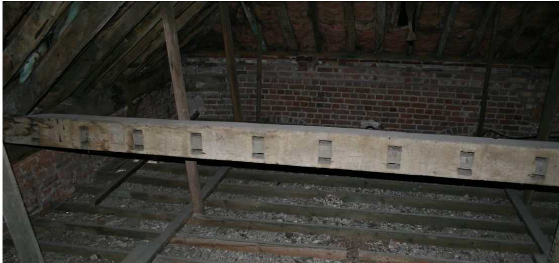
Detail of the tie-beam over the Stable.
