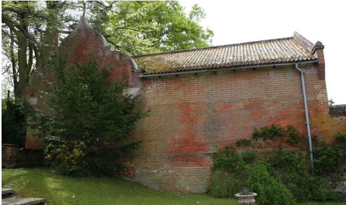
The NE elevation comprises three brick builds.
