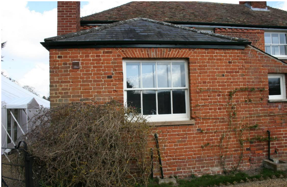
The SW elevation of the extension to the cottage.
