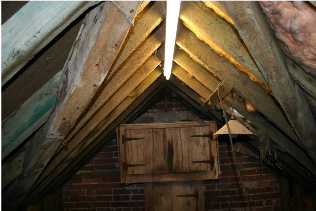
Looking SE at the clock gable roof structure.
