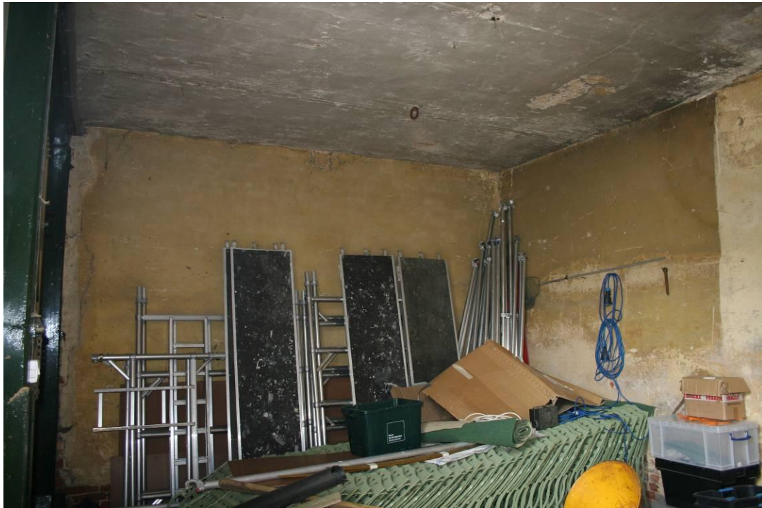
Looking NE inside the Car Port.
