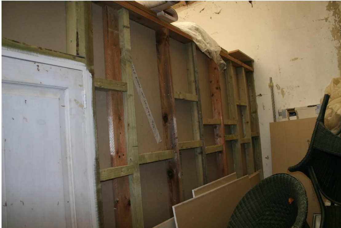
Modern studwork for the wedding reception rooms.
