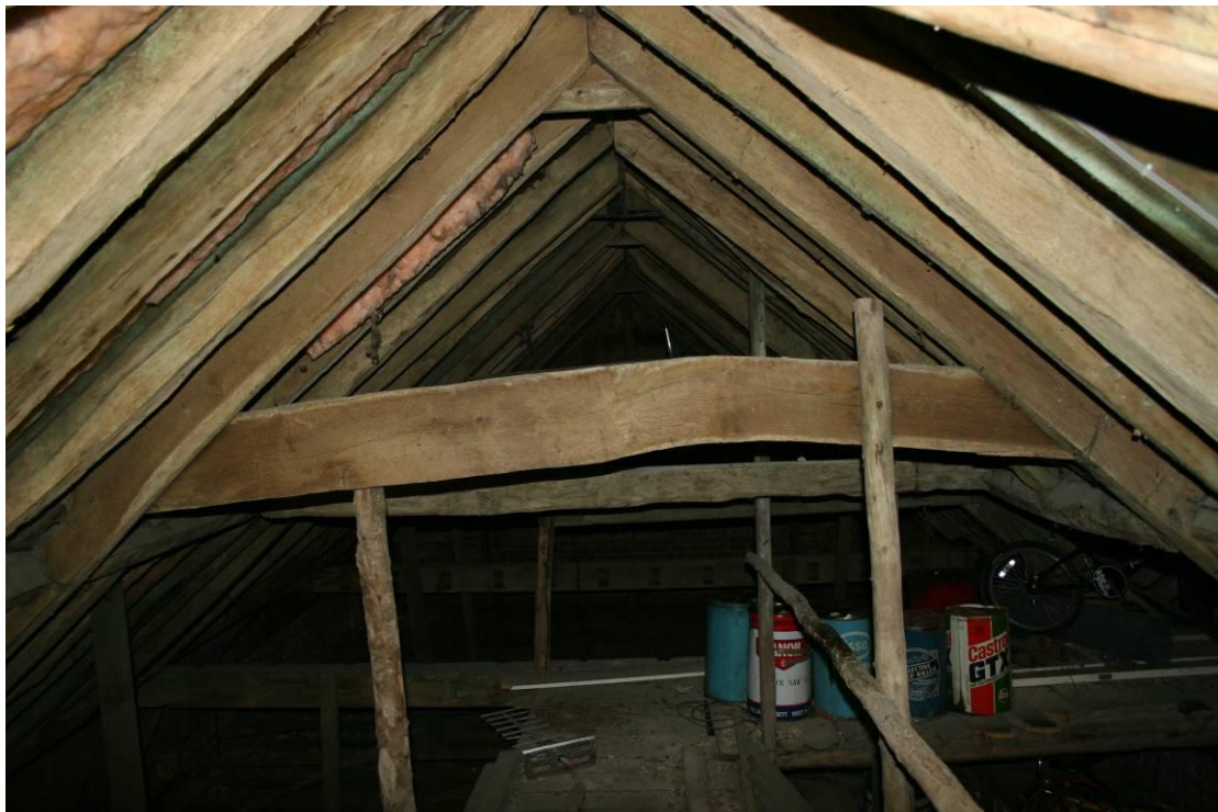
Looking SW along the roof over the clock gantry.
