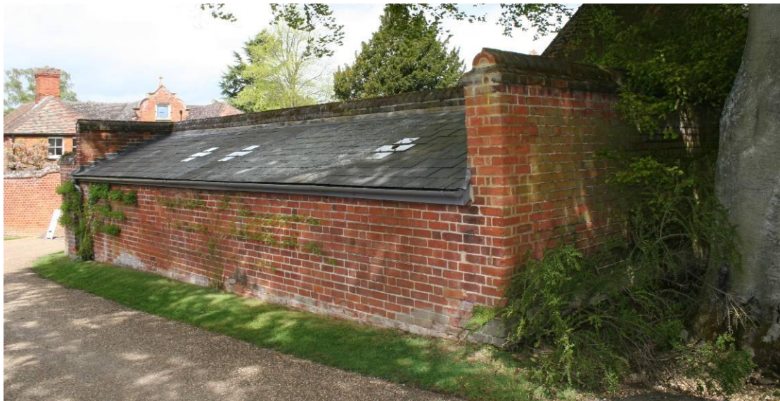
The junction with the perimeter wall. Looking N.
