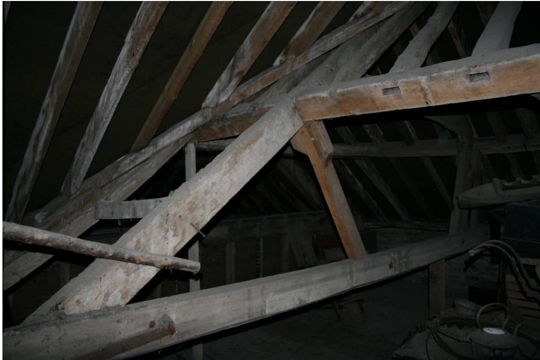
The roof structure over the Stables.
