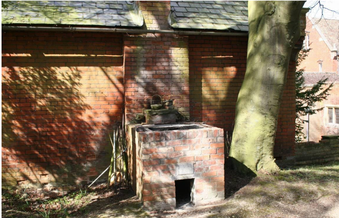
The modern incinerator has been ducted into the NE chimney stack.
