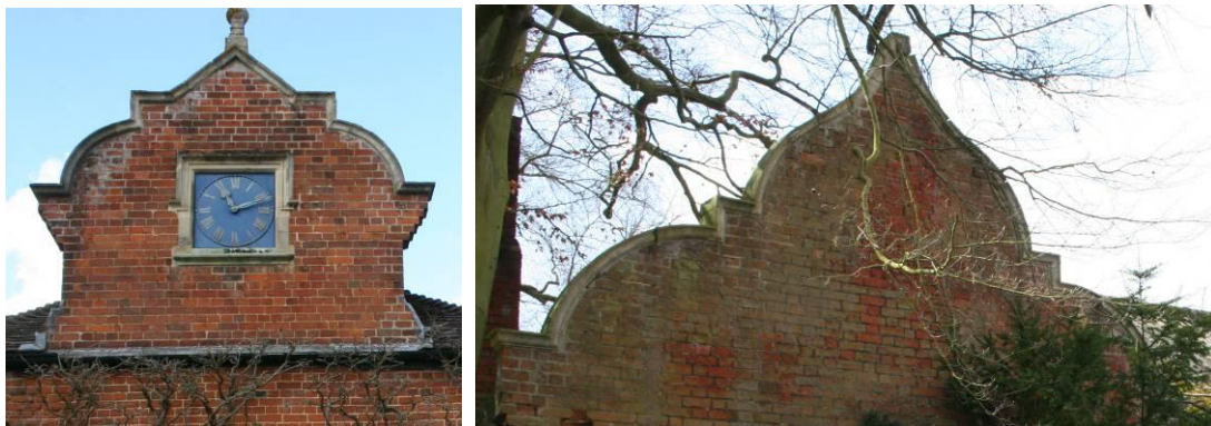
The clock gable compared to the gable of the Squash Court.
