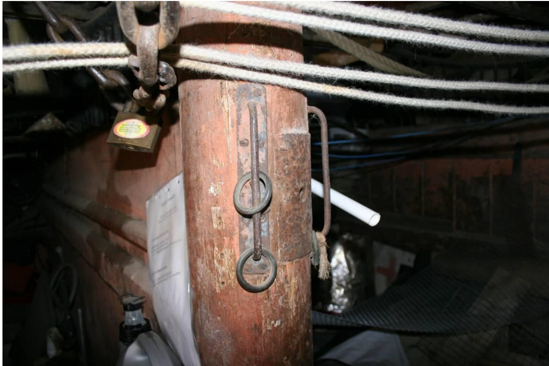
Mild steel sliding tethering rings.
