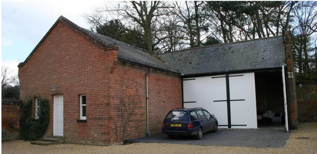
The NW elevation of the Squash Court.
