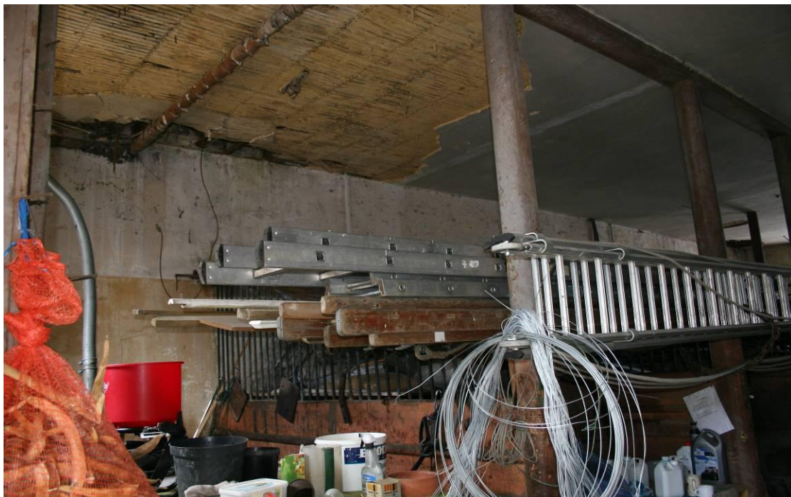
Looking SW up at the ceiling above the first stall.
