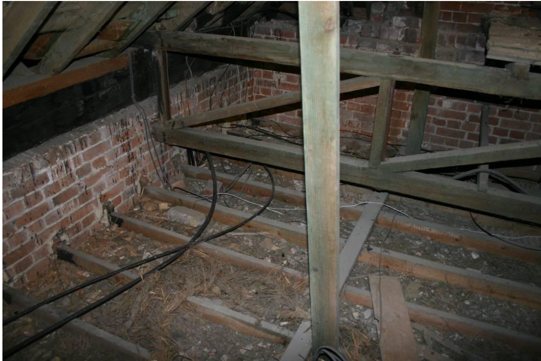
The machined timber supports for the gantry.
