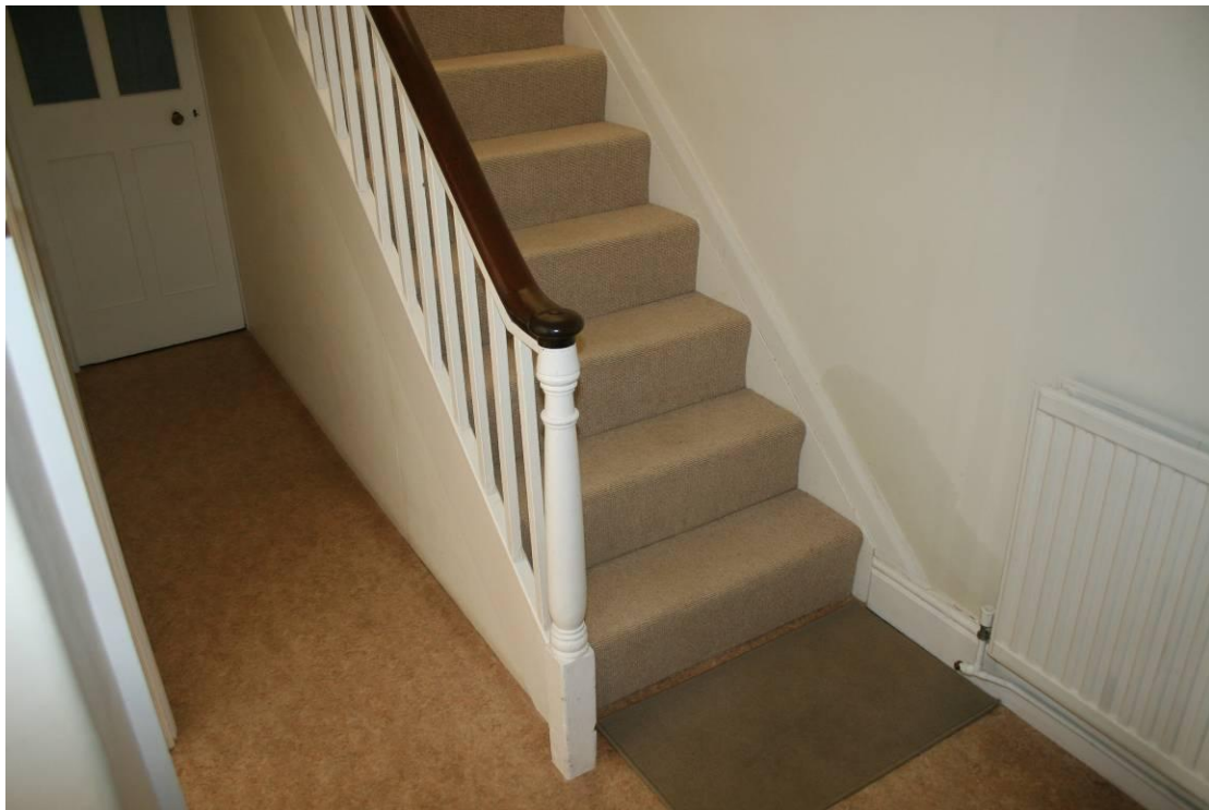
The C19th style staircase with turned newel post and stick balusters.
