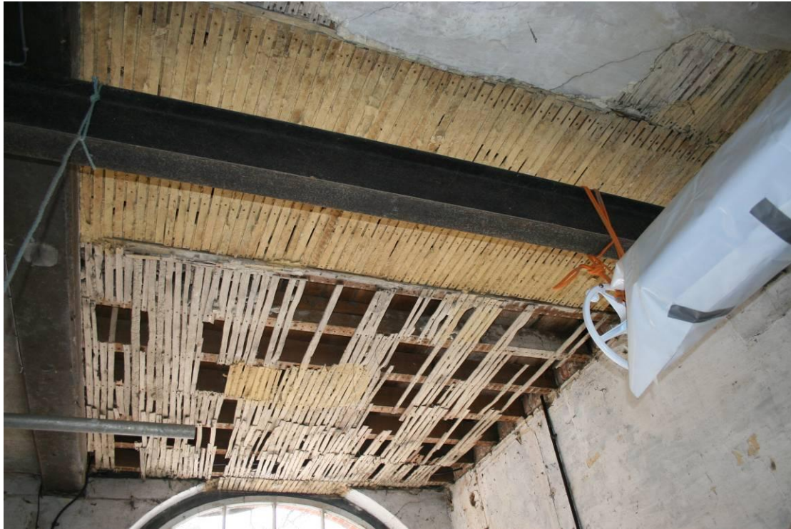
The ceiling above the Garage near the main doors. Looking E.
