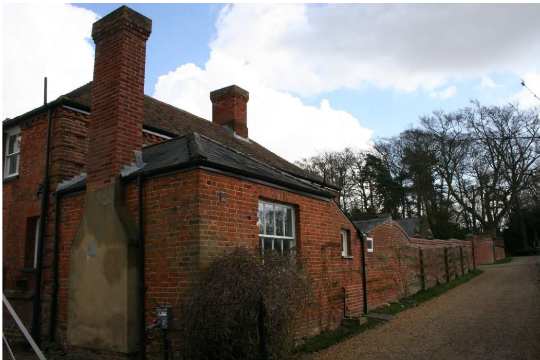
The NW and SE elevation looking E.
