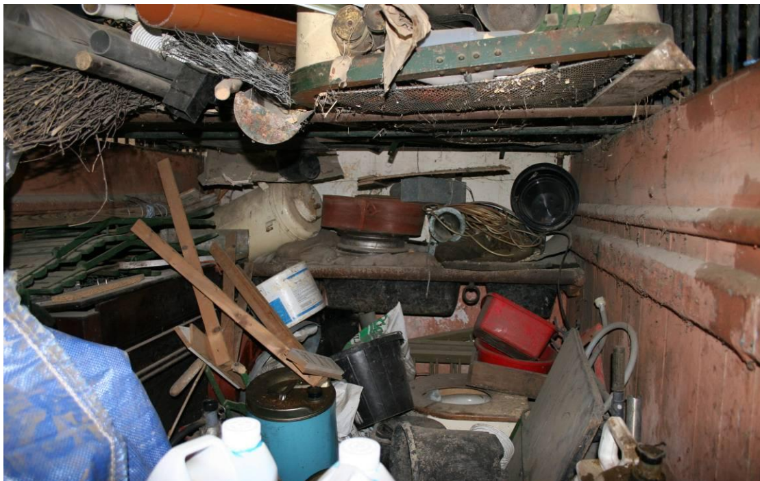
Looking SW in Stall 3 at the cast iron feed and water trough with tethering ring.
