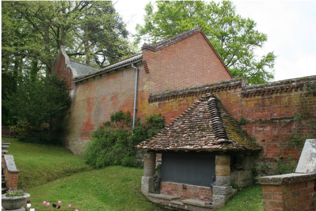
The perimeter wall continues along the sunken garden.
