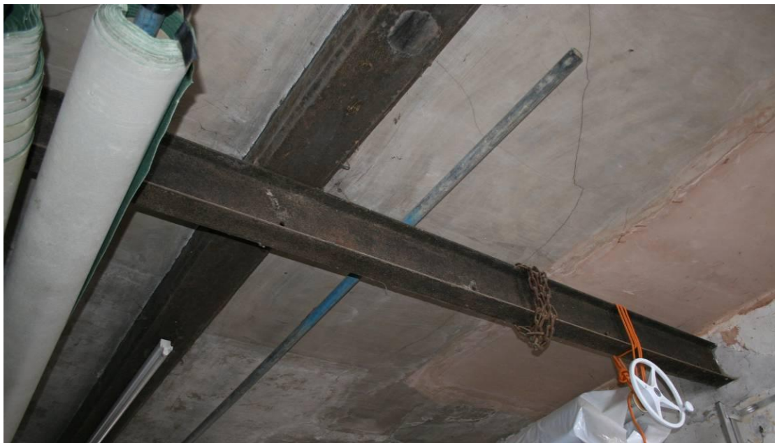
Detail of the steel beams.
