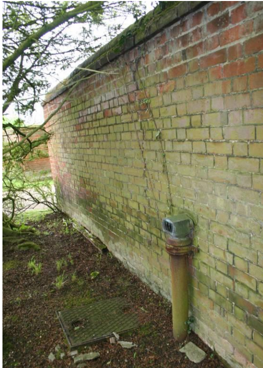
The exterior of the perimeter wall looking SW.
