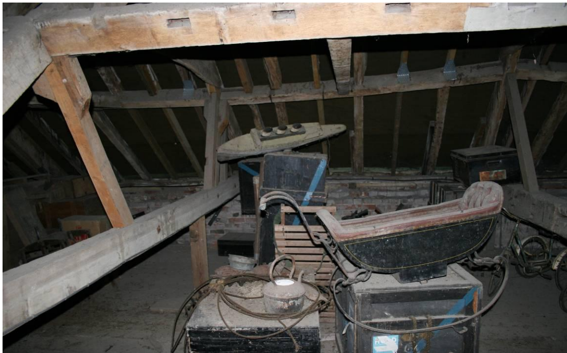
Looking N into the Garage loft space.
