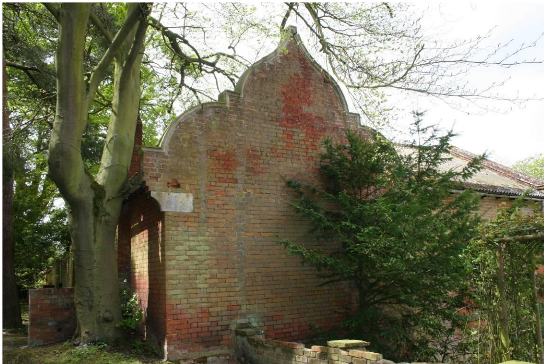
The NE elevation has an ornate ogee gable.
