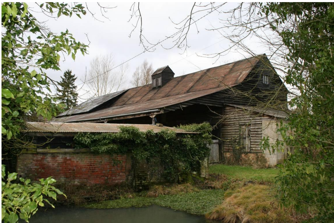
The corrugated iron roof of the East Frame.
