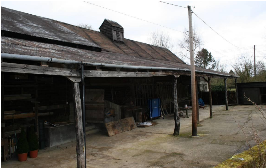
The Open Shelter looking NE.
