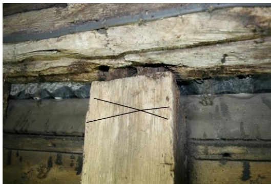
Stud marked with an X in the West Frame.
