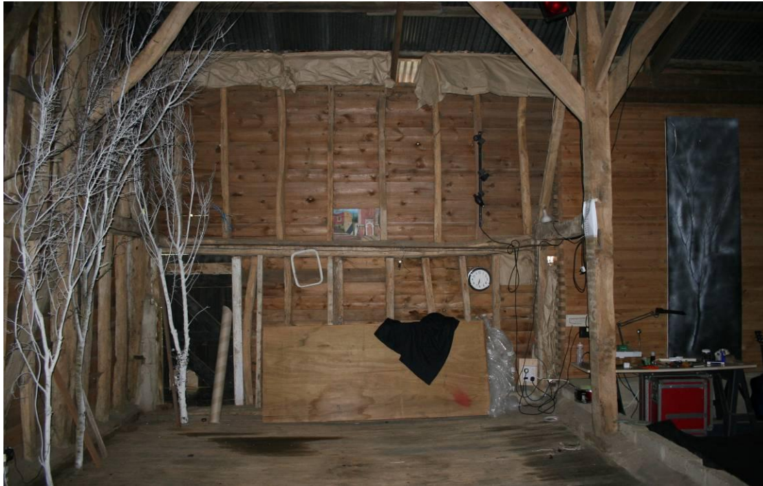
The southern side of Bay 5. The boarded floor appears LC19th.
