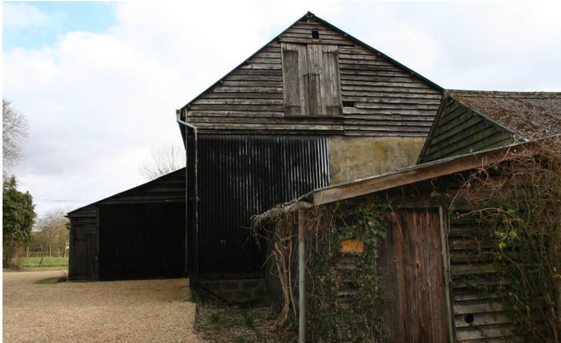
The Pre-dresser, the Barn and the Workshop looking E.
