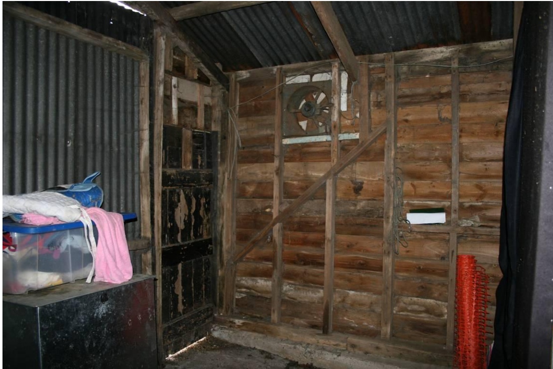
The western room of the Pre-dresser.
