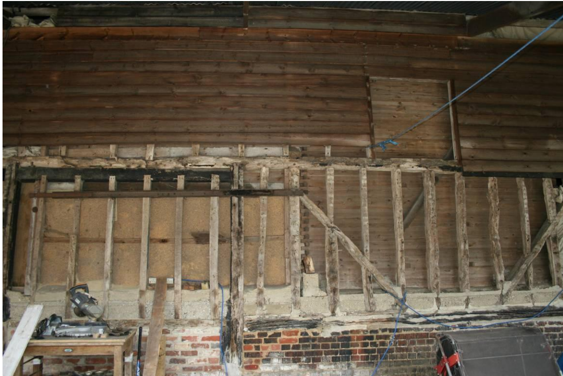
Bays E3 and E4. Bay E3 has been rebuilt with side nailed studwork.
