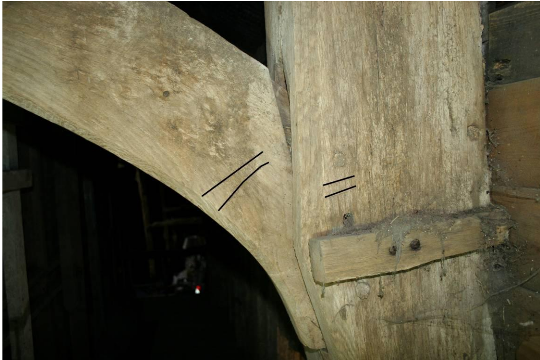
The West Frame storey post and brace is marked II.
