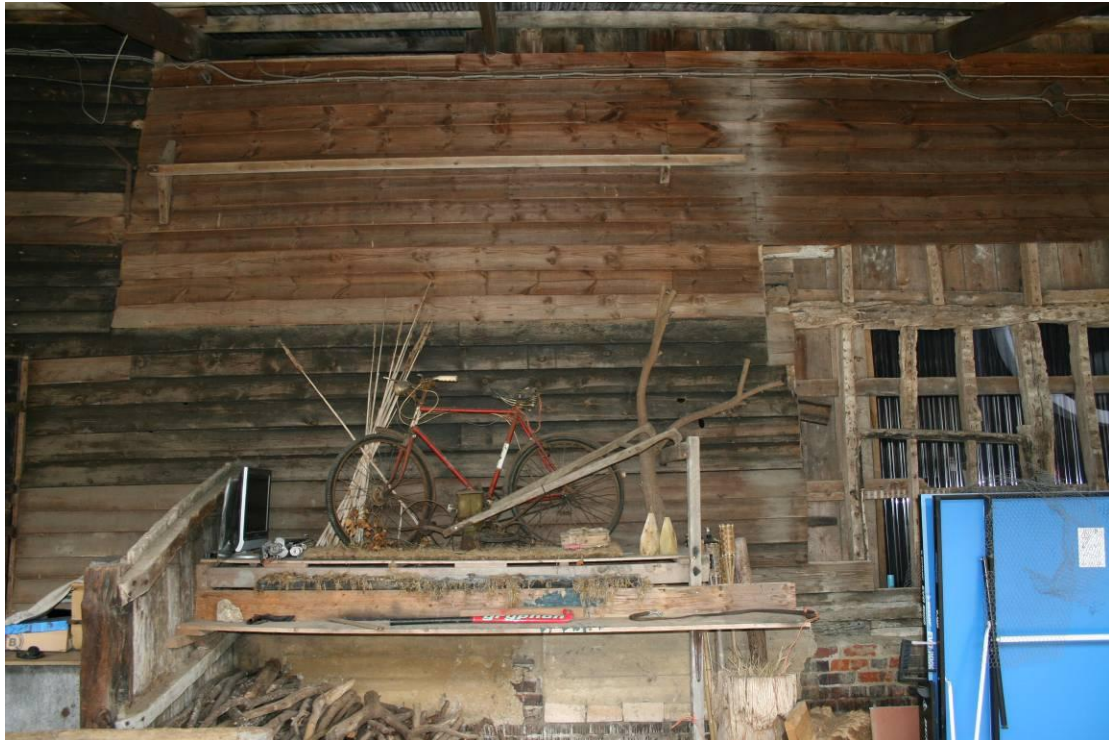
Bay E1 has been largely reclad with new boards.
