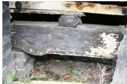
Detail of the suspended timber floor.
