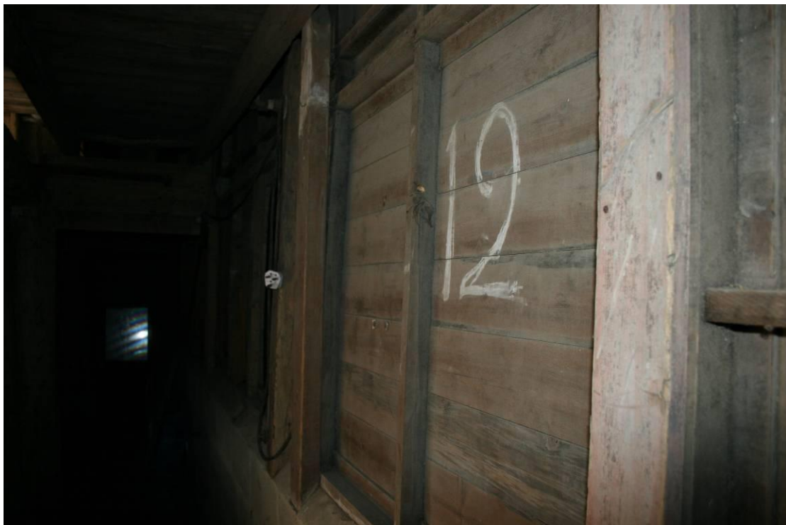
The silos were built inside the West Frame.
