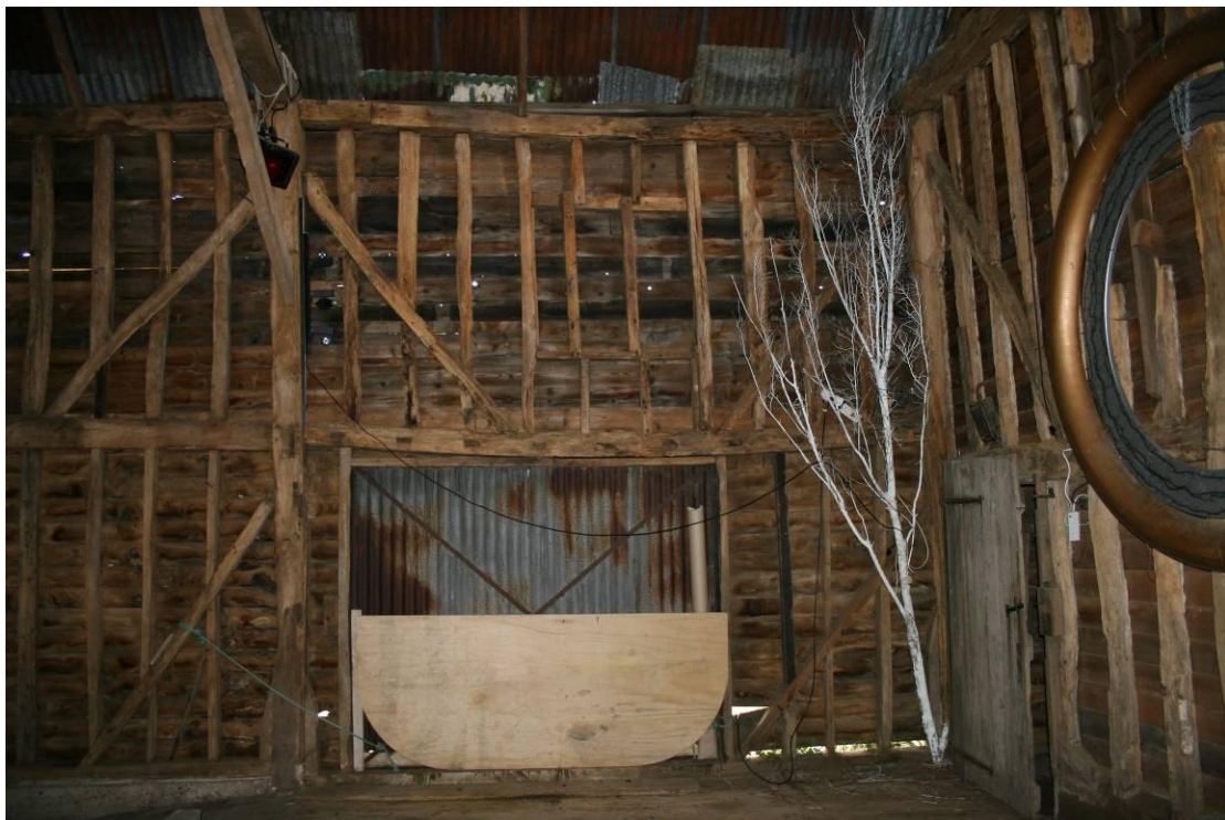
The northern side of Bay 5.
