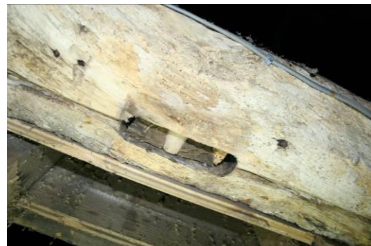
Rounded mortice and wattle groove.
