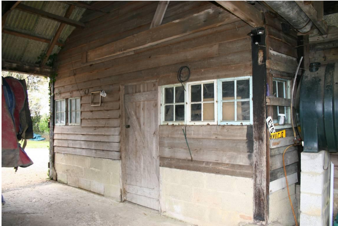
The garage workshop under the carriage arch. Looking NW.
