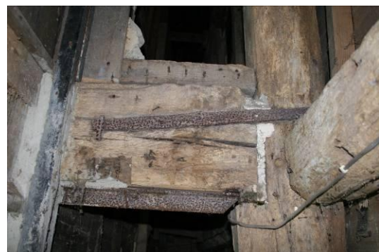
C.1800 iron tie reinforcing the floor joist.
