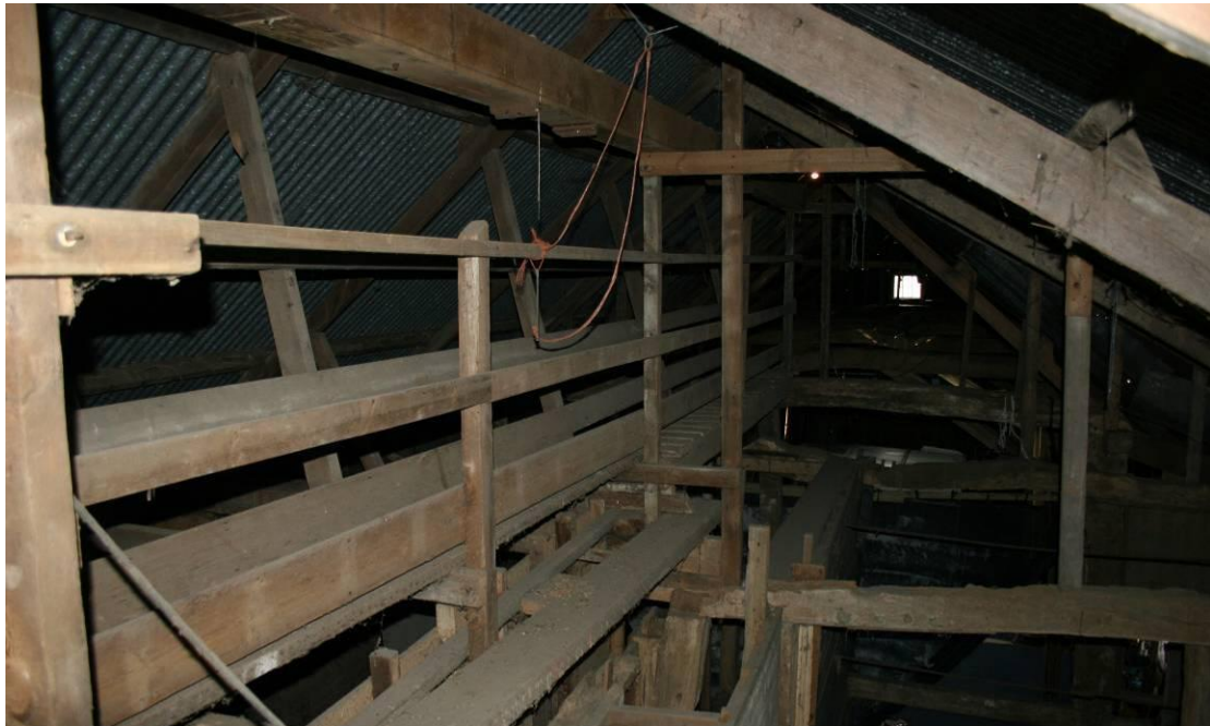
Looking E along the upper gantry. The box channel above contains the chain drive.
