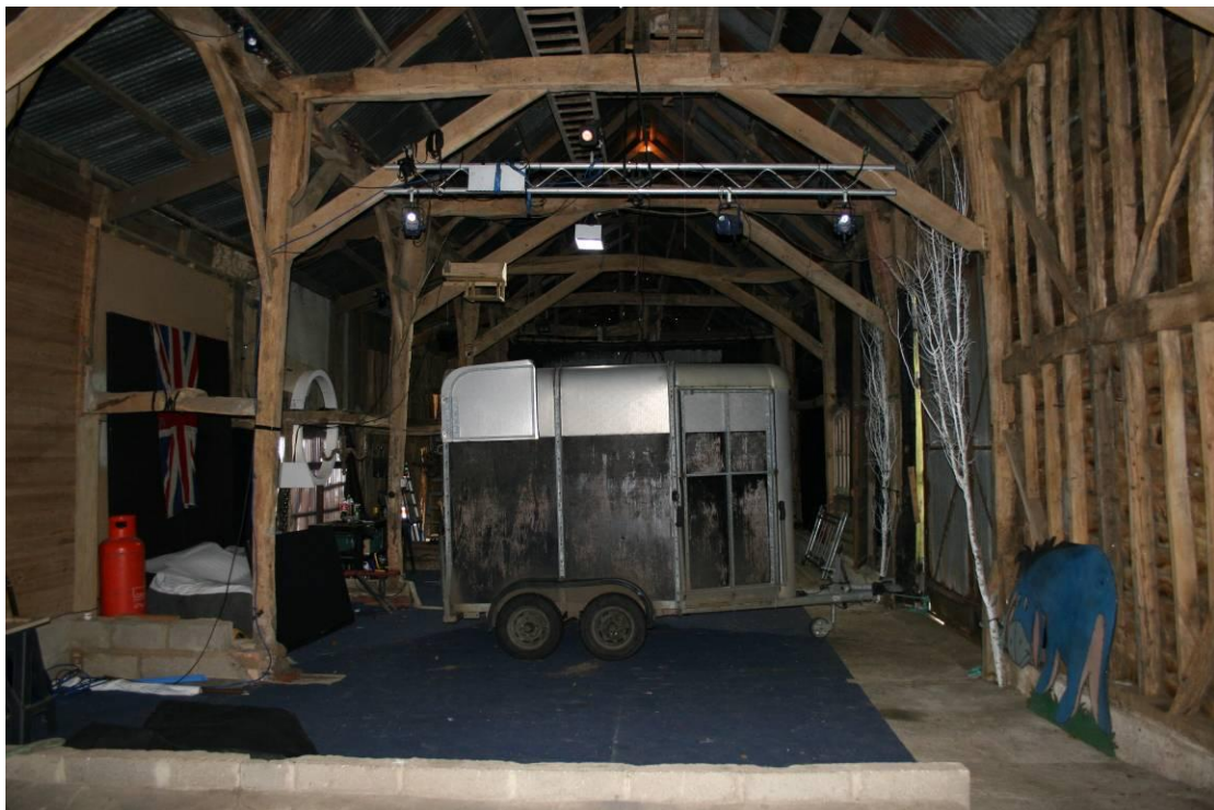
Looking W inside the East Frame.
