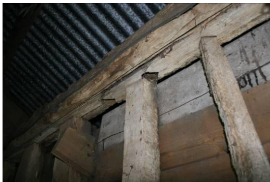
There is evidence for two mullioned windows in the southern wall.
