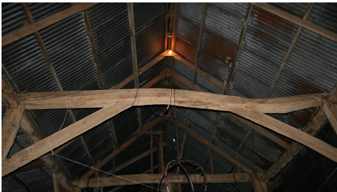
The roof structure over the East Barn looking W.
