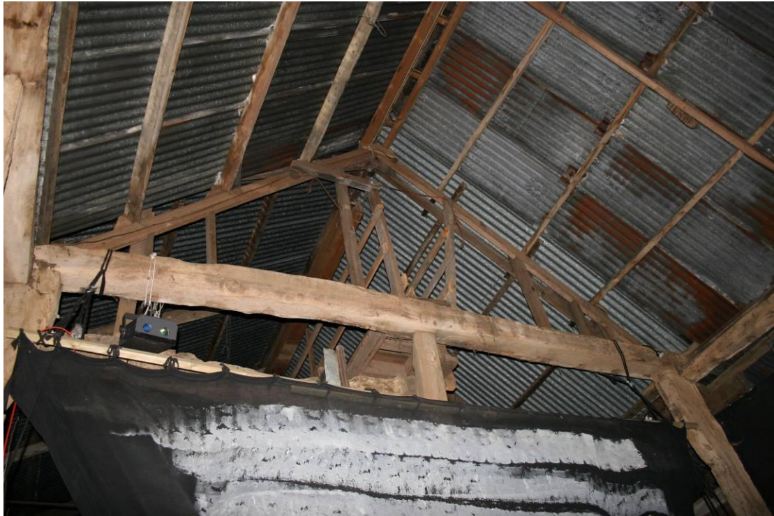
The roof structure over the West Frame. Looking W.
