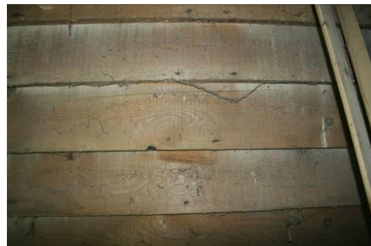
Detail of the LC20th weather-boarding.
