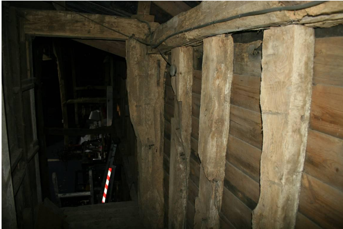
Trenched studwork in the southern wall.
