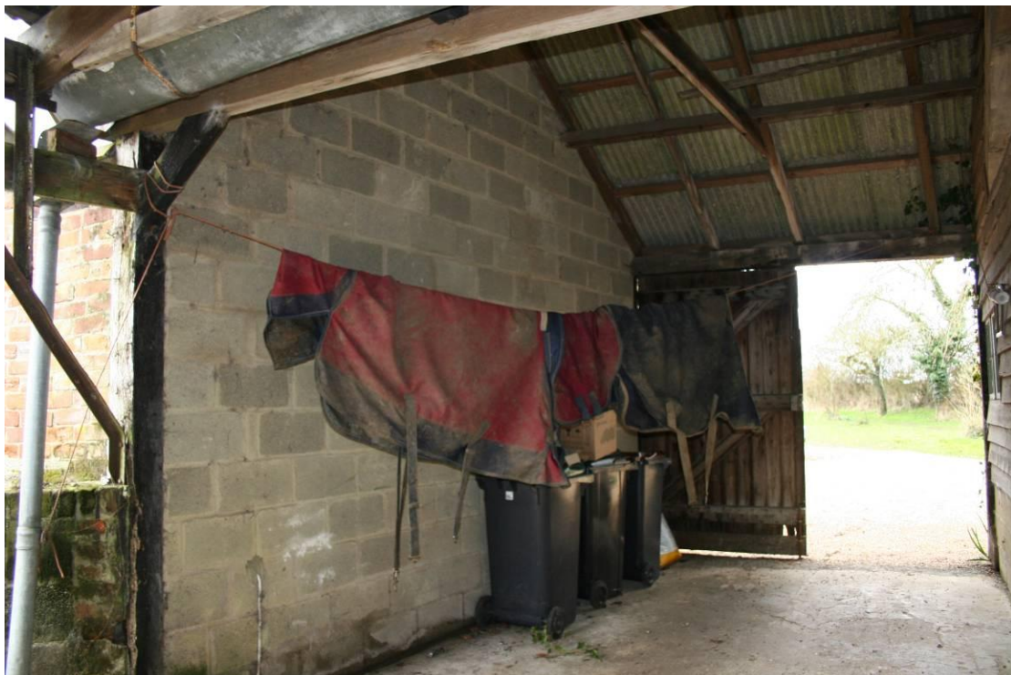
The House side of the carriage arch is made of blockwork.
