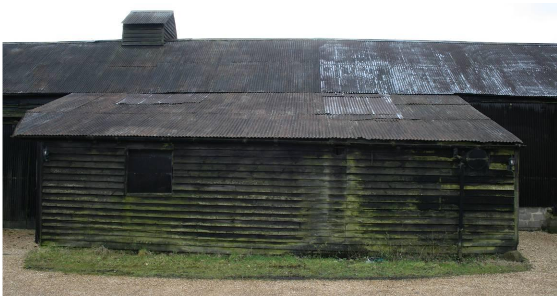
The Pre-dresser, north elevation.
