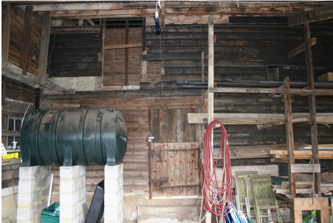
The southern elevation of Bay W1 in the West Frame.
