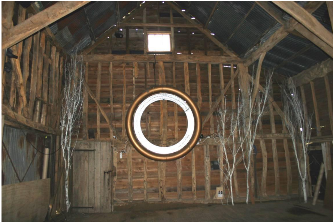
Looking E at the eastern wall of the East Frame.
