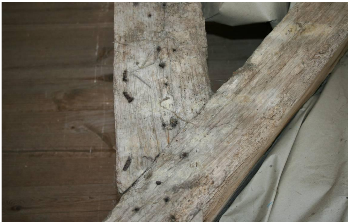
Interrupted stud nailed to the primary brace and numbered V.
