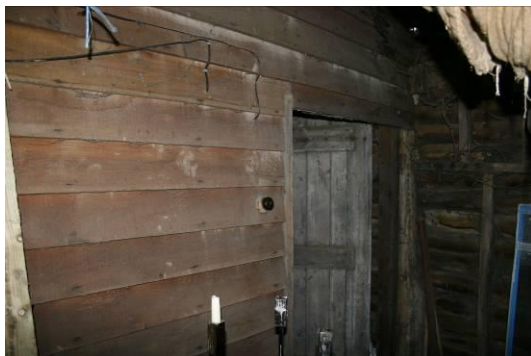
The entrance door from the Barn.
