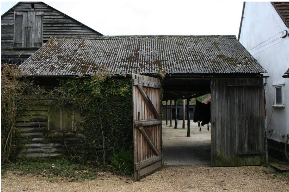
Detail of the garage workshop.
