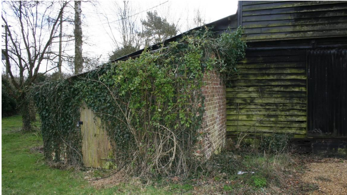
The Drier Motor House looking SE.
