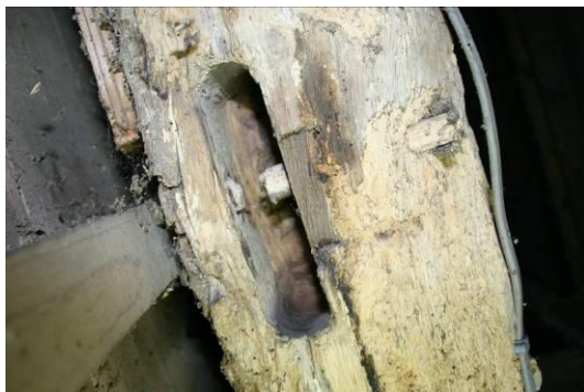
Rounded mortice with original peg.
