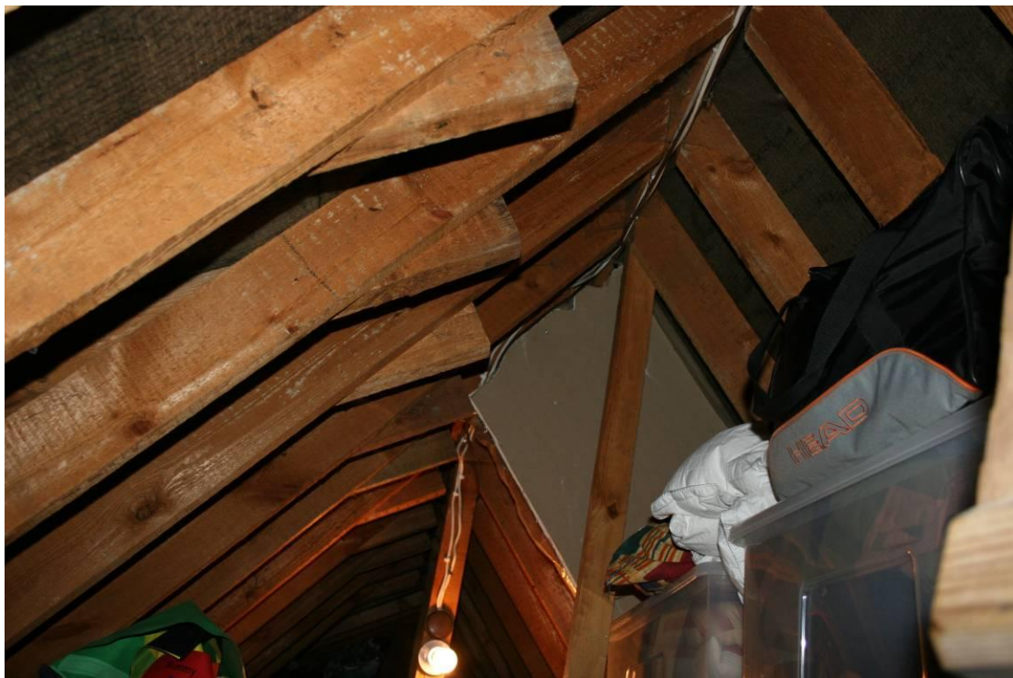
The modern roof structure above the bedroom.
