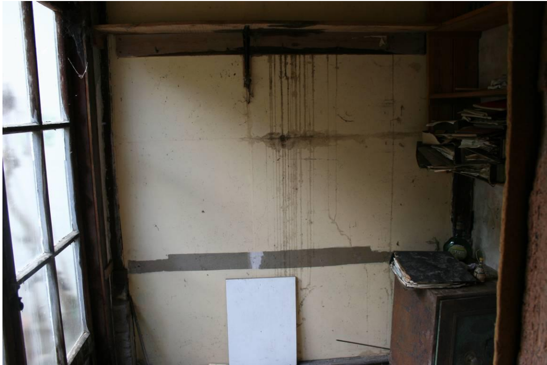
The alcove beside the fireplace has a plasterboard wall.
