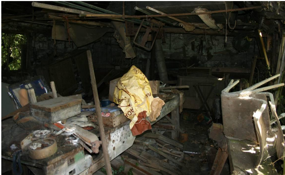
Looking NE from the entrance to the Workshop.
