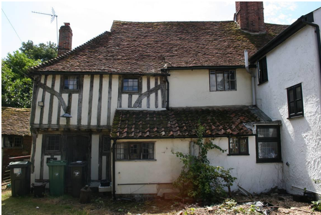
The northern elevation of the main range and cross-wing.
