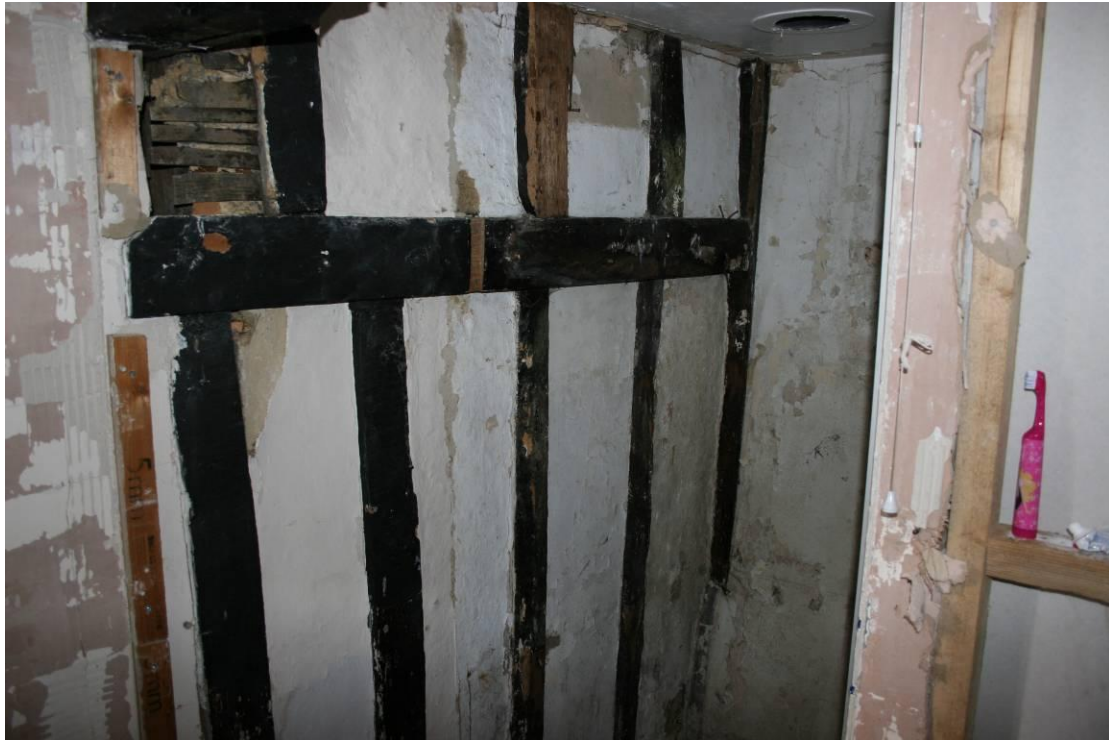
Studwork in the bathroom.
