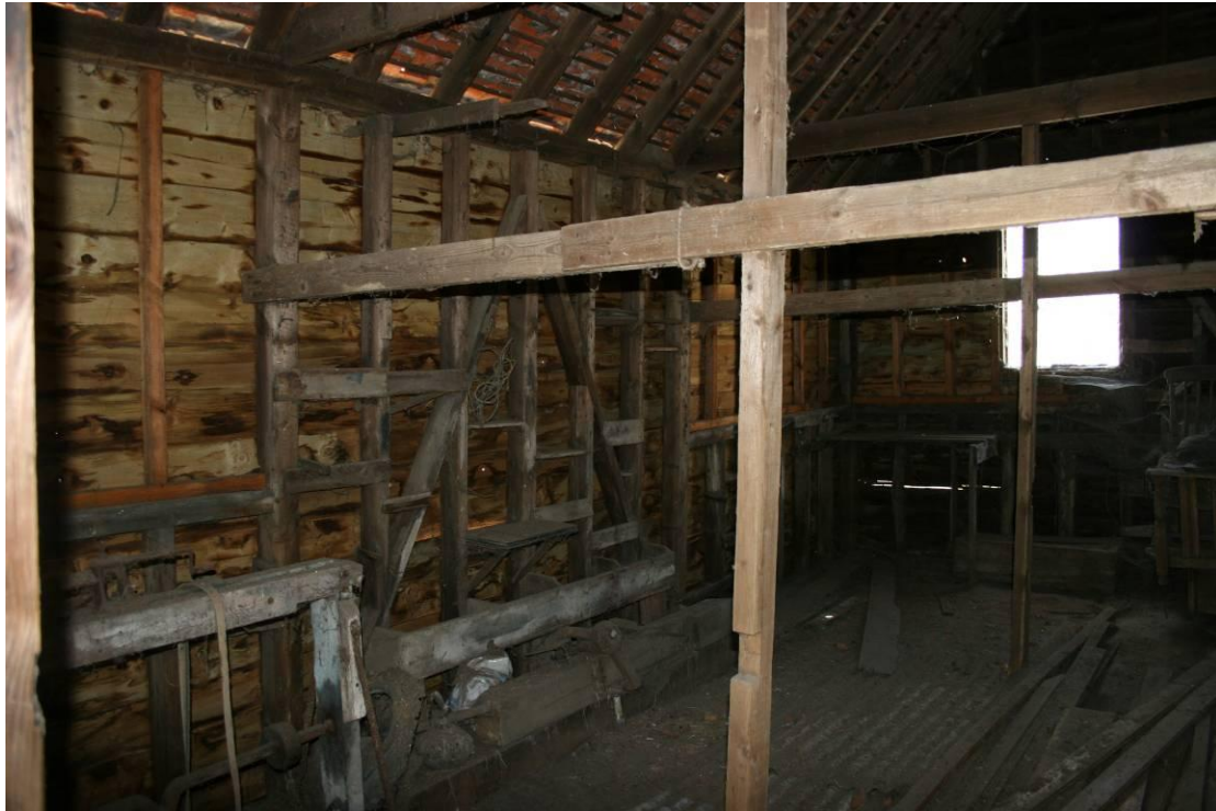
The Stables upper floor was used as a woodworking workshop.
