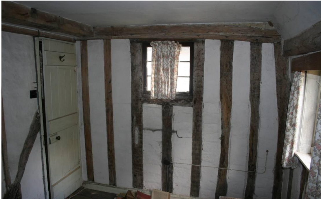
The cross-wing north bedroom looking N.
