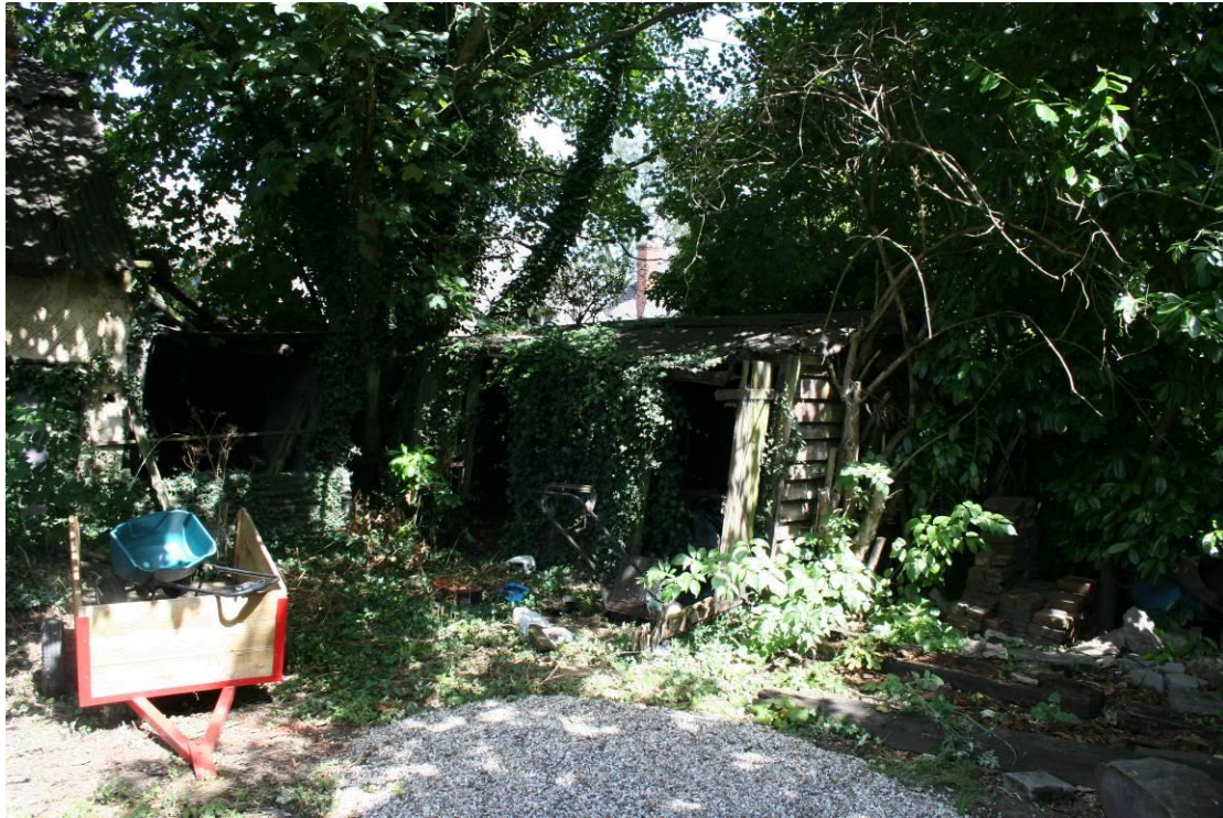
Store buildings. Looking NE.
