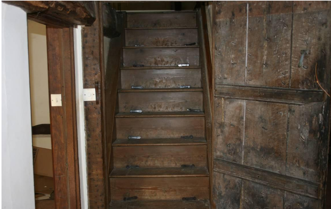
Detail of the EC20th staircase. Looking N.
