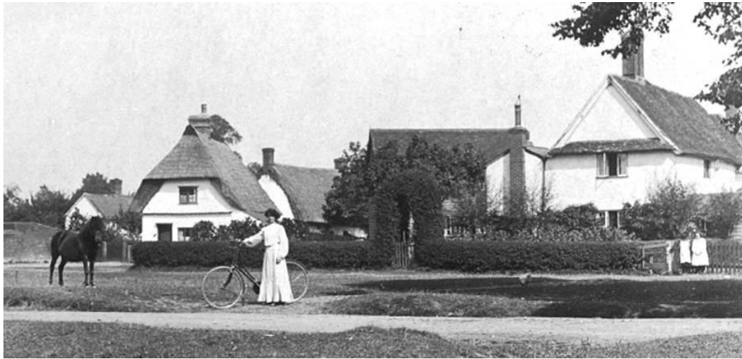
1907. Wyndies. Note the two storey extension.
