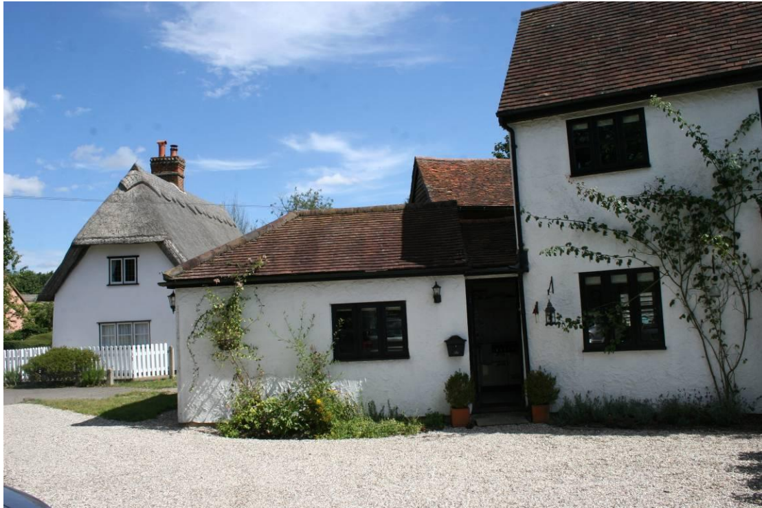
Southern elevation of the former garage.
