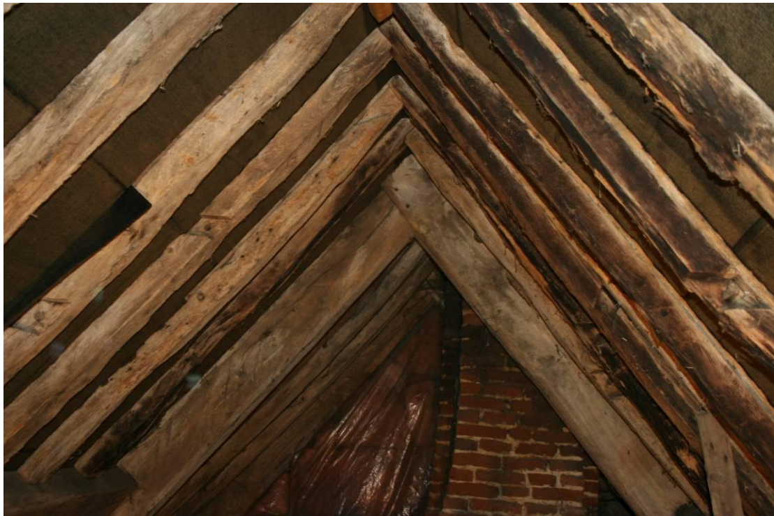
Reused sooted rafters from a hall roof.
