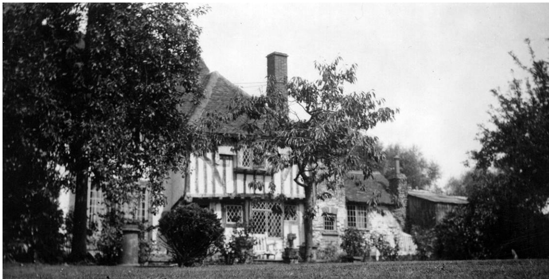
1930's. The south elevation with Mr Turner's windows.
