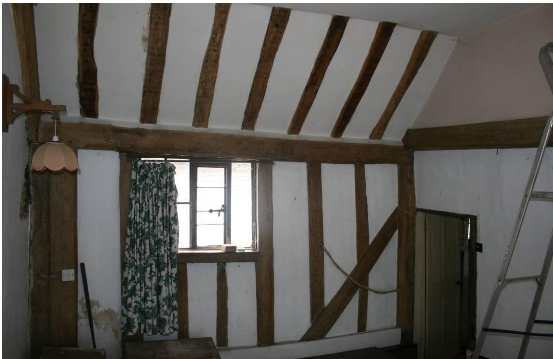
The exposed frame of the raised main range.
