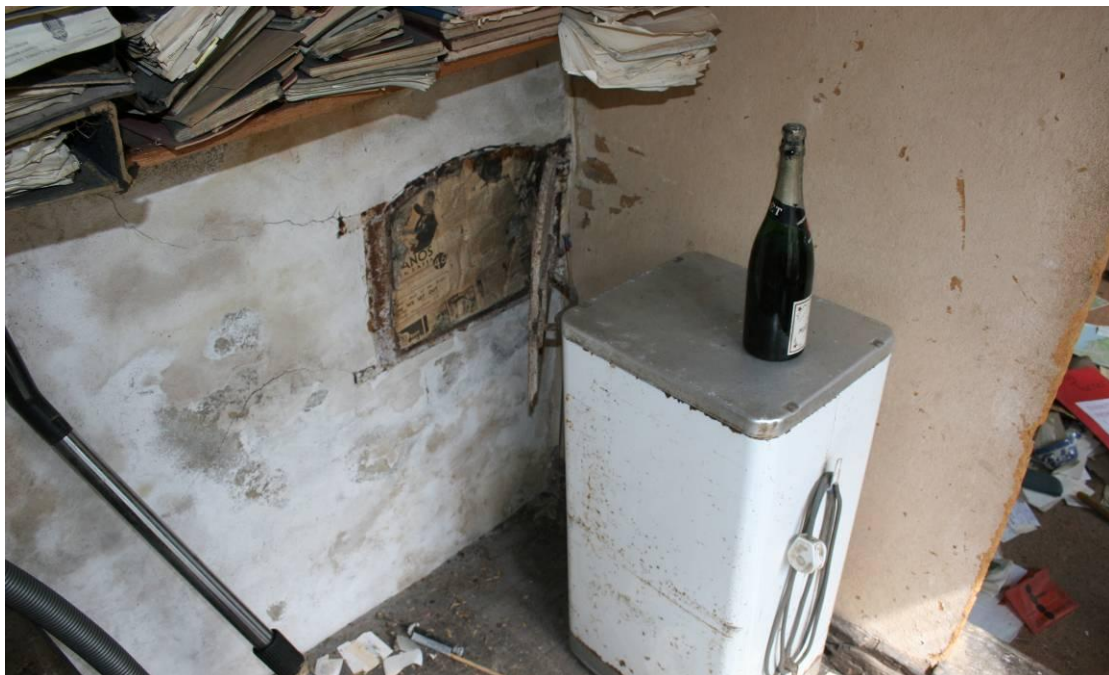
The bread oven door in the side of the firestack.
