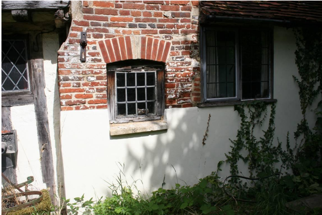
Base of the brick tower and Kitchen window.
