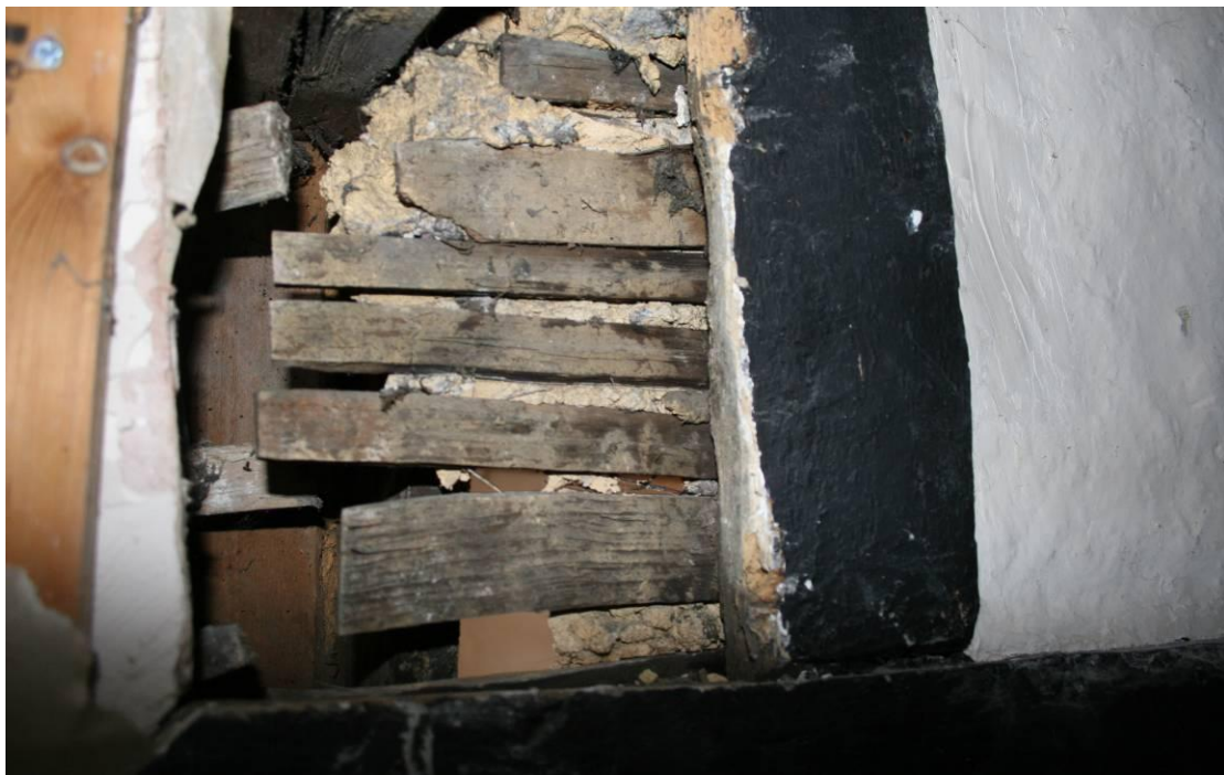
Detail of the lath and plaster.
