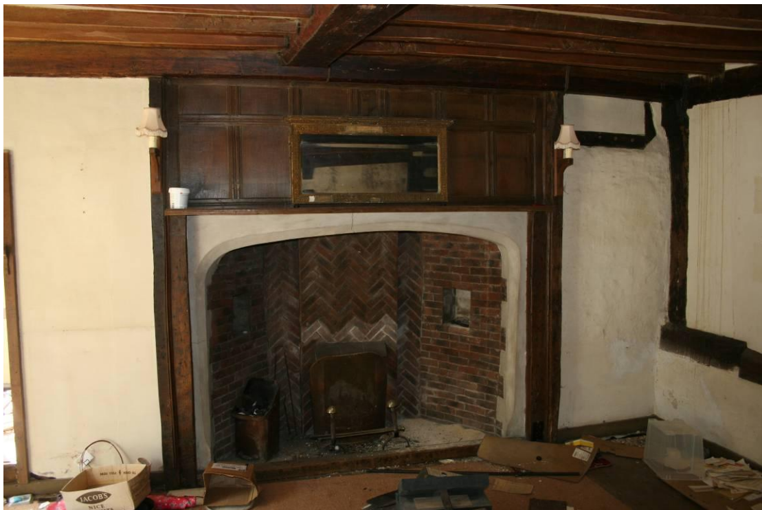
Replica fireplace and overmantel made of early panelling. The fireplace is tiled.
