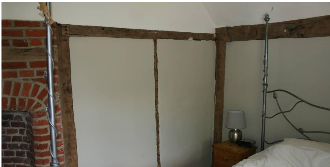
Original top-plate and partition wall by Mr Turner.
