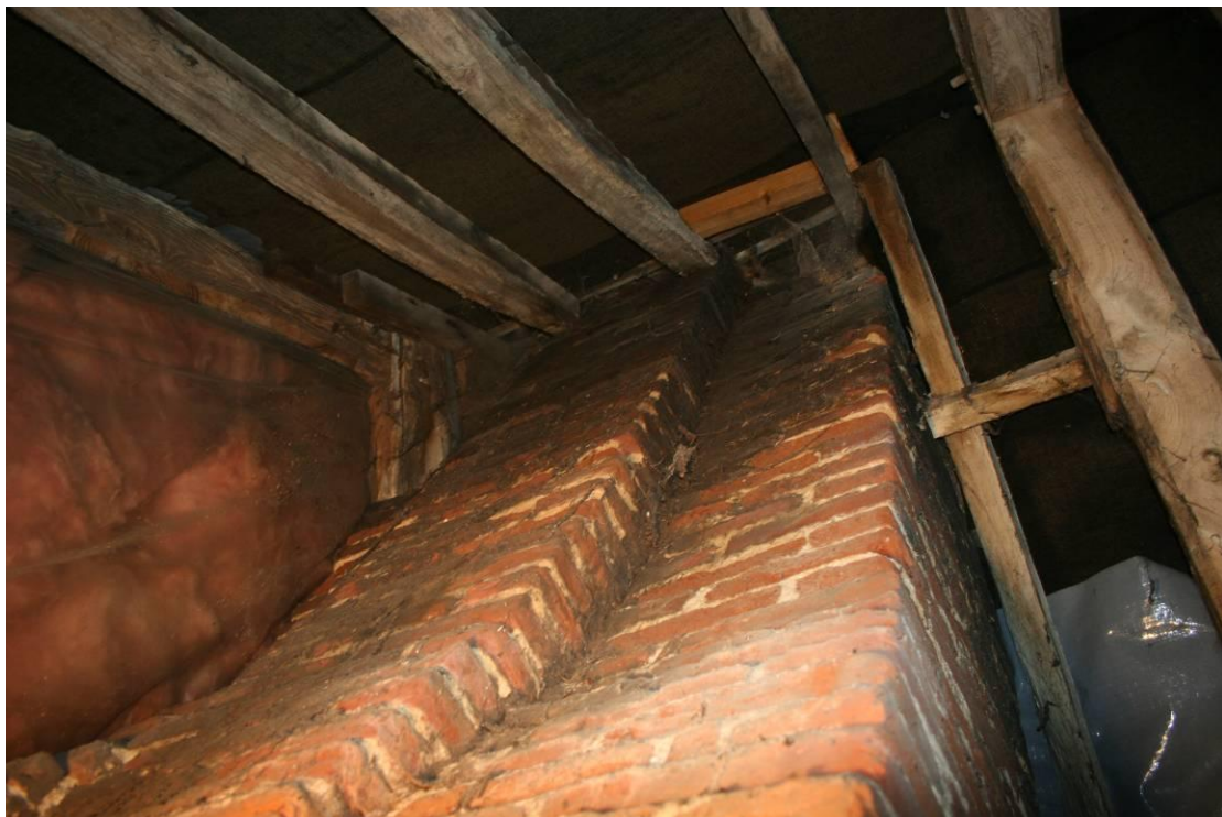
Looking up the firestack.
