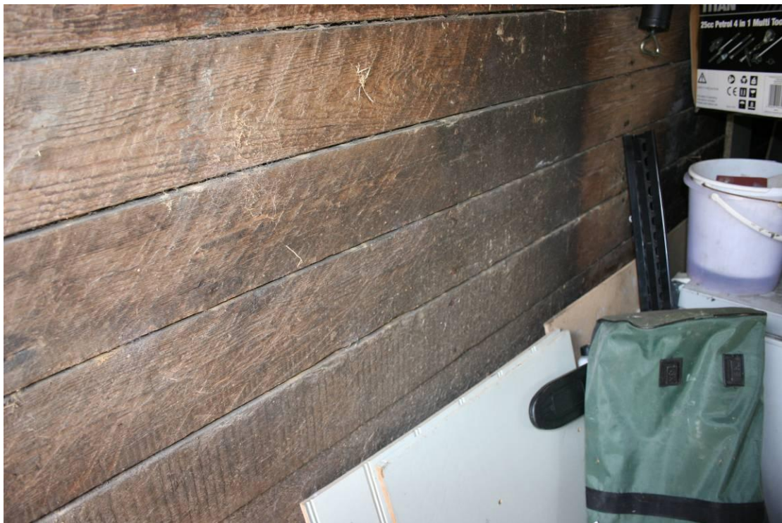
Detail of the machine cut kickboards.
