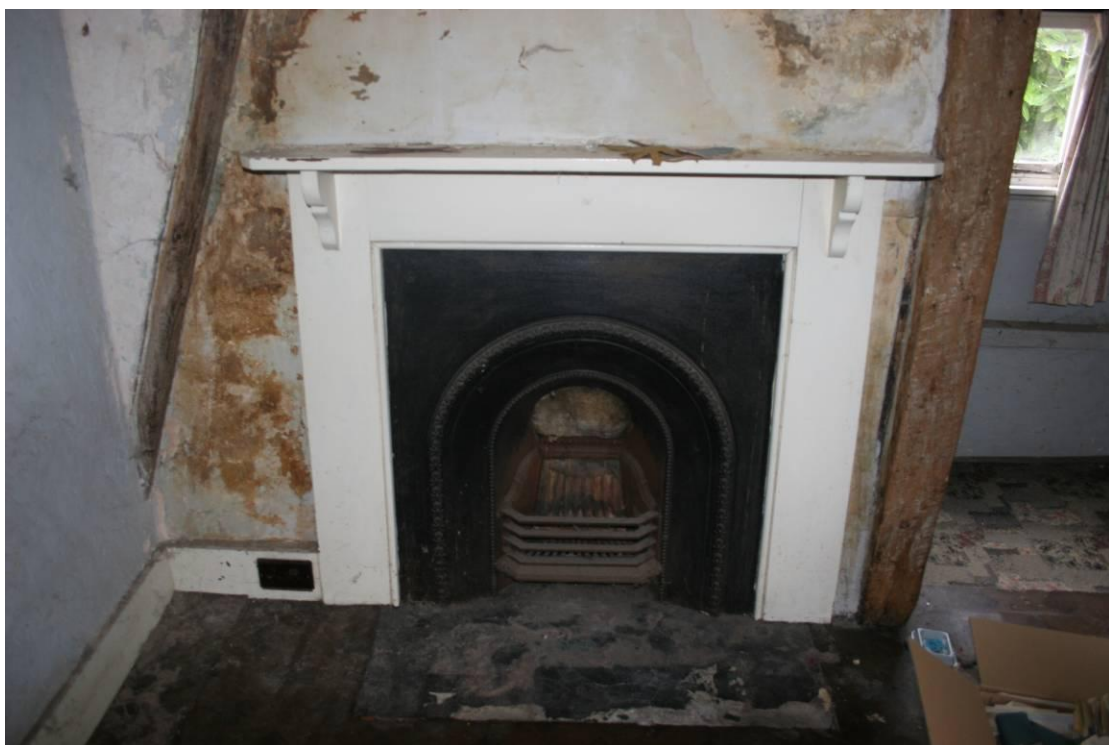
C19th cast iron fireplace with timber surround.
