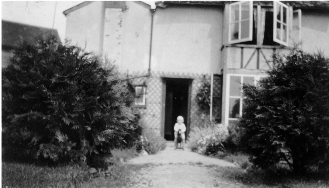
1930's. Note the plain casement windows.
