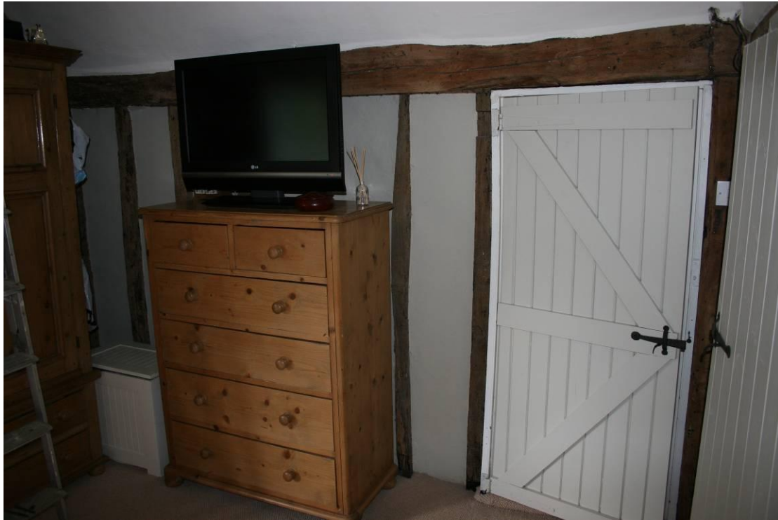
Wall common with the extension has some original studs.
