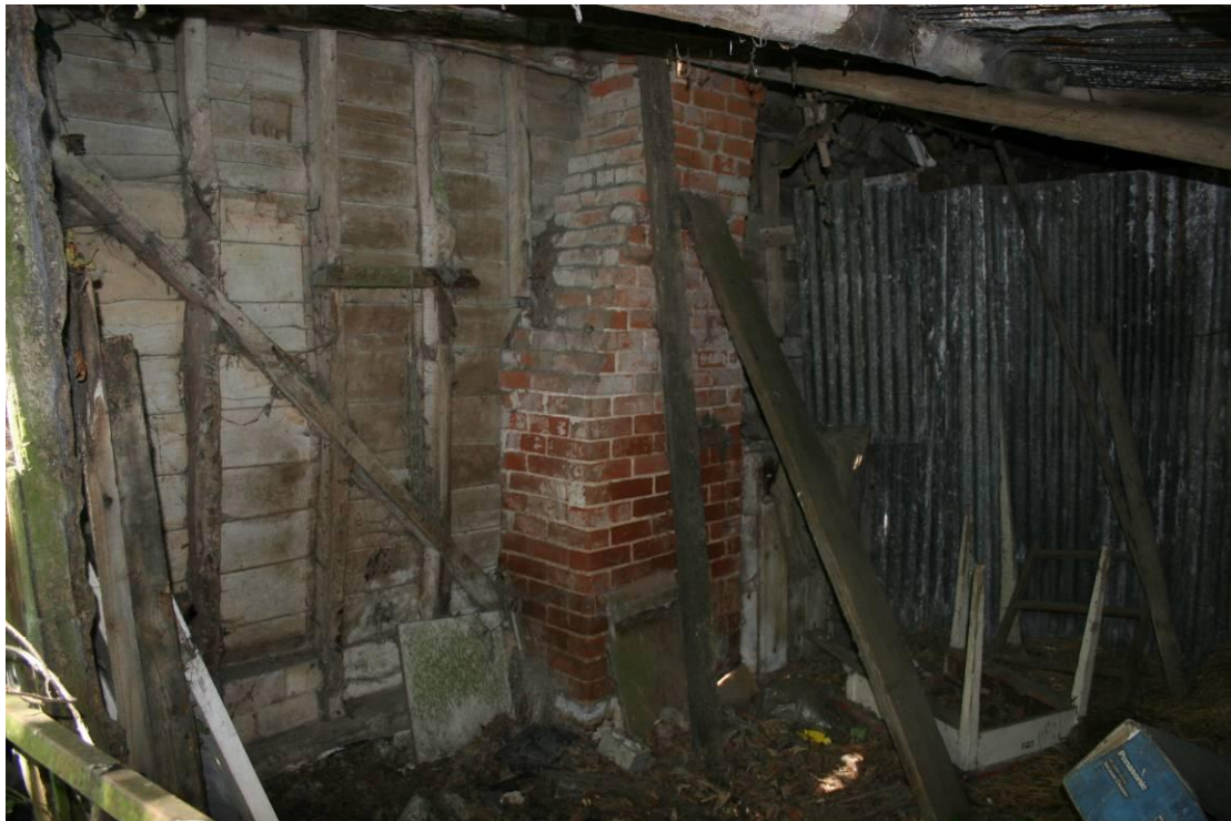
C19th chimney and nailed interrupted studwork seen in the tin shelter.
