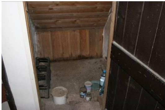
The underside of the staircase.
