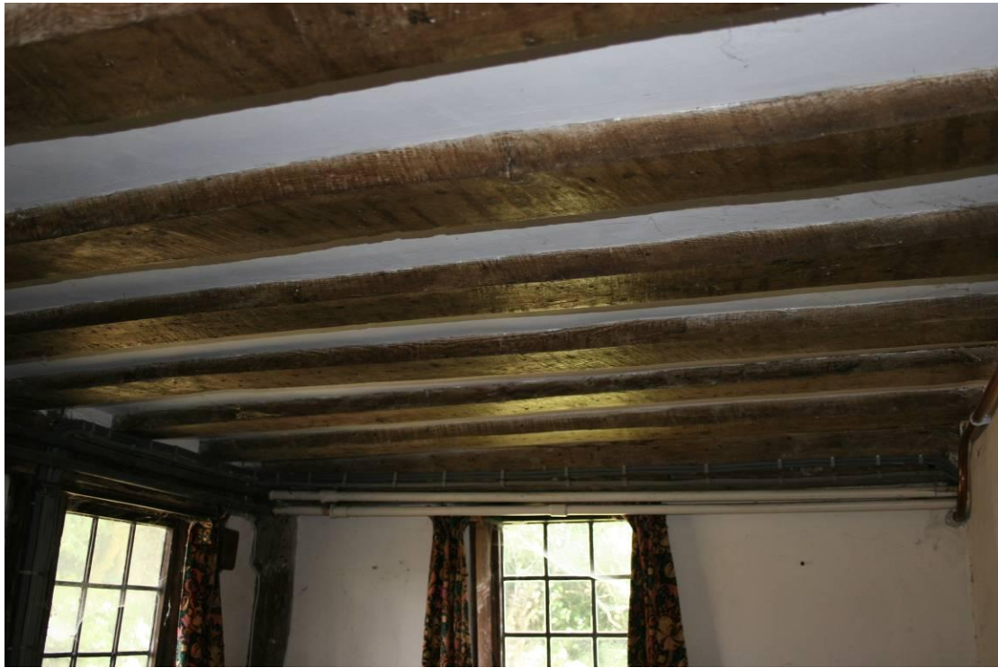
The framed floor in the Hallway.
