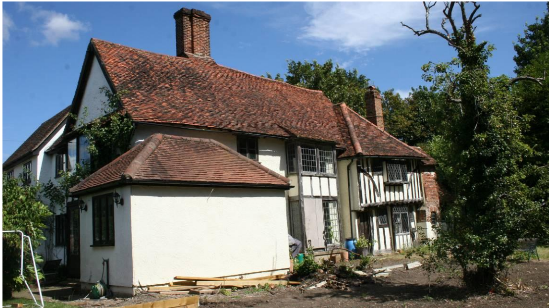
The west and south elevations.
