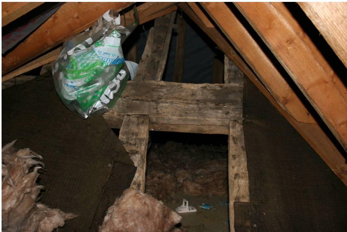
Continuation of the butt purlin roof seen from the modern extension.
