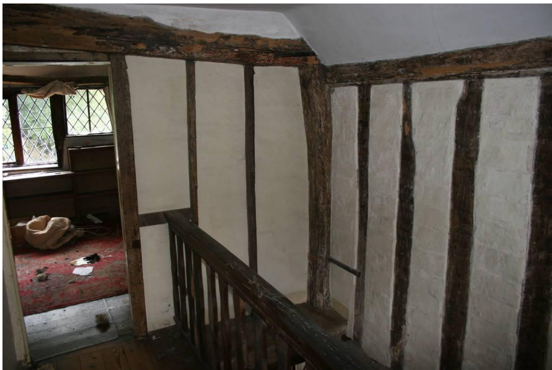
Looking across the stairwell. Note the brick noggin the wall panels.
