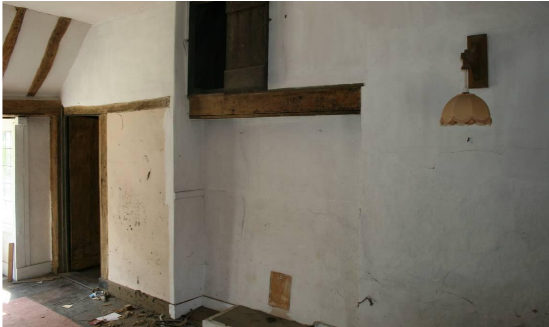
The fireplace in the main range bedroom. Looking SW.
