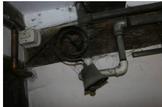
Reused C19th bell and pulley system.
