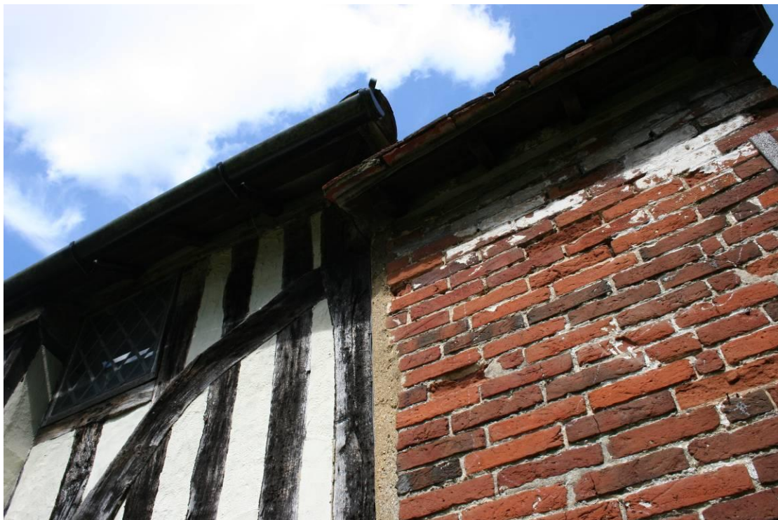
Detail of the brickwork of the brick tower.
