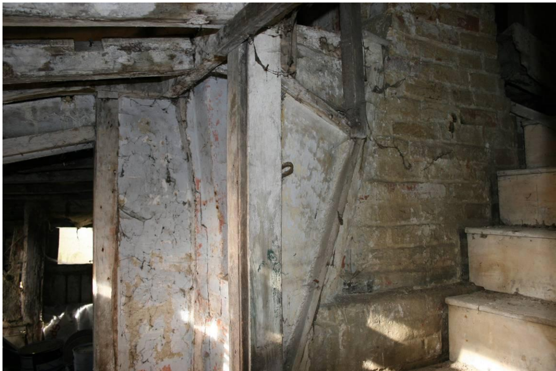
The eastern side of the firestack.
