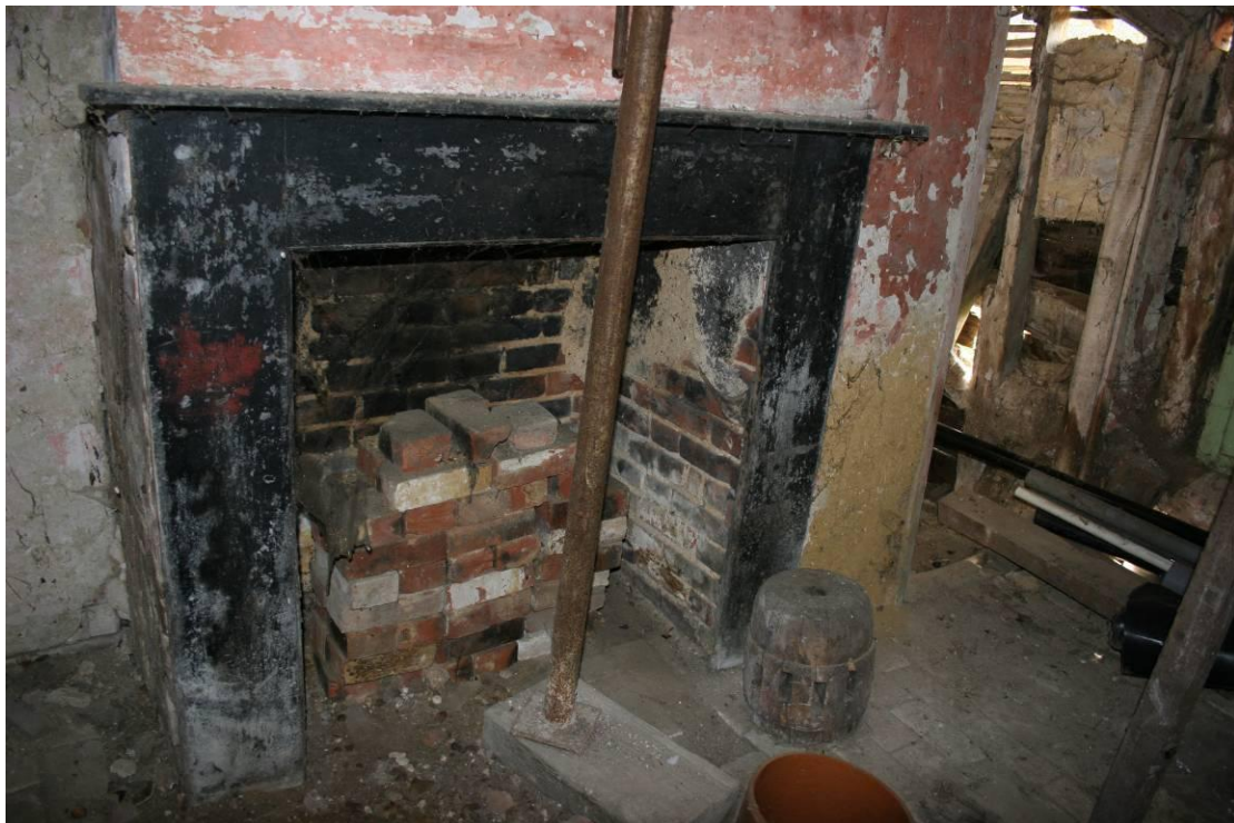
The timber fire surround in the Living Room.
