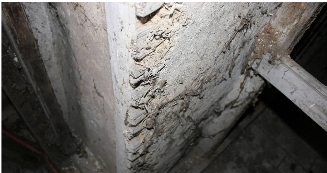
Detail of the lath and daub panel in the partition wall.
