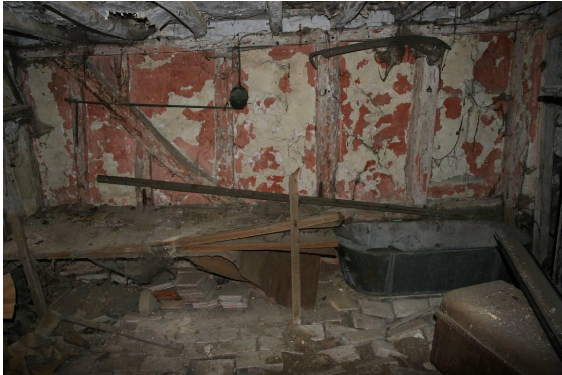
The north wall in the Living Room.
