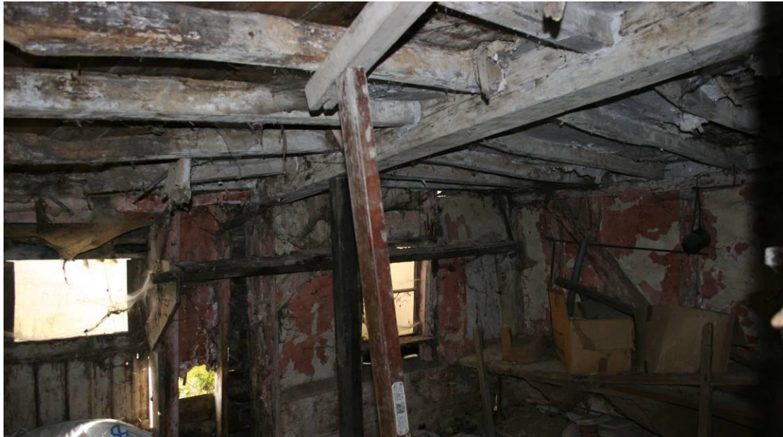
Looking W in the Living Room.
