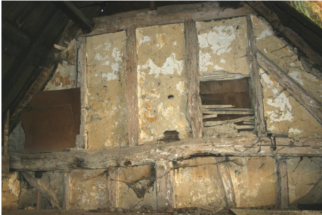
Looking E at the gable end in the upper rooms.
