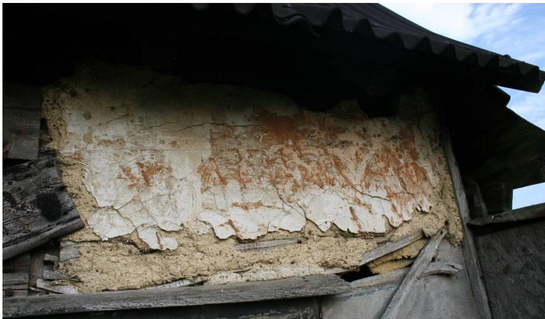
Detail of the lath and daub panel.
