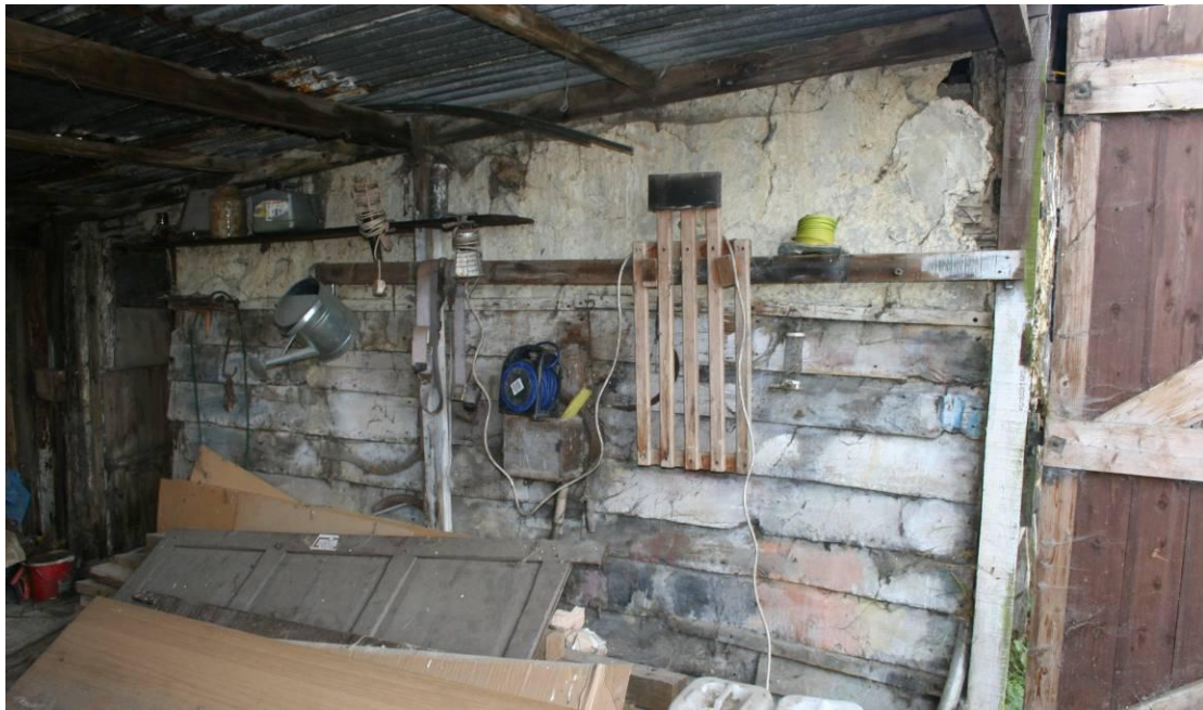
The end wall of the outbuilding in the garage.
