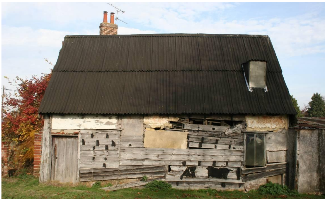
The southern elevation.
