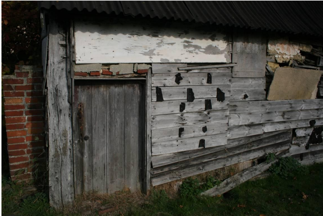
Detail of the doorway and boarded over window.
