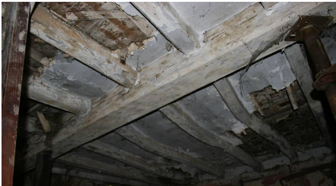
Detail of the ceiling looking NW.
