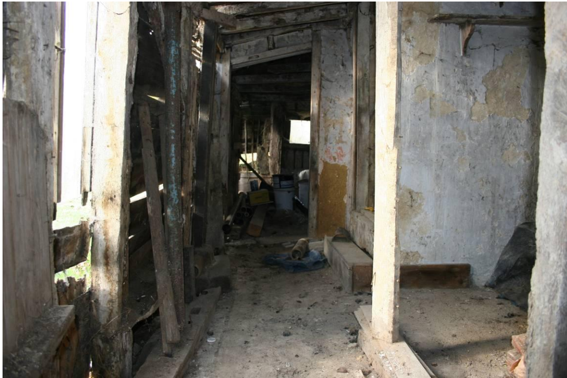
Looking W into the outbuilding. Note the many props to support the falling floor.
