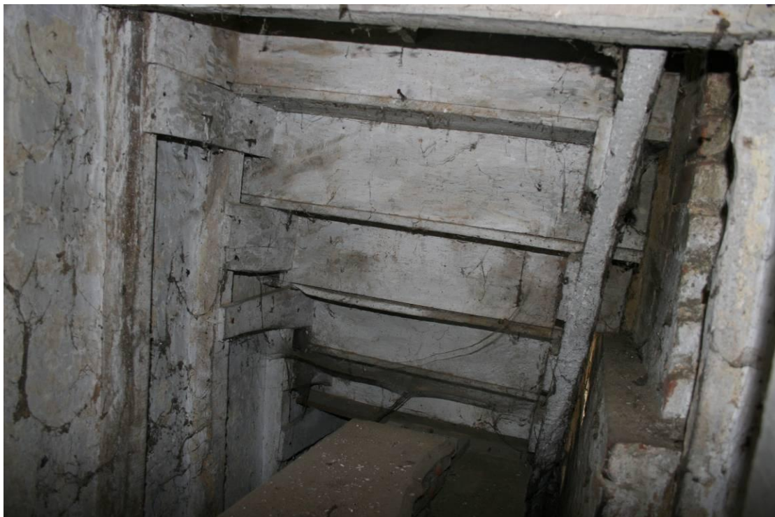
The underside of the staircase.
