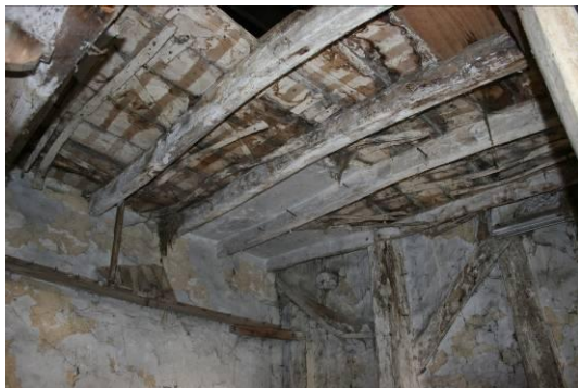
The lath and plastered ceiling.
