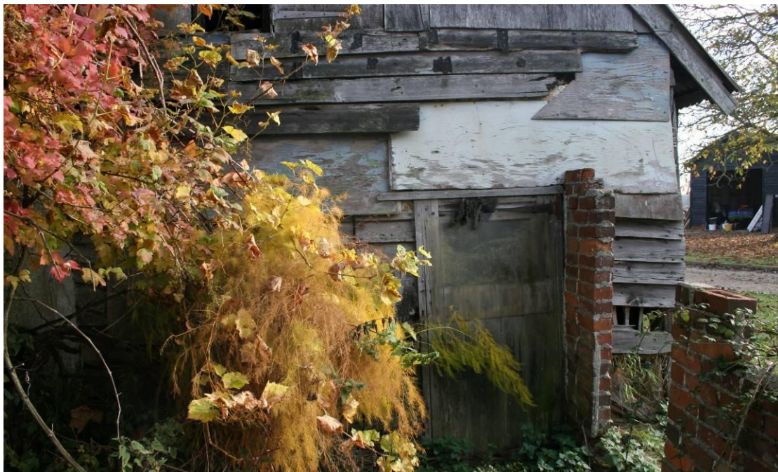
The ground floor section of the western elevation.
