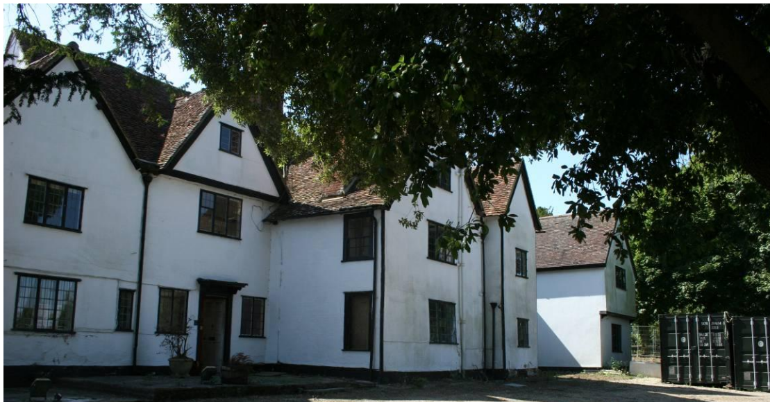
Looking SW along the northern elevation towards the Lord Butler wing.
