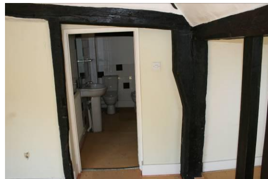
The cross-wing storey post and tie-beam.
