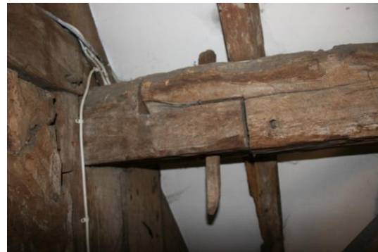
The scarf joints have oversized vertical pegs used for reassembly.
