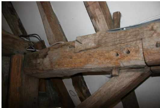
The scarf joints have oversized vertical pegs used for reassembly.
