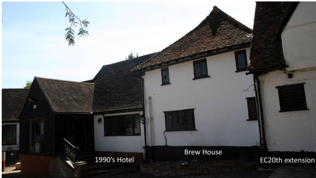
The northern elevation of the Brew House.
