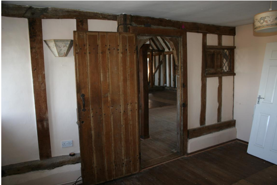
Detail of the inserted partition wall at the western end.
