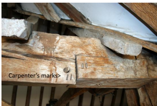
carpenter's marks on the scarf joints.
