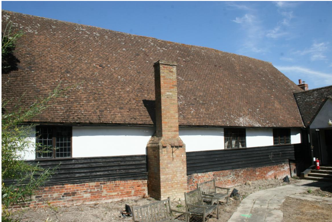
The southern elevation detailing the LC20th firestack.
