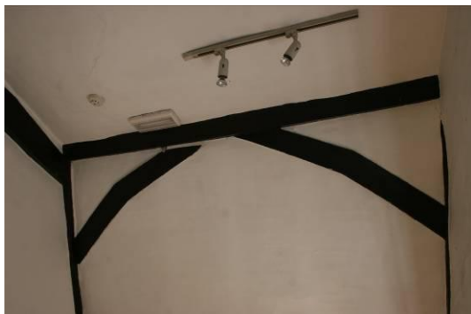
Cranked windbraces.
