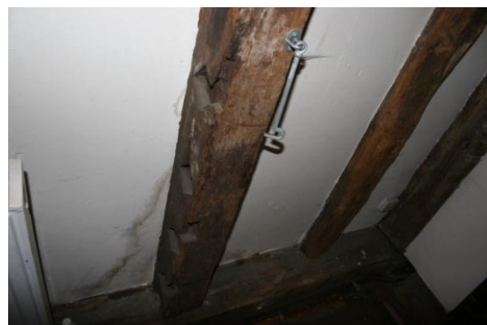
Reused window cill with diamond mullions.
