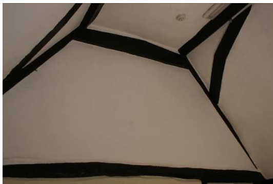
The cross-wing roof structure.
