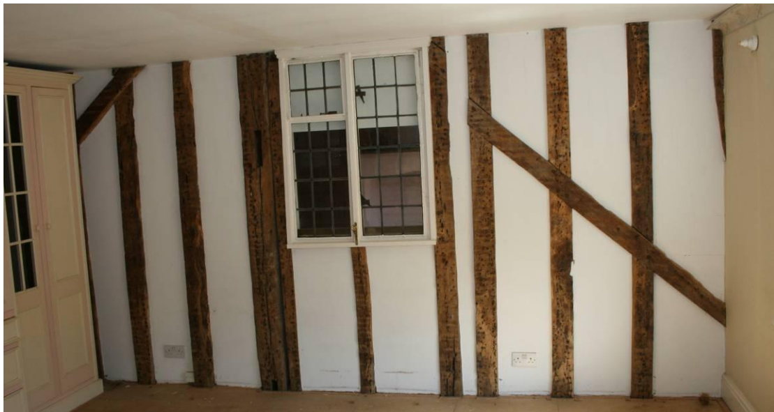
The exposed frame in the room above.
