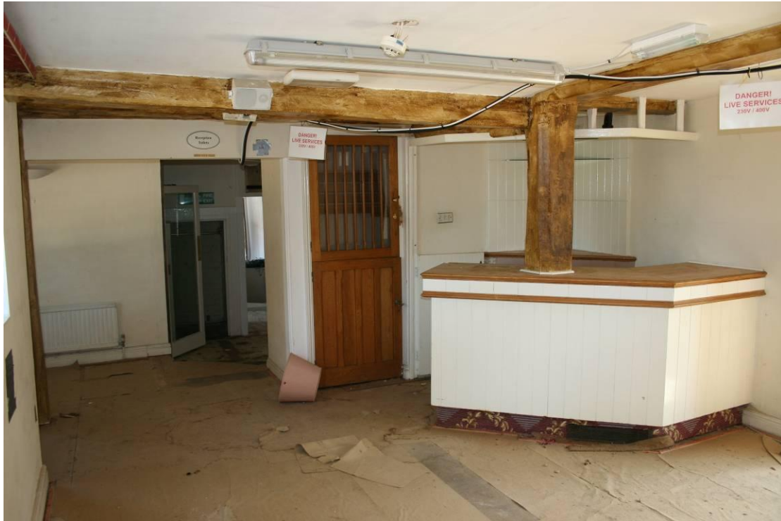
Looking E in the cross-wing. The original frame has been removed.
