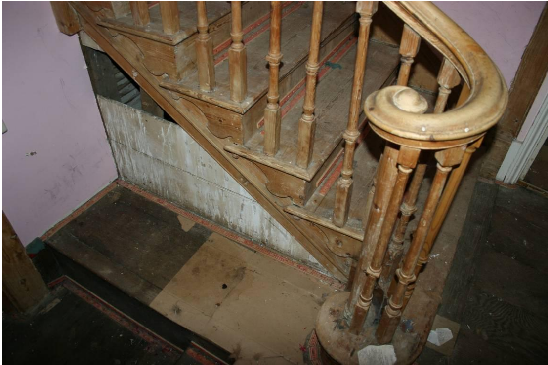
Staircase in the northern stairtower.
