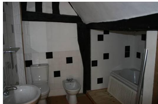
Wall removed to install bath.
