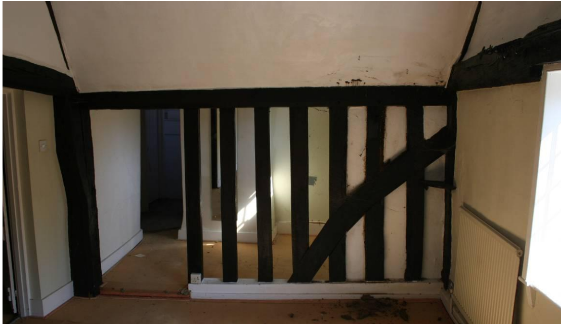
The cross-wing frame seen the upstairs bedroom
