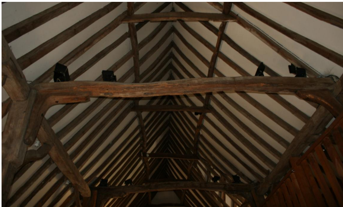
Detail of the roof structure.
