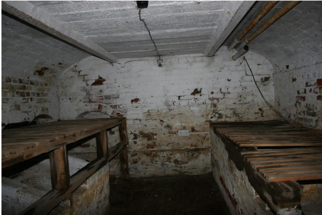
Brick vaulted cellar with wrought iron beams under the cross-wing.
