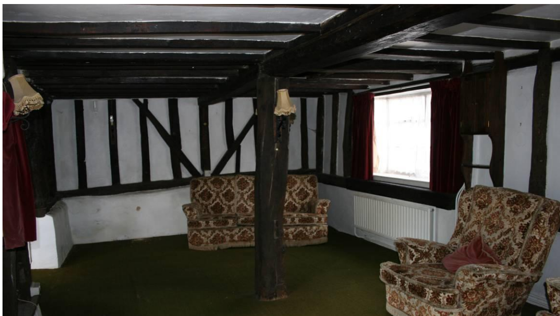
Looking W in the Sitting Room.
