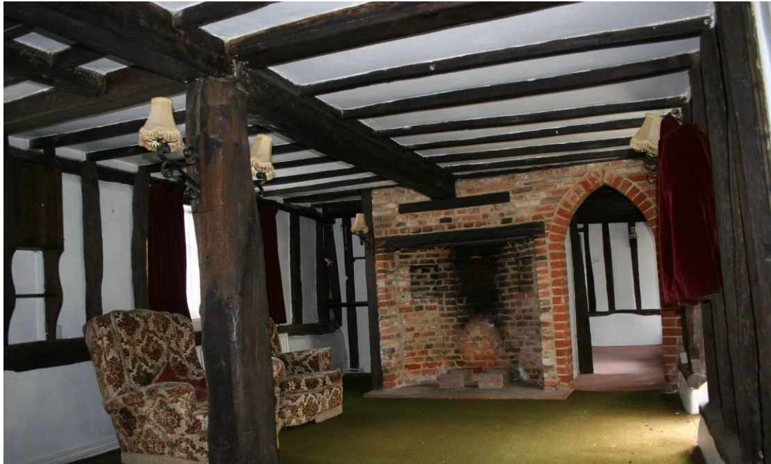
The large post replaces the original wall partition. Looking E.
