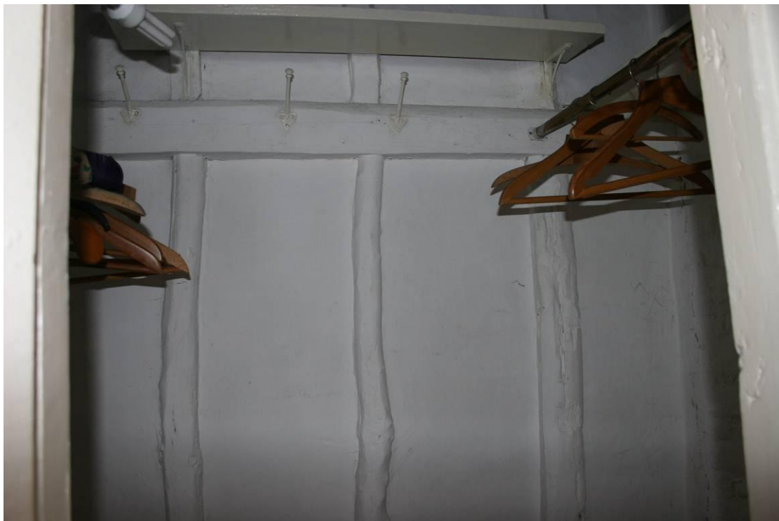
Pole construction in the closet.
