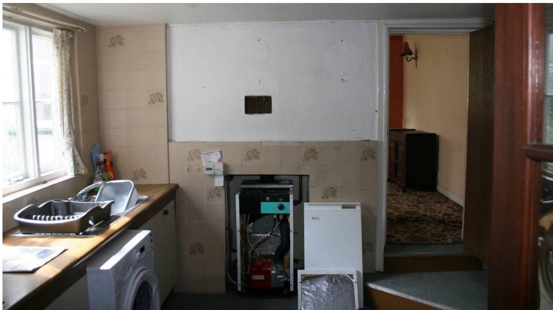
Looking N into the Kitchen.
