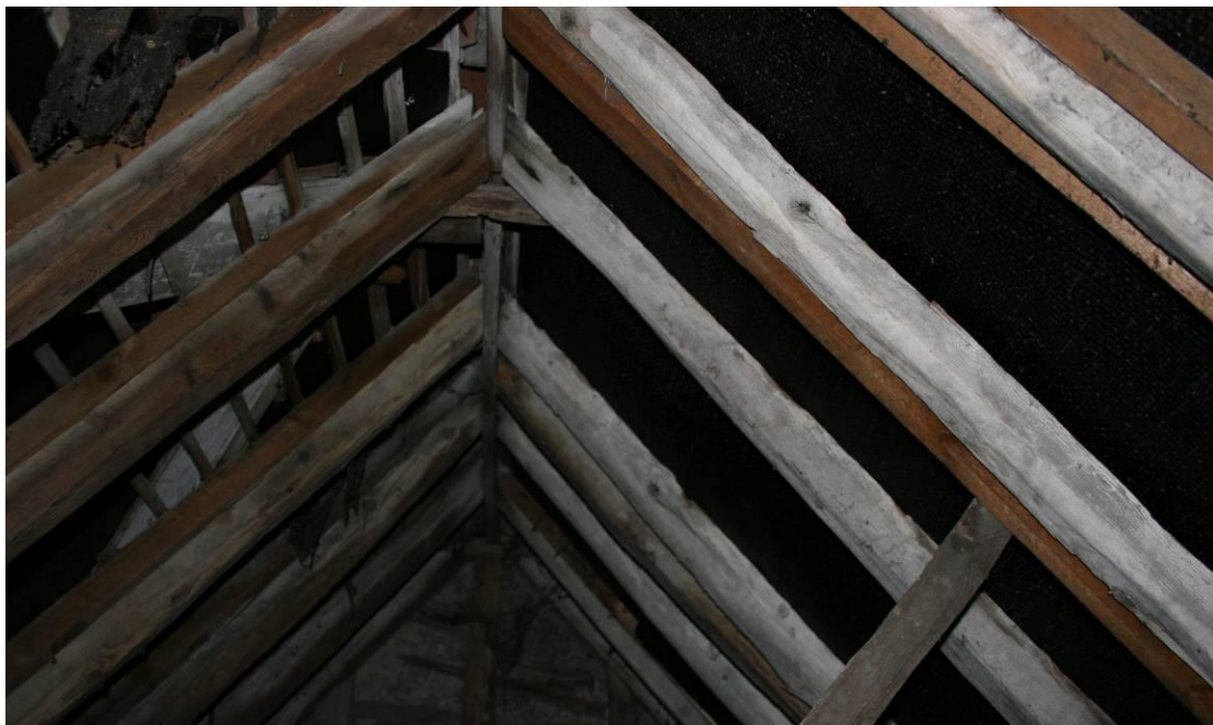
Looking W in the roof over Bedroom 2.
