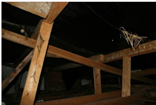
The structure of the low pitched roof and the medium density blockwork forming the wall.
