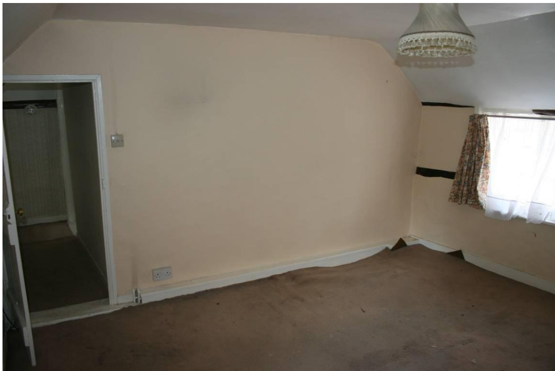
Bedroom 3 looking NW.
