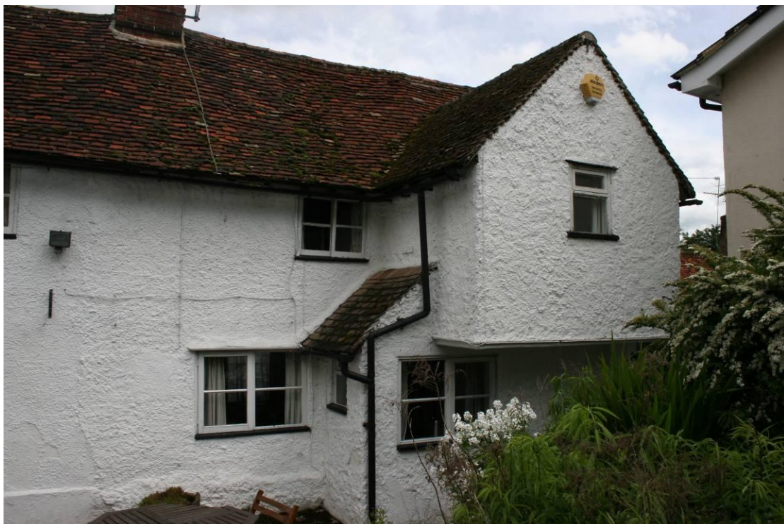
The eastern end of the southern elevation.
