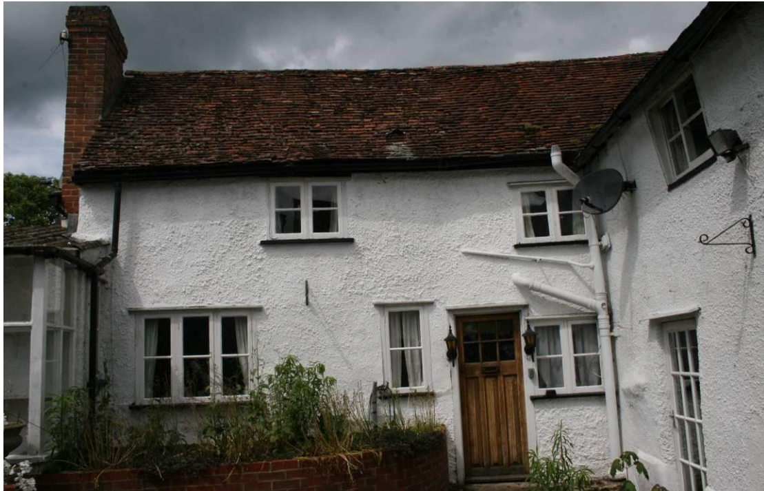
The eastern elevation of the rear range.
