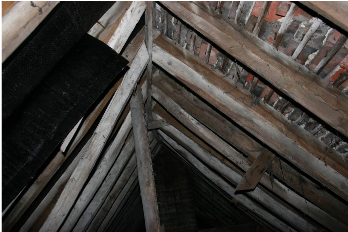
Looking E in the roof above Bedroom 3.
