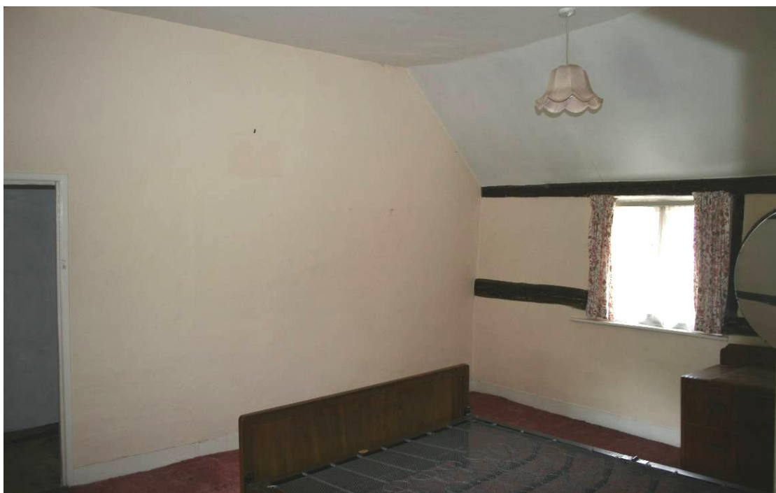
Looking NW in Bedroom 4.
