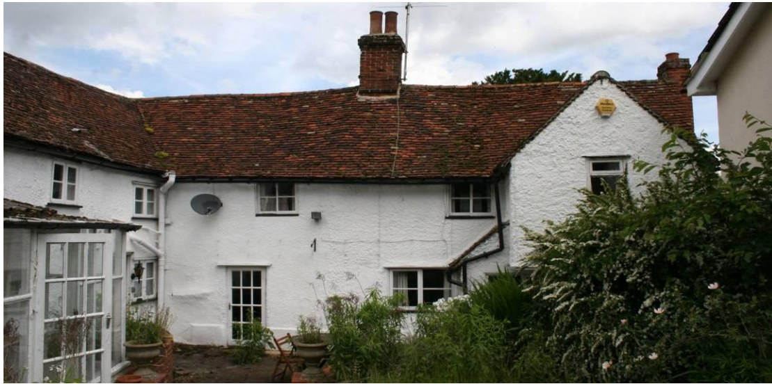
The southern elevation.
