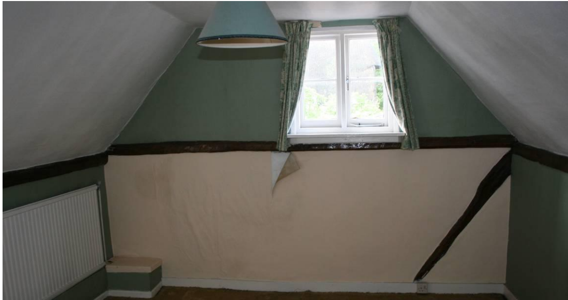
Bedroom 1 above the Kitchen displays parts of an historic frame.
