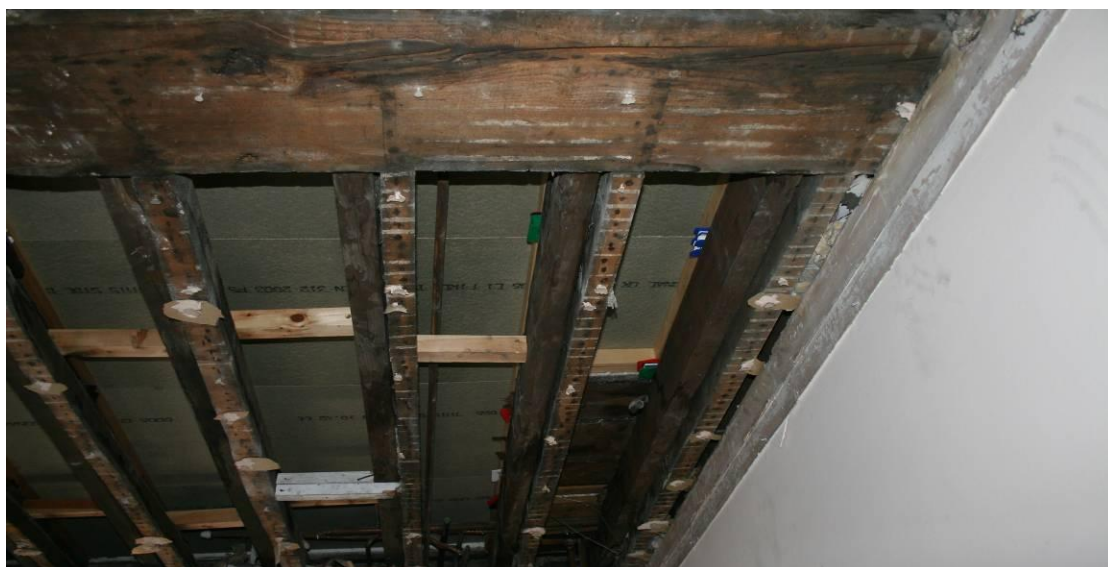
Detail of the doubled-up joists. Looking N.
