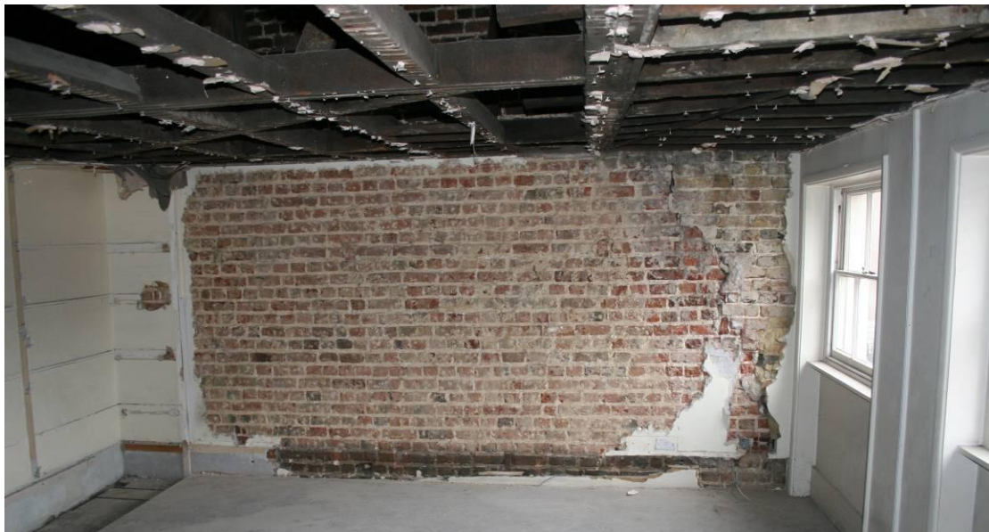
Looking W in Room TF1.
