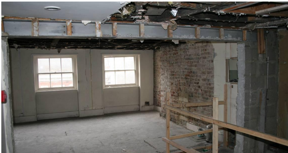
Looking N into Room TF1. Note the RSJ.
