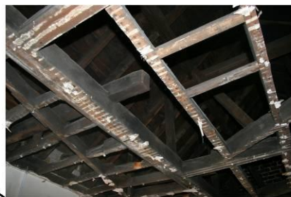
Drilling 004 - Test drilling on dry timber
