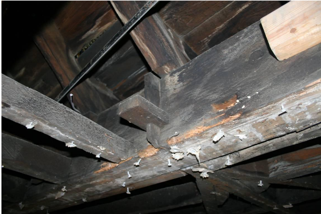
Detail of the main joist in the central valley.
