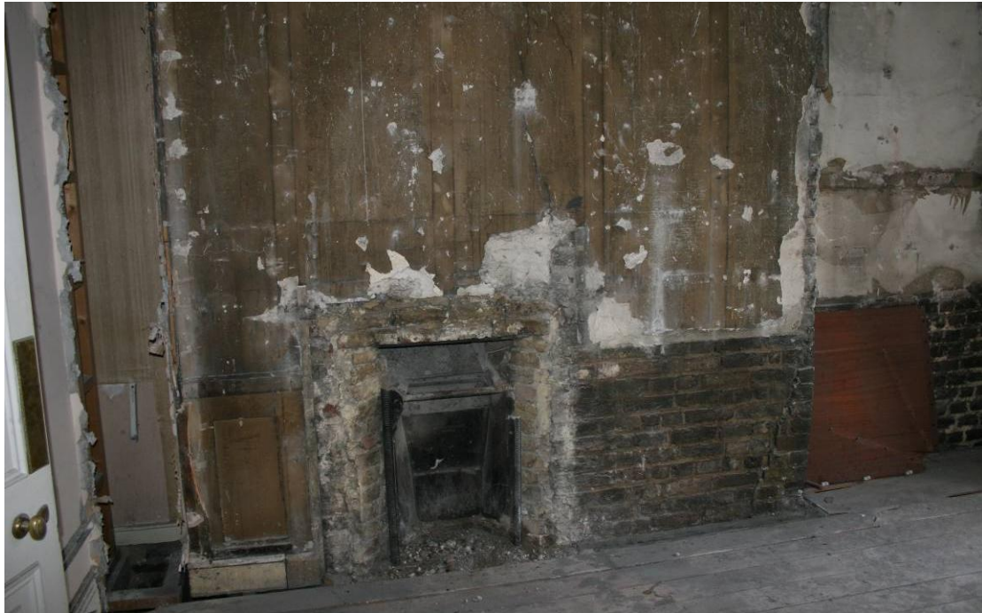
The firebreast in Room SF3. Looking E.
