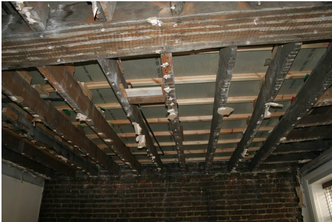
Second Floor. Room SF1 looking W. Ceiling Structure.
