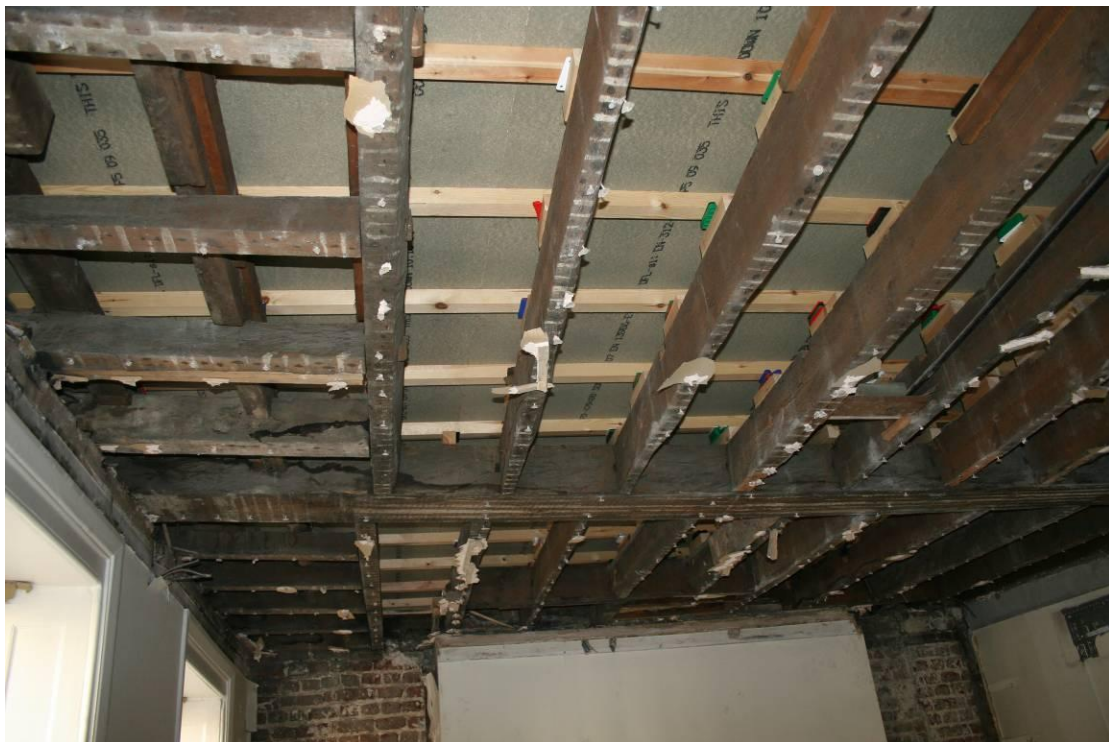
The ceiling structure near the fireplace. Looking E.
