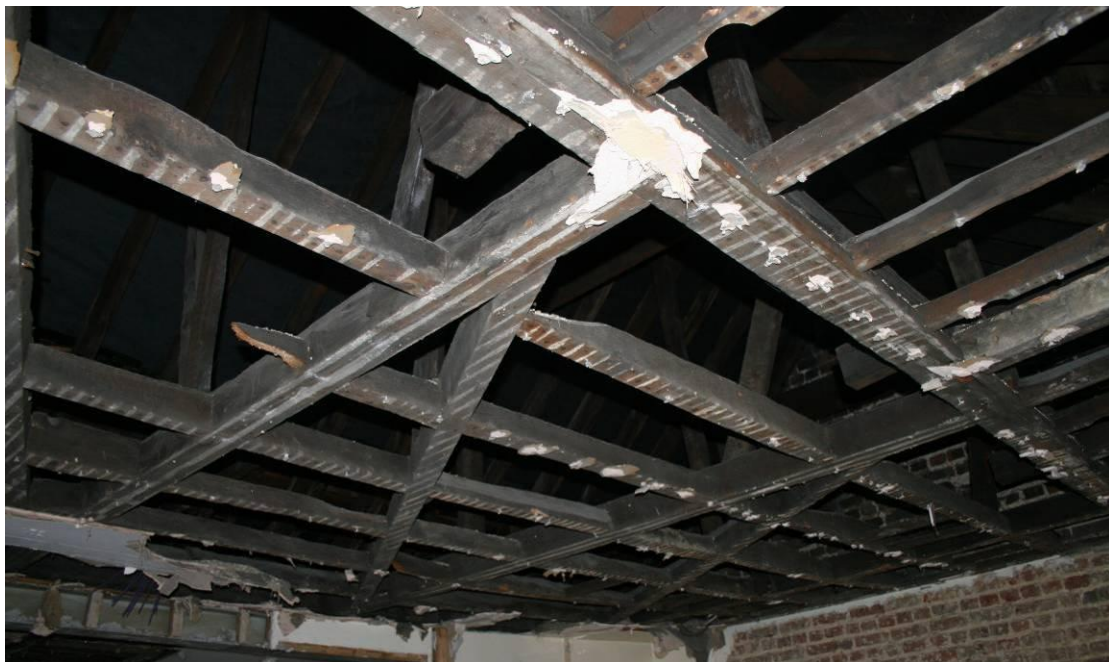
Looking SW at the ceiling
