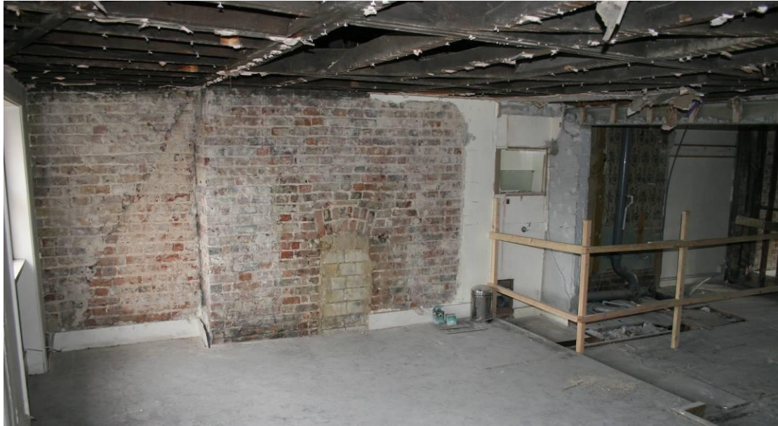
Looking SE in Room TF1. Note the line in the brickwork denoting the old roofline.
