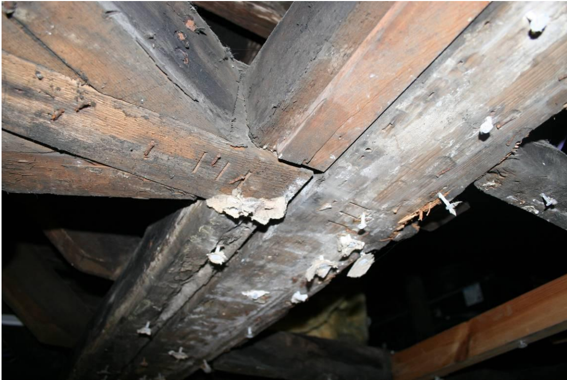
Detail of the carpentry marks at the same junction.
