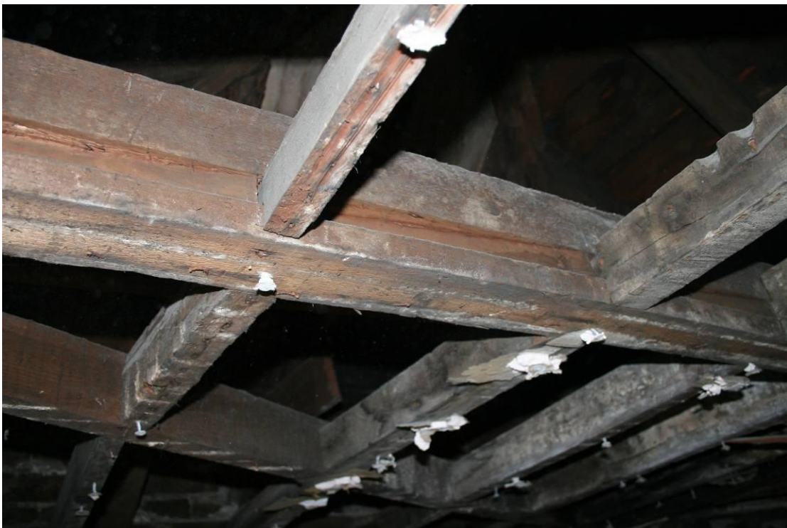
Detail of the main joist showing curved grooves to allow the common joist to be rotated in.
