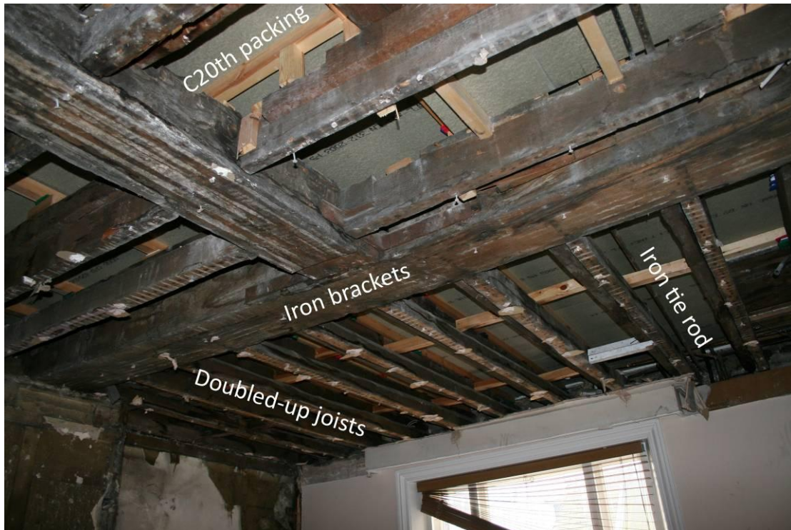
The ceiling in the back room SF3.
