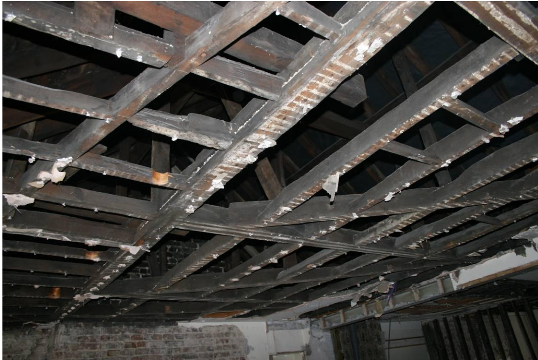
Looking SE at the ceiling near the fireplace.
