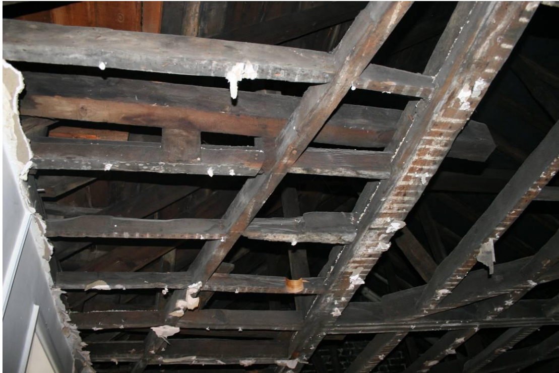
The ceiling joists at the front of the house. Looking E.
