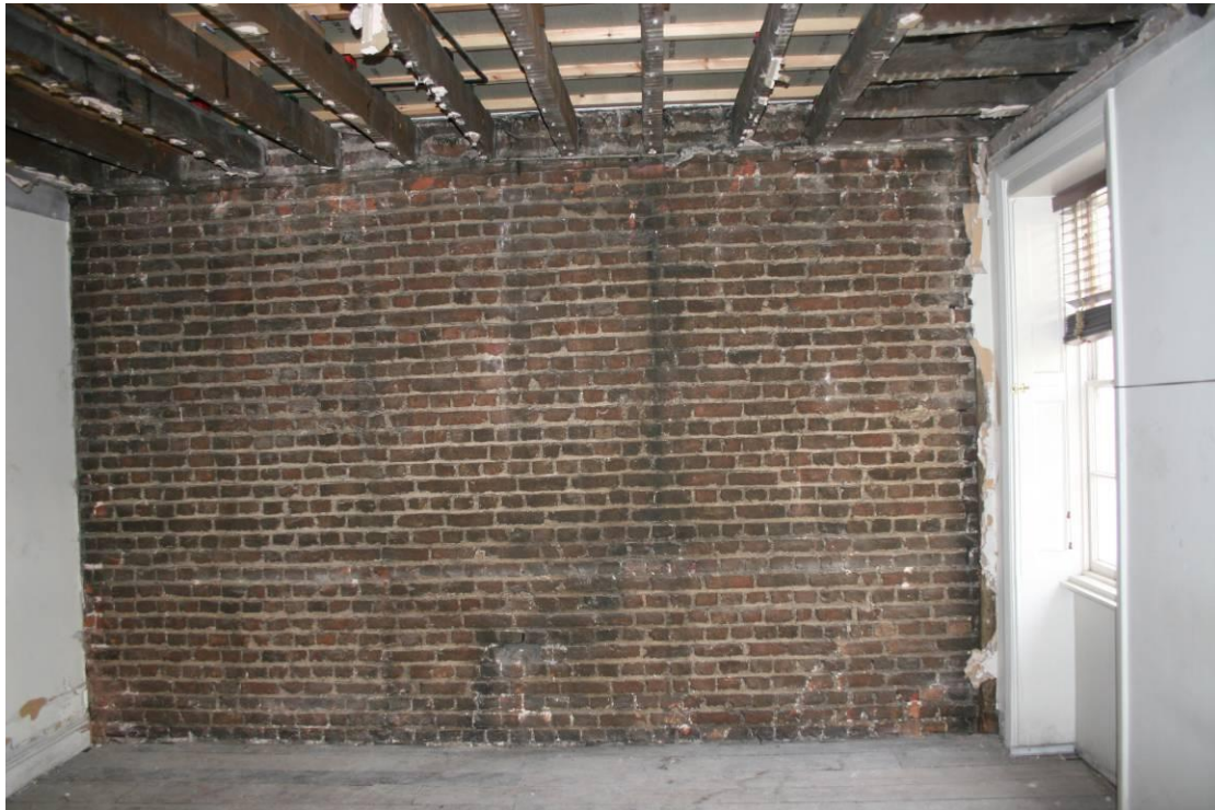
Second Floor. Room SF1 looking W.
