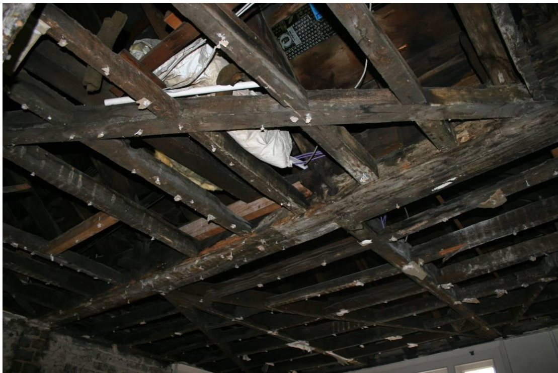
The ceiling in Room TF3 looking SE.
