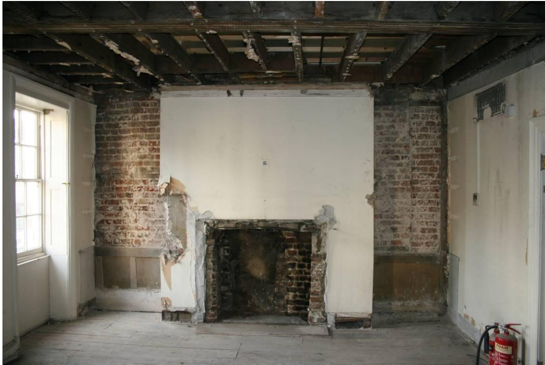
Second Floor. Room SF1 looking E. Exposed fireplace and panelling.
