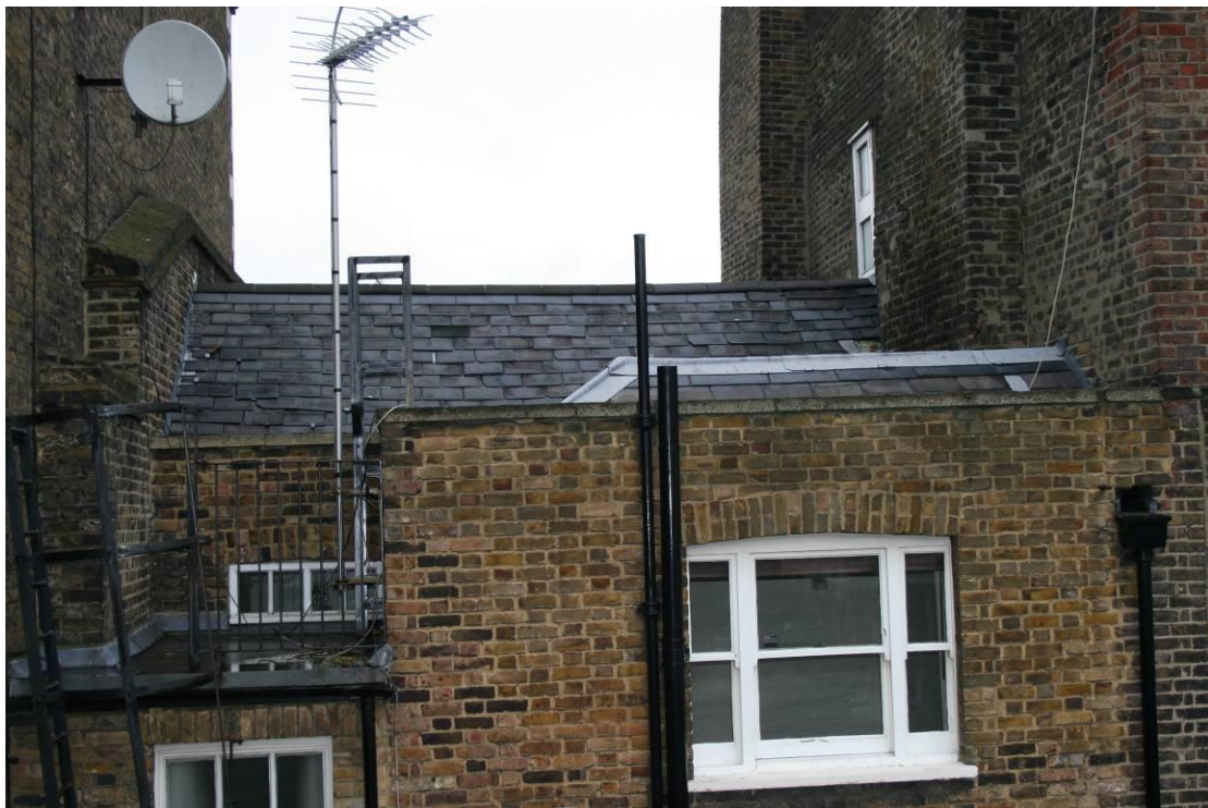
Detail of the rear of the roof. Looking N.
