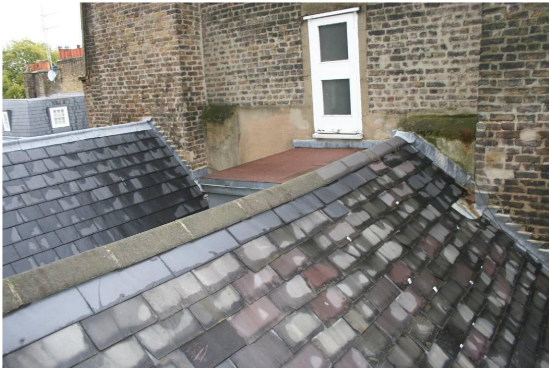
Detail of the roof looking NE. Note the flat roofed cubicle.
