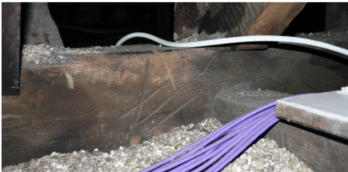
Detail of the main axial joist.
