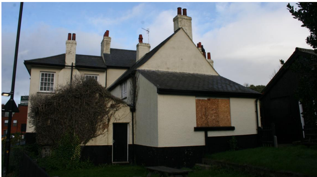
The southern elevation.
