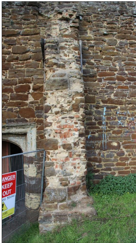
Plate 8: Buttress detail showing brick pieces in the infill
