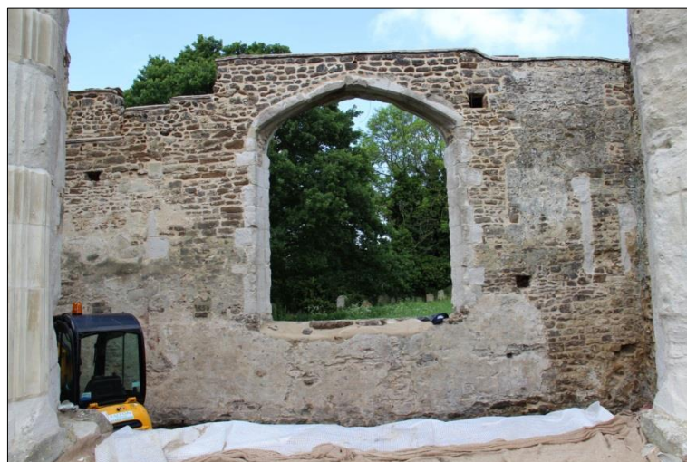
Plate 36: North nave wall
