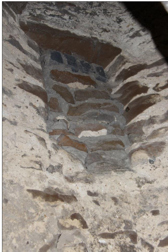
Plate 21: Blocked stair turret window
