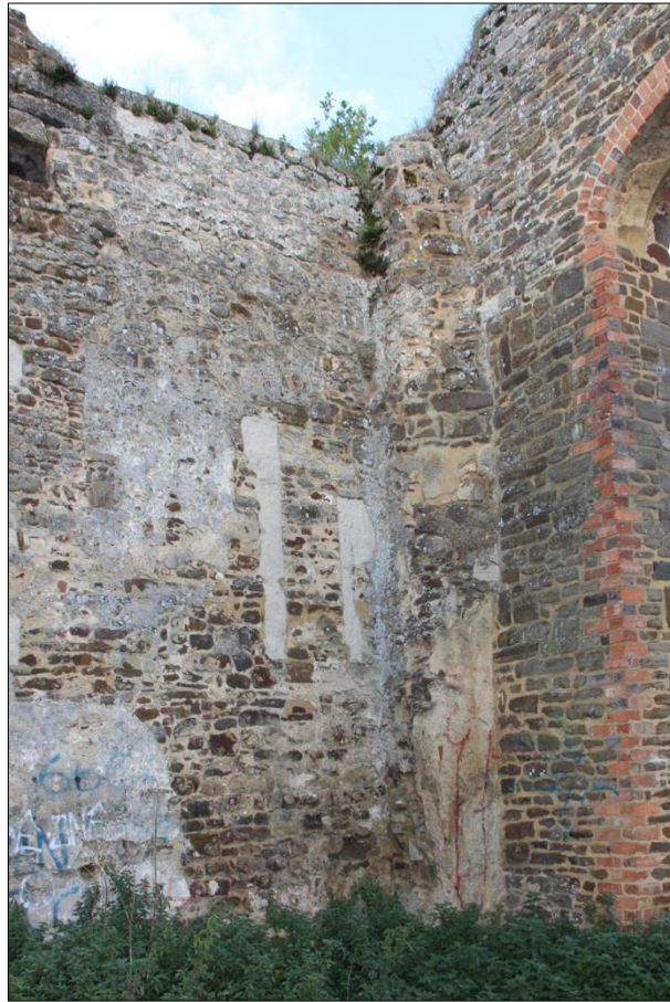
Plate 10: Eastern end of the north wall
