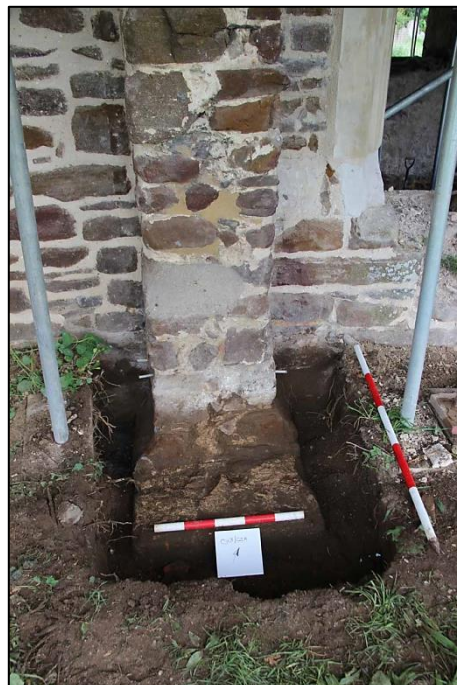
Plate 30: Test pit C: butress footings (104), looking N (0.5m and 1m scale)
