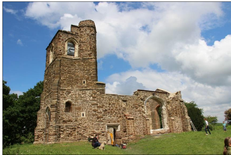
Plate 35: General view from the southwest
