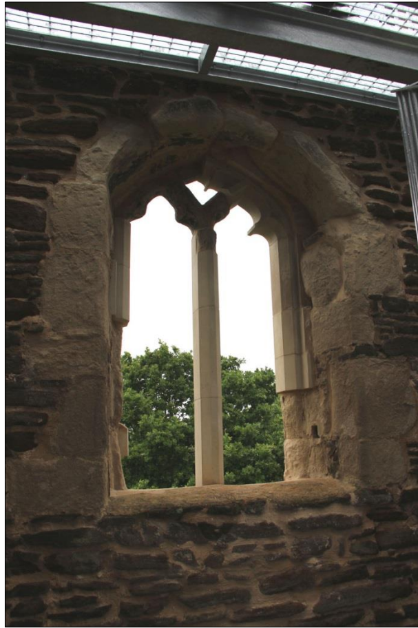
Plate 25: North window tracery restored
