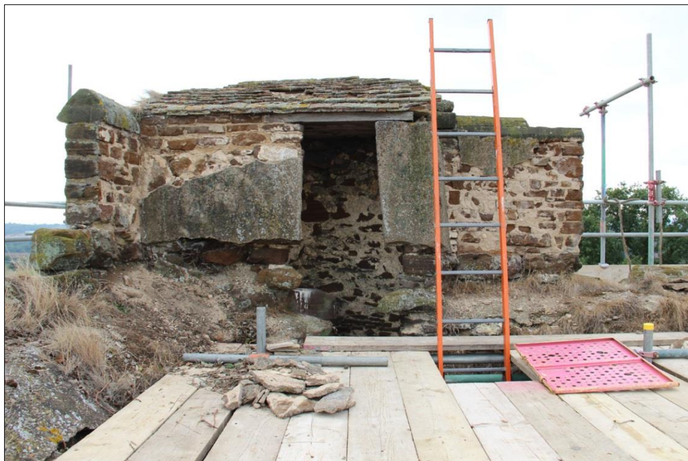
Plate 18: The top of the stair turret
