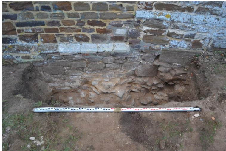
Plate 6: Eastern test pit showing earlier masonry below the foundation (Kenny 2011)
