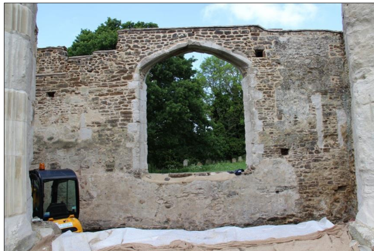
Plate 39: North nave wall
