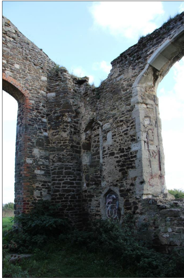
Plate 17: Rood loft doors in the south wall
