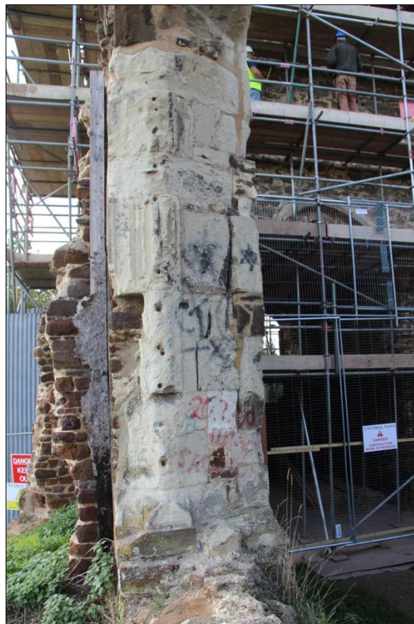
Plate 16: Detail of the western side of the southern Perpendicular window
