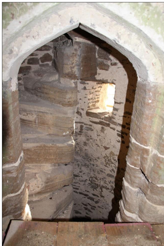
Plate 22: Upper stair turret window and stairs
