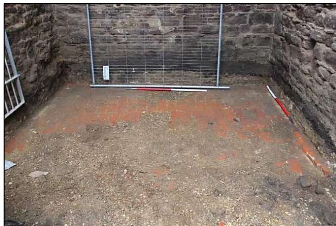
Plate 31: Brick floor [105] in tower, looking W (2x1m scale)
