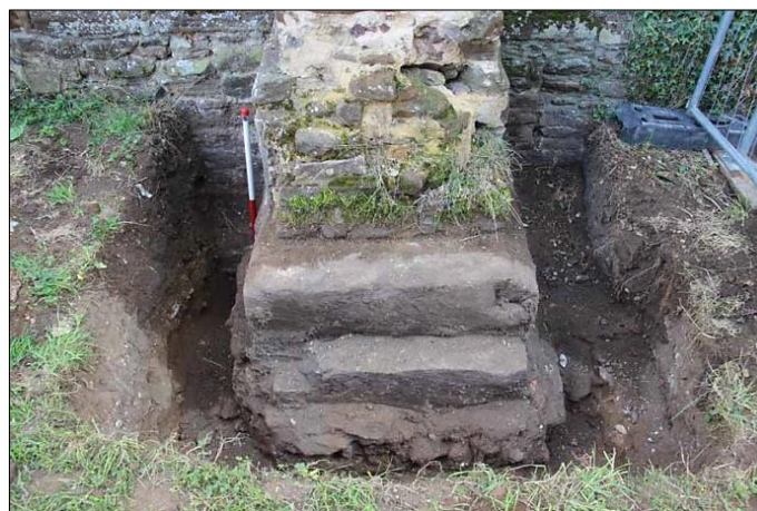
Plate 28: Test pit B: butters footings (104), looking S (1m scale)
