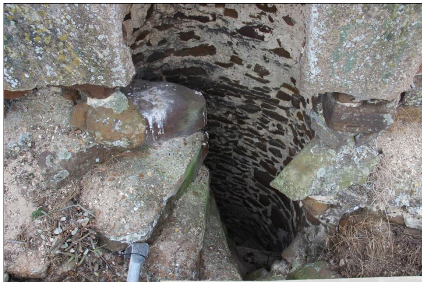
Plate 20: View into the stairwell from above
