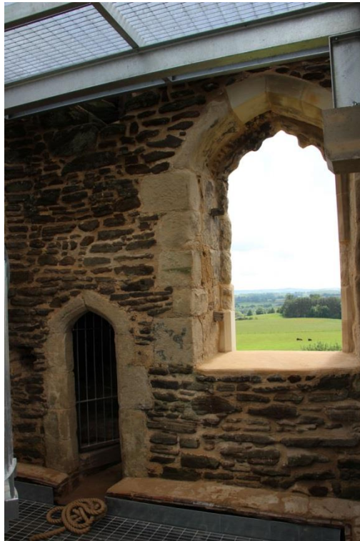
Plate 40: Bell chamber, south wall
