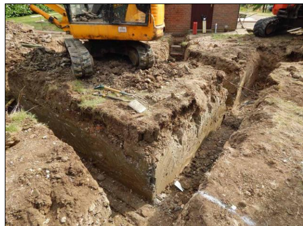
Plate 6: Trenches between main building garage, facing SE
