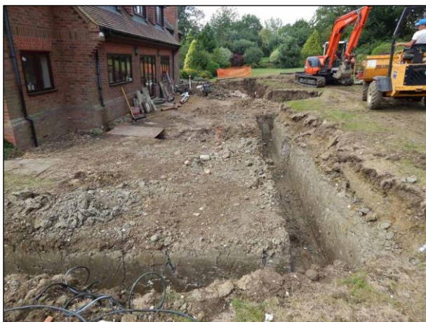
Plate 5: Footing trenches at rear of house, facing NW
