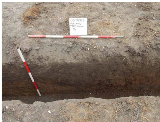
Plate 3: Tree throw towards northwest corner of footing trench for Plot 2 (scale 2x1m)
