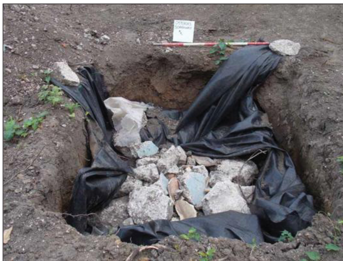
Plate 4: Backfilled soakaway trench (scale 1m)
