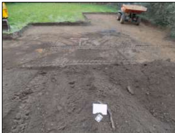
Plate 1: SW section of house ground reduction
