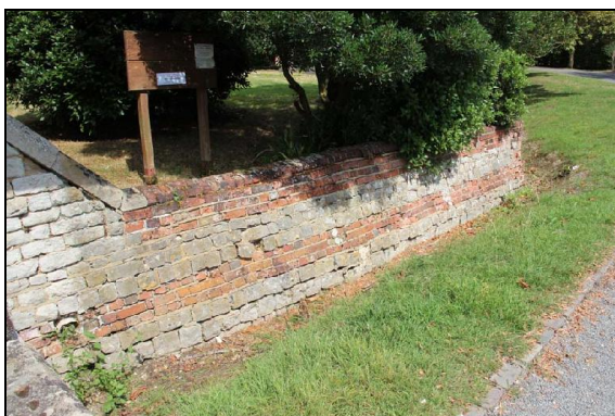
Plate 5: Retaining wall with existing drain pipe on left, view northeast
