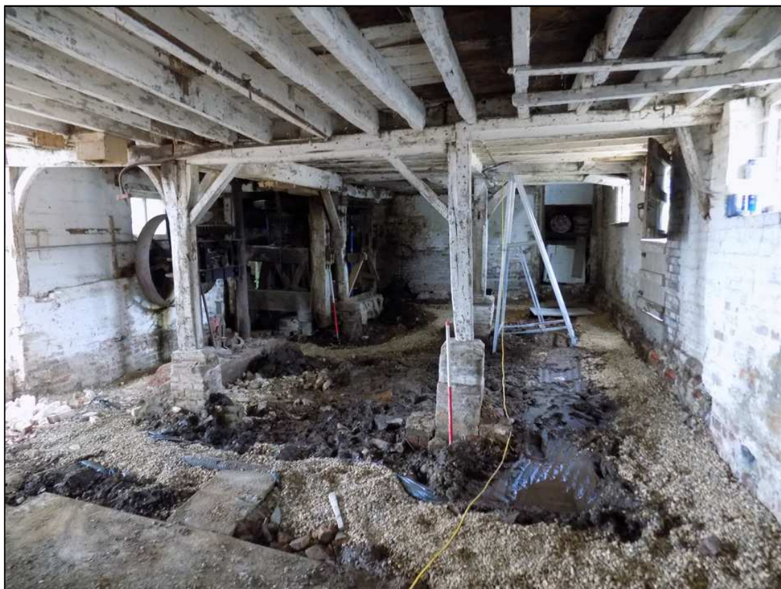
Plate 3: After ground reduction, facing south
