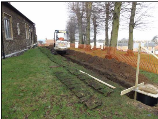
Plate 9: Drainage trench, looking NW
