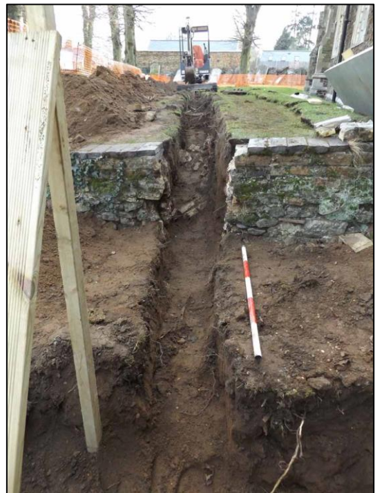
Plate 8: Drainage trench, looking E (1m scale)
