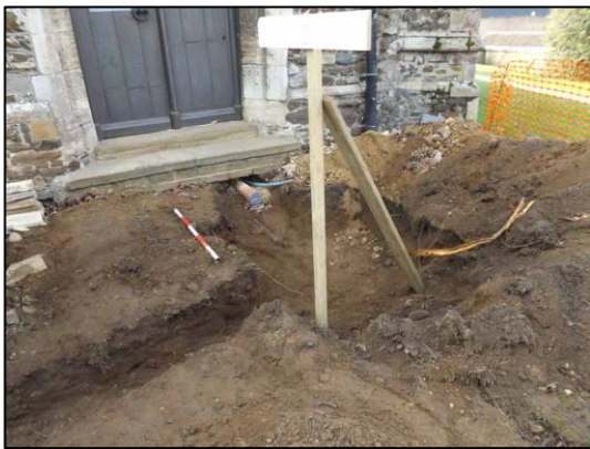
Plate 7: Drainage trench, looking SW (1m scale)
