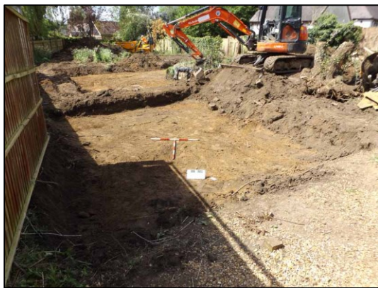
Plate 3: New garage area, looking SW (2x1m scale)
