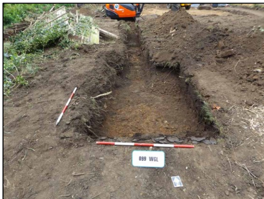
Plate 5: Soakaway and drainage trench, looking NNE (2x1m scale)
