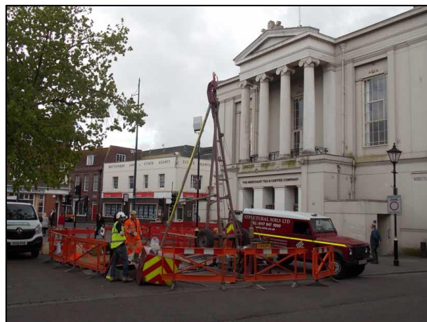
Plate 15: Borehole drilling to the NE of the Town Hall, looking S
