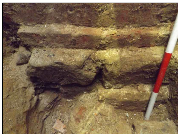
Plate 8: Test Pit 4, clunch foundations [403], looking SE (1m scale)
