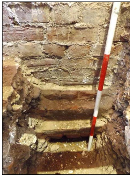
Plate 4: Test Pit 3, Town Hall brick foundations [301], looking NE (2m scale)
