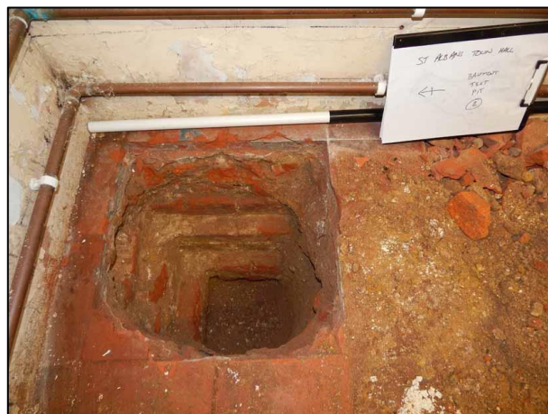
Plate 2: Test Pit 2, looking NE
