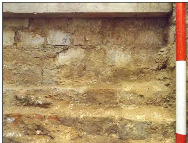
Plate 7: Test Pit 4, brick foundations [401], looking SE (1m scale)
