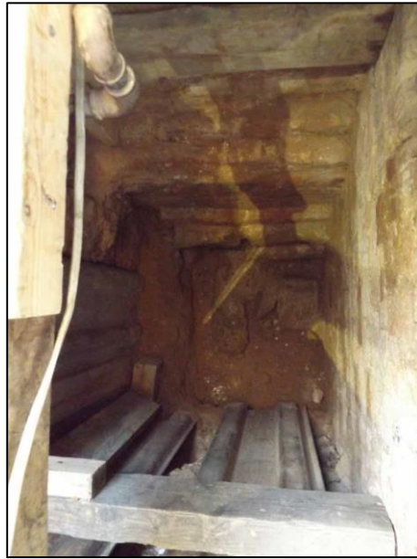
Plate 6: Test Pit 4, Town Hall foundations, looking SE
