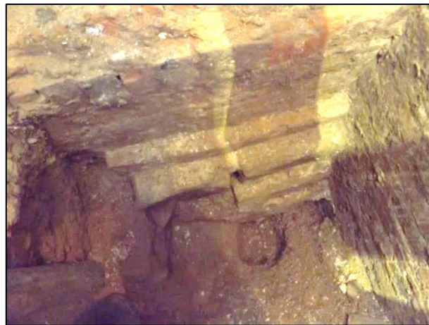
Plate 10: Test Pit 4, foundations [401 & 403] and cellar construction cut [406], looking SE
