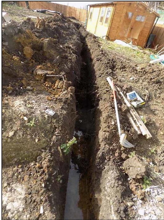
Plate 20: Services, trench 4, looking south-west (1m scale)
