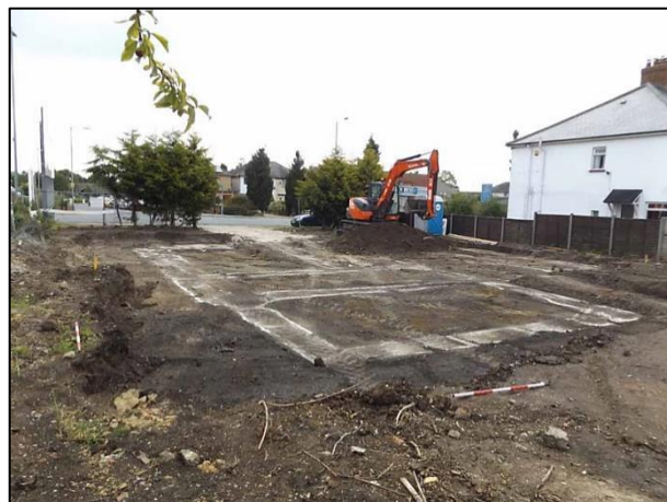
Plate 3: Ground reduction, looking east (2x1m scale)
