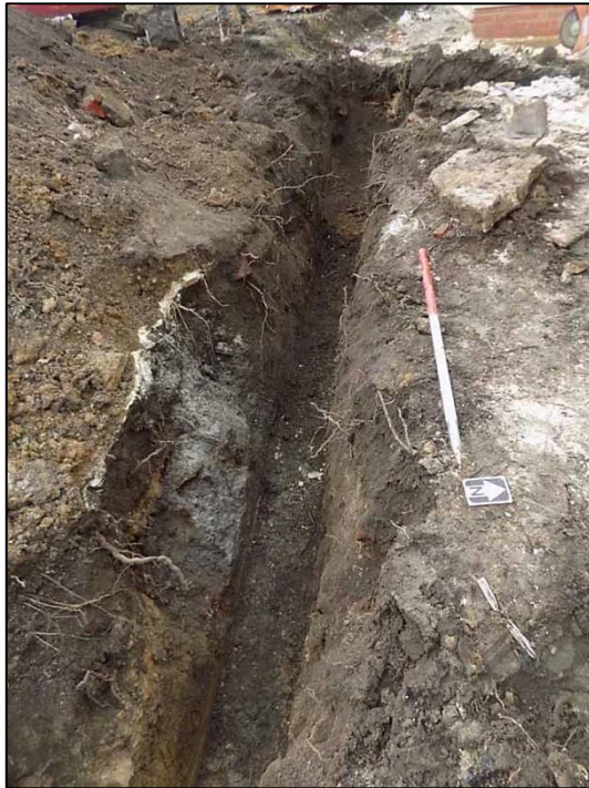
Plate 15: Services, trench 2, looking west (1m scale)
