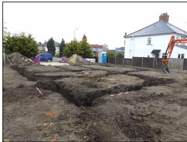
Plate 1: Footing trench, looking east (2x1m scale)
