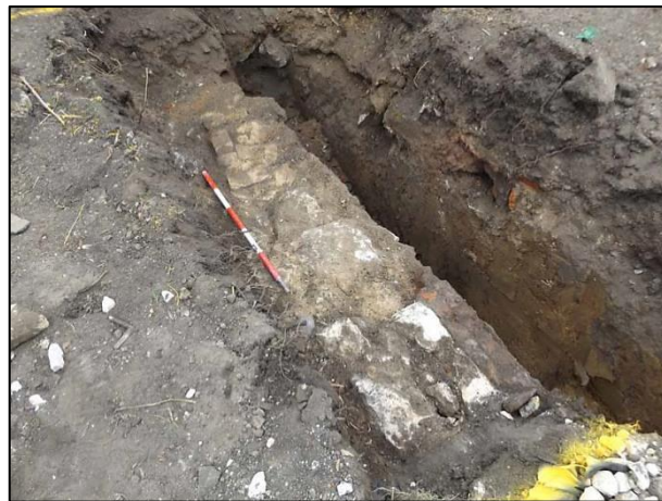
Plate 5: Footing trench, stone wall [108] & brick wall [110], looking south (1m scale)
