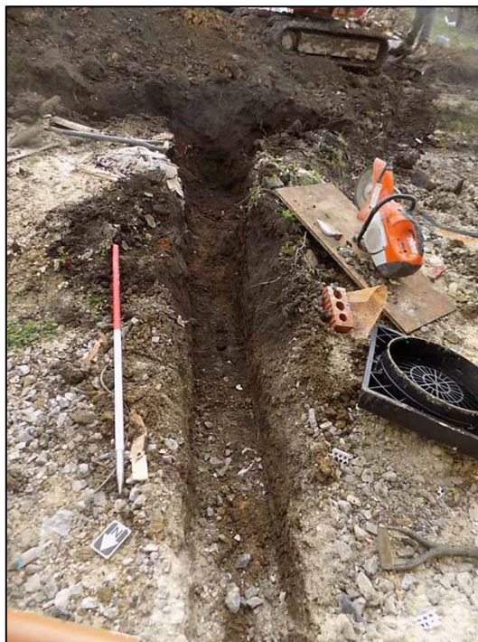
Plate 18: Services, trench 3, looking south-west (1m scale)
