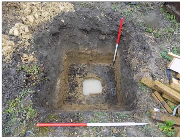
Plate 13: Services, soakaway, looking north-east (2x1m scale)
