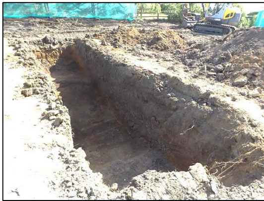
Plate 6: Trench 1: large ditch [104], looking SW (scale 2x1m)
