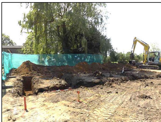
Plate 9: Footing trenches: general shot, looking S (scale 2x1m)
