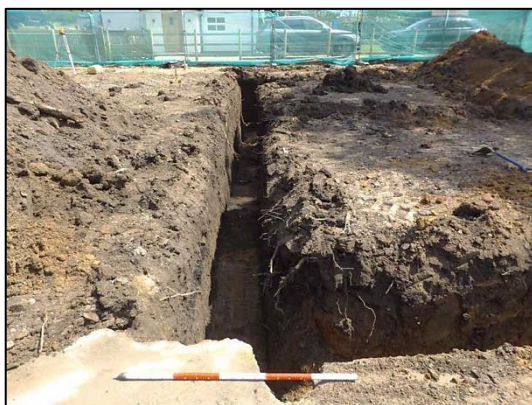
Plate 11: Footing trenches: large ditch [104], looking E (scale 1m)
