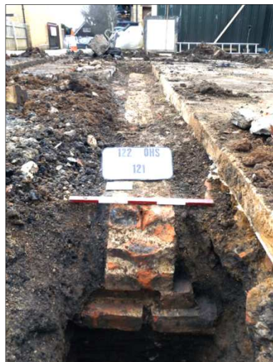
Plate 21: Plot 2, Brick wall (121), centre trench facing E
