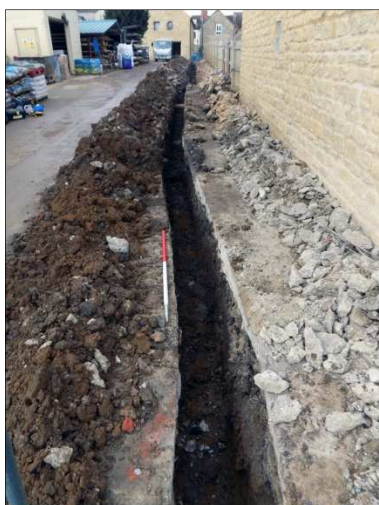
Plate 25: Service trench, facing W
