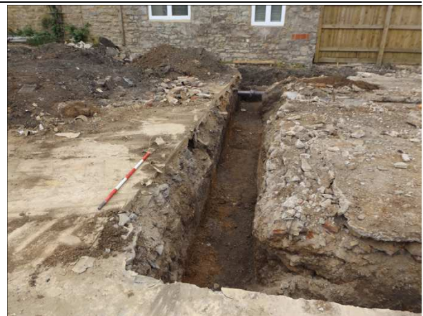
Plate 4: Plot 4, west trench facing N
