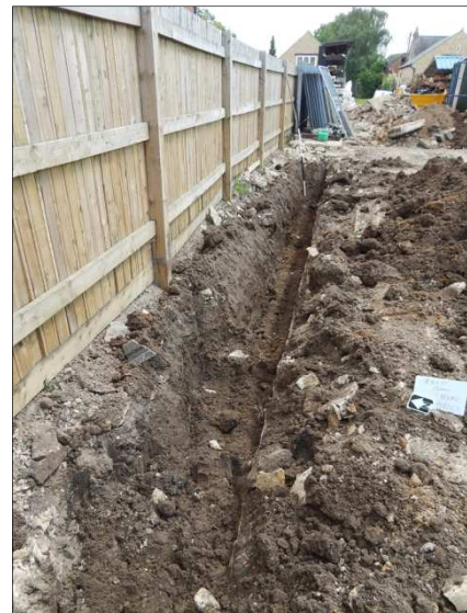
Plate 2: Drainage ditch along north boundary of site, facing E
