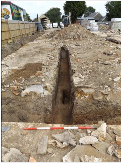
Plate 7: Plot 4, middle trench facing E
