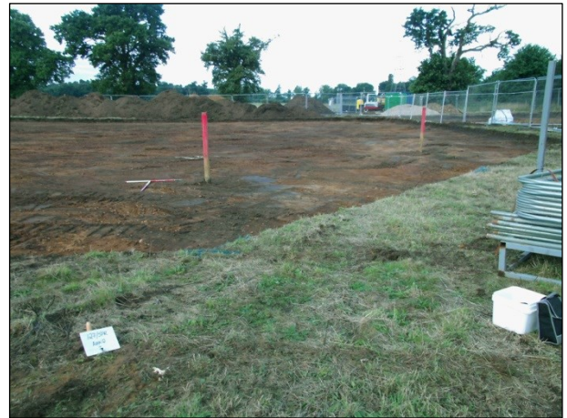
Plate 9: Area 2 ground reduction facing southwest
