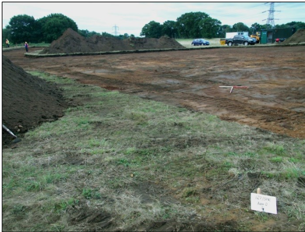
Plate 8: Area 2 ground reduction facing south
