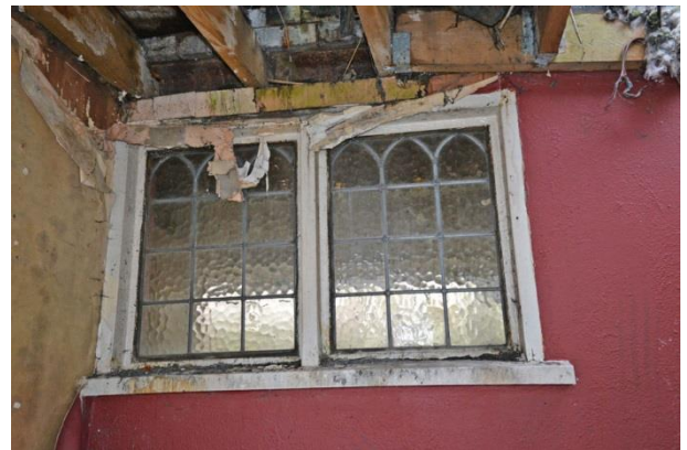
Plate 28: Modern leaded window in west wall of G2
