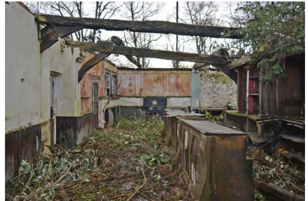
Plate 20: View northwards from Room G3
