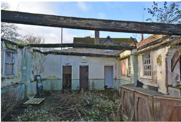
Plate 9: Interior of Main Range (G4) looking west
