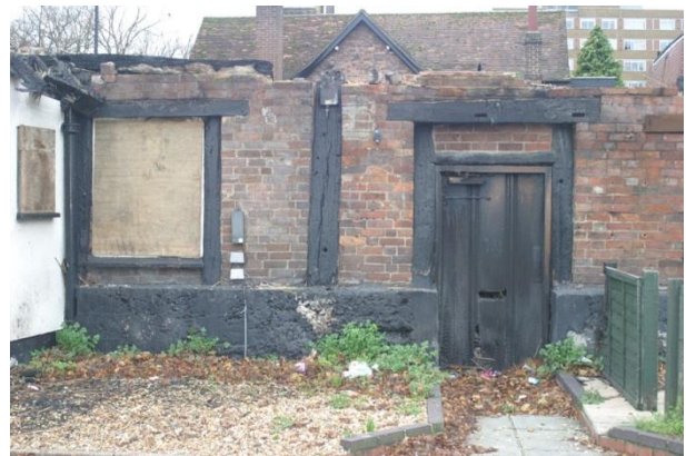
Plate 14: East wall, Bay 1
