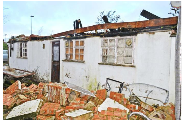
Plate 4: West elevation of East Range from the SW
