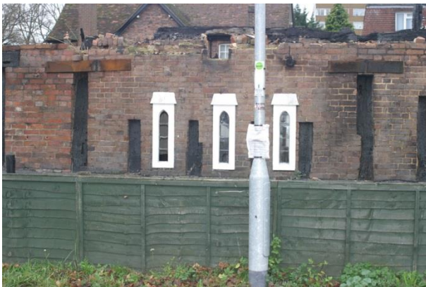
Plate 15: East wall, Bay 2
