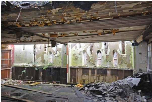
Plate 25: East wall of Room G2
