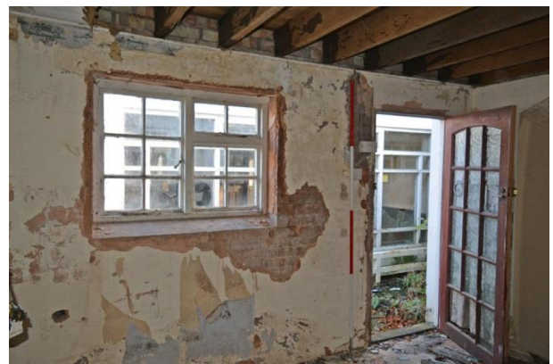
Plate 36 East wall of Room G6
