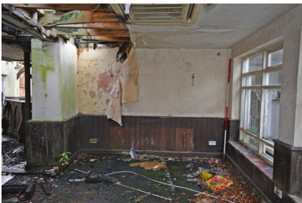
Plate 29: Room G1, looking south
