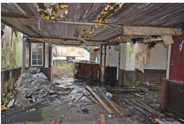
Plate 23: Room G2 looking south
