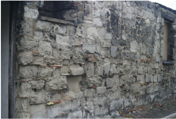
Plate 7: Brick & tile within clunch wall
