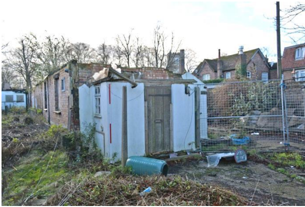
Plate 1: North & east elevations of East Range
