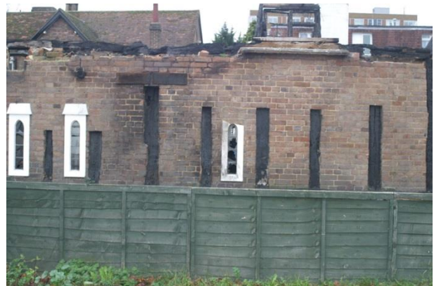
Plate 16: East wall, Bay 3
