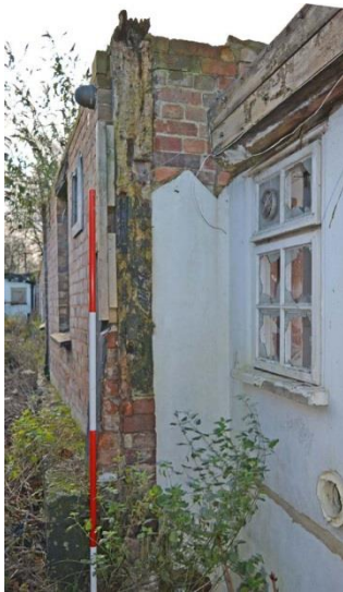
Plate 19: Northeast corner post of East Range
