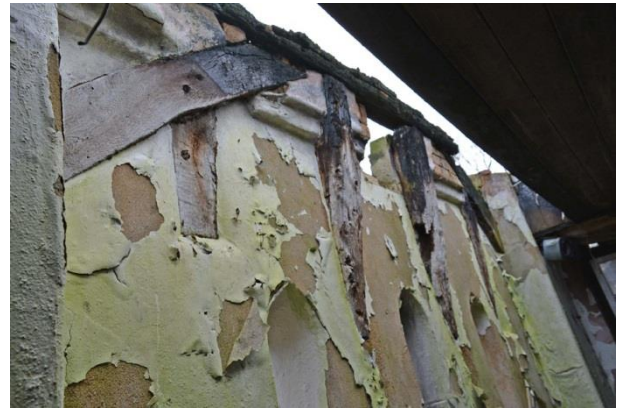
Plate 26: Internal bracing in east wall of Room G2
