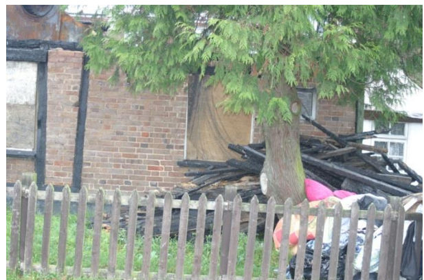
Plate 18: East wall, Bay 5
