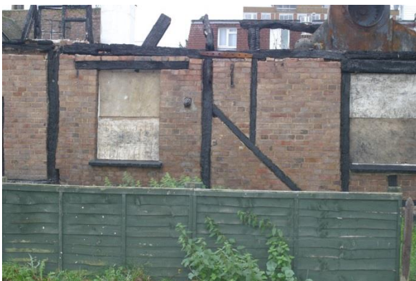
Plate 17: East wall, Bay 4
