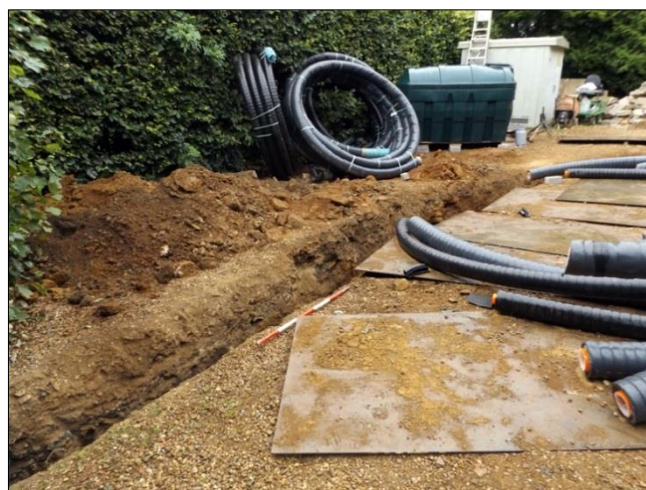
Plate 5: Southwestern end of trench, facing south, with 1m scales
