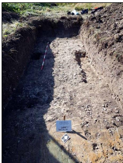
Plate 7: Stone surface (109), wall base [107] and possible wall foundation [105]. 2m scale.
