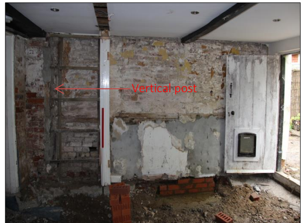
Plate 16: Partition wall between Rooms G6 & G8
