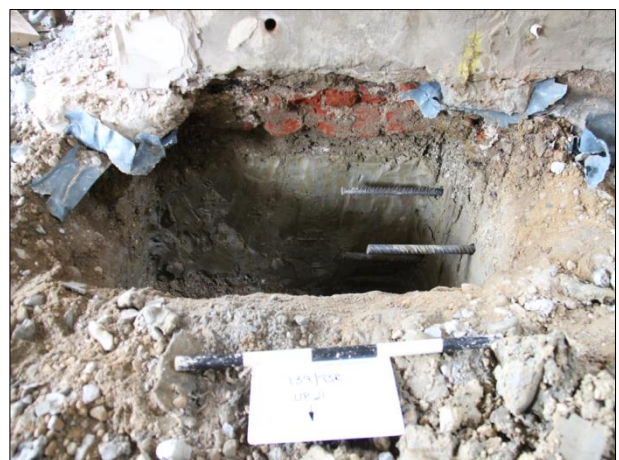
Plate 12: Internal wall footings
