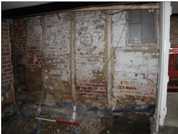
Plate 15: Studwork and window in the north wall of G1
