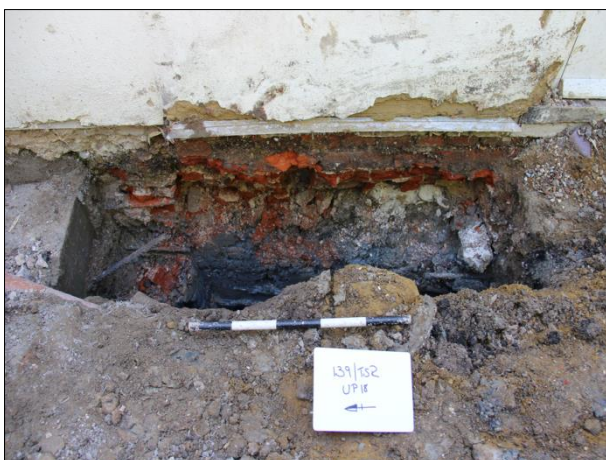
Plate 11: Footings of the western external wall
