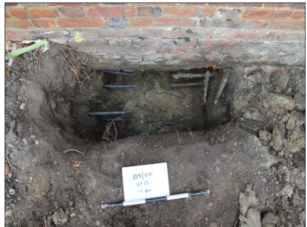
Plate 10: Brickwork in the eastern external wall
