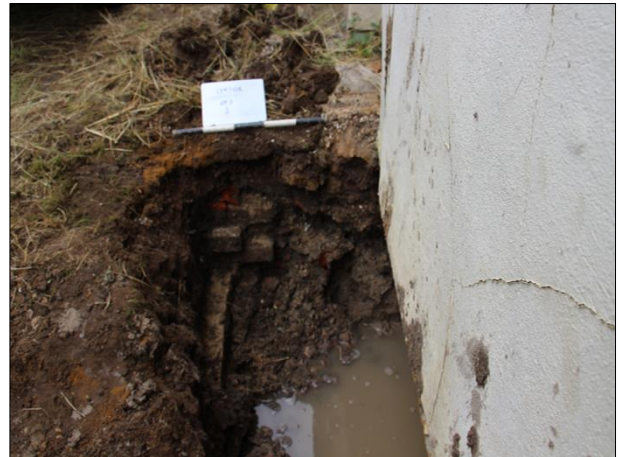
Plate 8: Culvert, facing north
