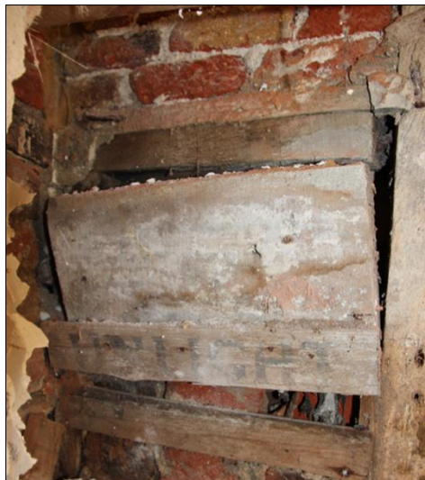
Plate 21: Wooden packing in the north wall of Room G1
