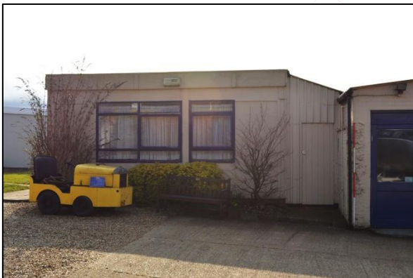
Plate 30: Shot 31. North elevation of crew room
