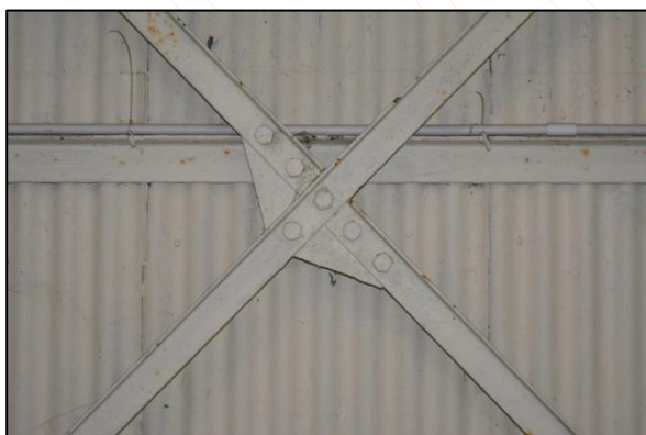
Plate 13: Shot 11. Structural detail, southeast corner
