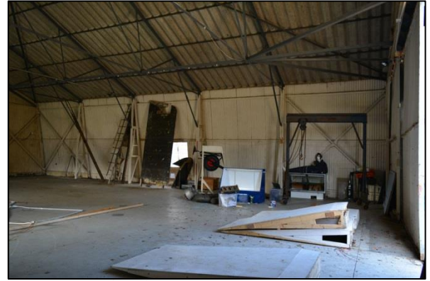
Plate 16: Shot 14. North wall from the southeast
