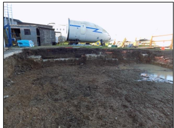
Plate 55: Original Hangar Wall, looking southwest
