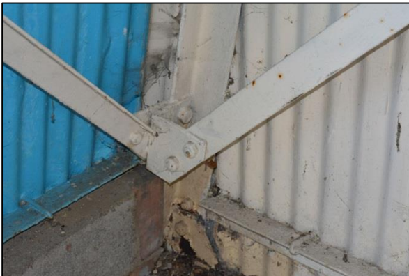
Plate 23: Shot 21. Structural detail in southwest corner
