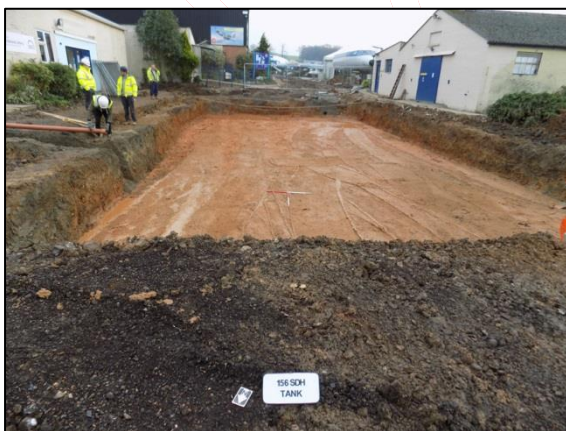
Plate 48: Water Storage Tank, looking south southeast
