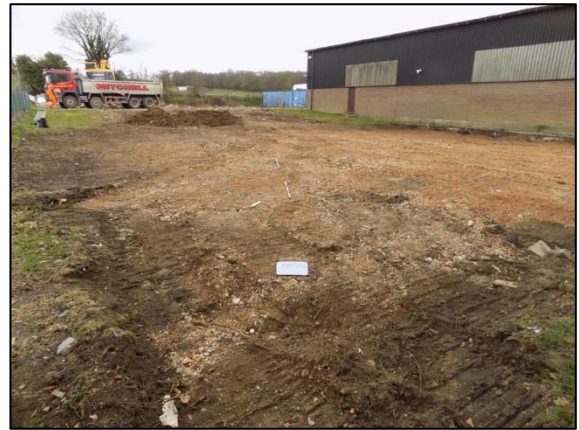
Plate 45: Stripped area for new hangar, looking southwest
