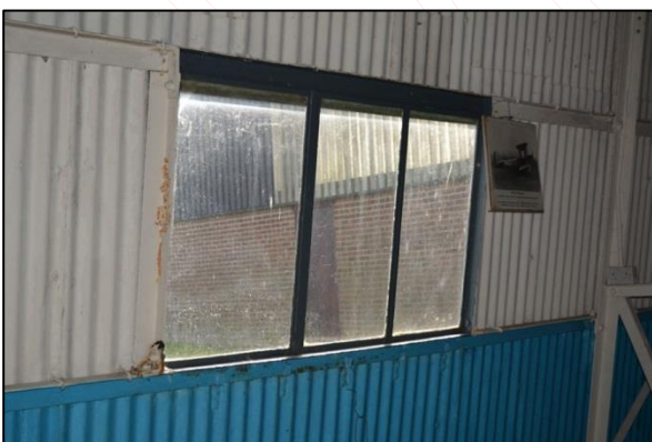
Plate 25: Shot 23. Window detail on south wall
