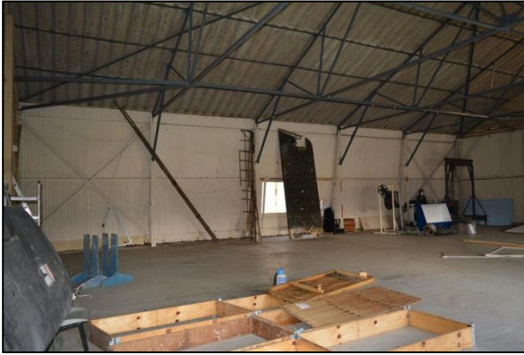
Plate 15: Shot 13. North wall from the southwest
