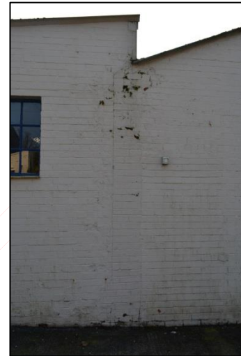
Plate 38: Shot 40. Point of extension on the north elevation
