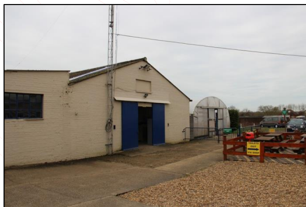
Plate 36: Shot 43. North elevation of the Workshop
