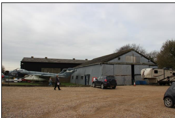
Plate 1: Shot 41. Robin Hangar from the east
