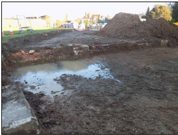
Plate 56: Original Hangar wall, looking northwest
