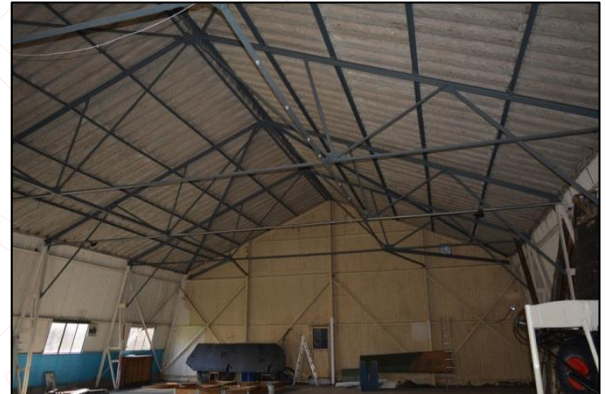
Plate 18: Shot 16. Roof structural detail
