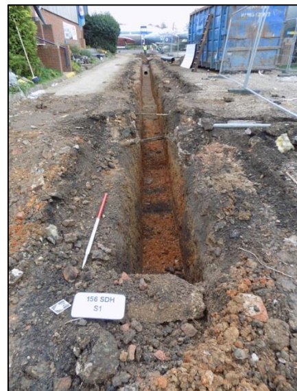
Plate 49: Service Trench 1, looking southeast
