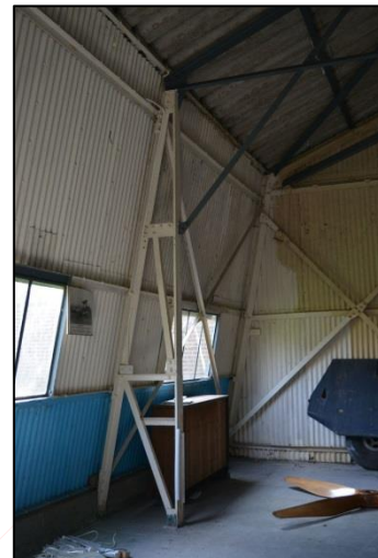
Plate 28: Shot 26. Structural detail south wall
