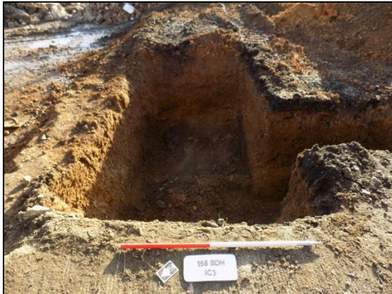
Plate 50: Inspection Chamber 3, looking southeast
