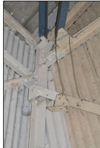
Plate 22: Shot 20. Structural detail in southwest corner
