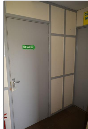
Plate 35: Shot 37. North wall of hallway
