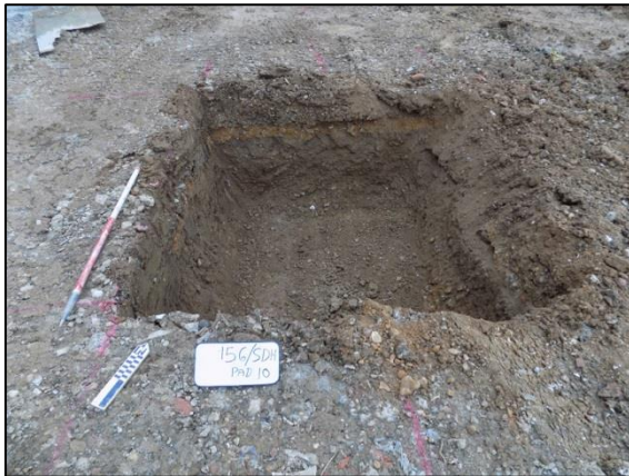
Plate 46: Pad of new hangar (Pad 10), looking north northwest
