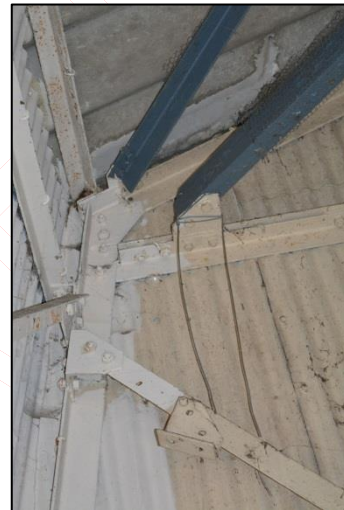
Plate 24: Shot 22. Structural detail in southwest corner
