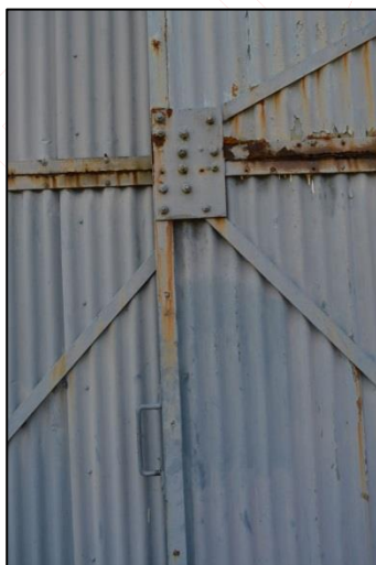
Plate 7: Shot 28. Detail on east elevation of hangar
