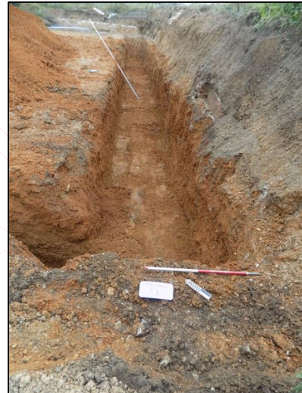
Plate 47: Footing Trench 1, looking northeast
