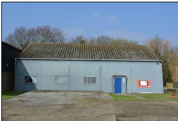
Plate 3: Shot 1. South elevation of hangar
