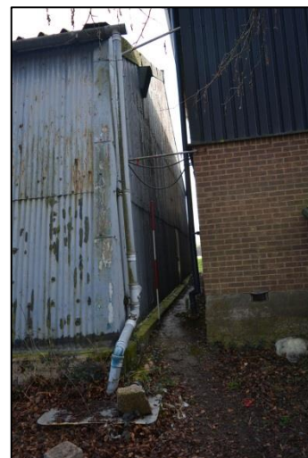
Plate 8: Shot 7. Northwest corner of hangar
