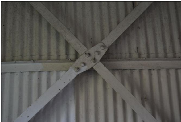
Plate 21: Shot 19. Structural detail west wall
