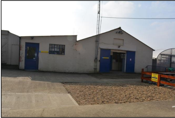
Plate 37: Shot 30. North elevation of the History Centre and Workshop
