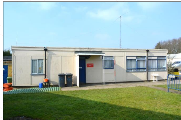
Plate 31: Shot 32. East elevation of crew room
