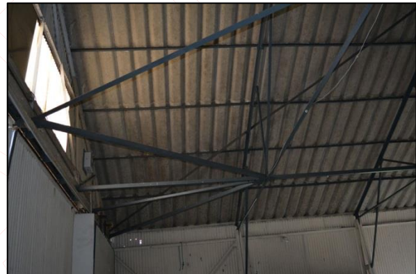
Plate 12: Shot 10. Roof detail, southeast corner
