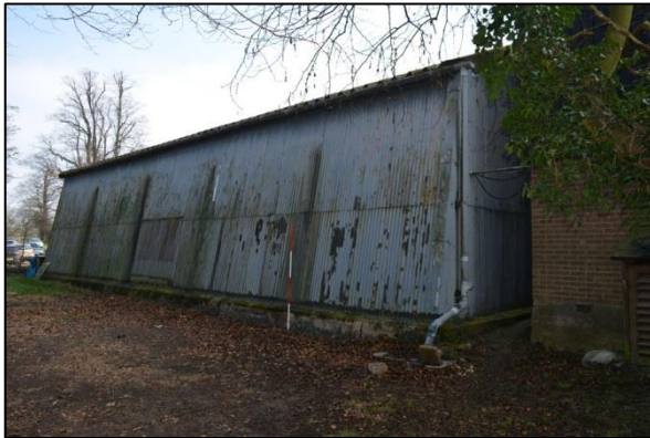
Plate 9: Shot 6. North elevation of hangar
