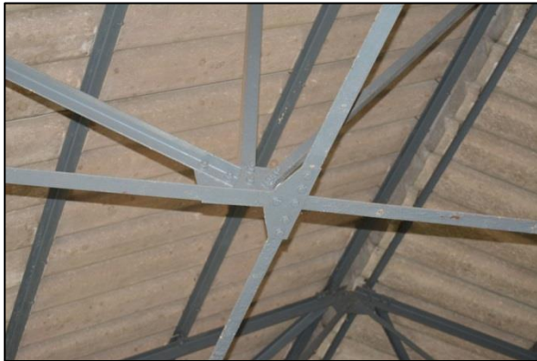
Plate 27: Shot 25. Roof structural detail
