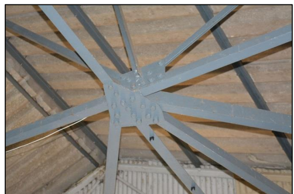
Plate 26: Shot 24. Roof structural detail
