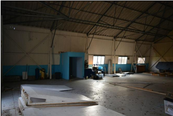
Plate 17: Shot 15. South wall from the northeast
