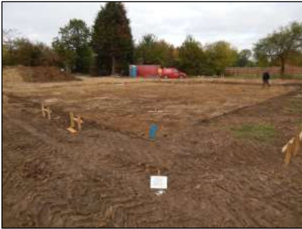
Plate 1: Ground reduction facing NW (1x1m scale)
