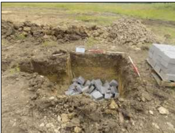
Plate 3: Soakaway facing SE (1x1m scale)
