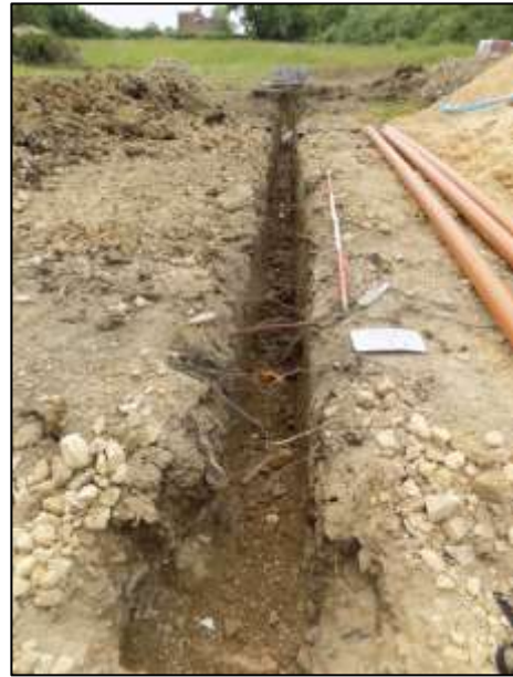
Plate 2: Trench 1 facing SW (1x1m scale)
