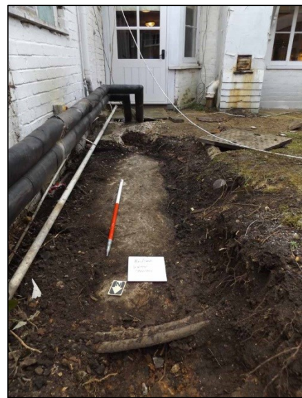
Plate 16: Water storage chamber, looking S (1m scale)
