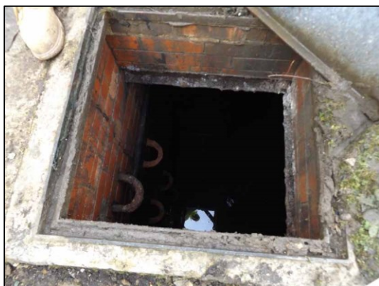
Plate 17: Inside view of water storage chamber
