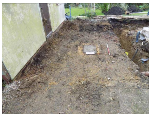
Plate 3: General view with modern culvert, facing east (scale 1m)
