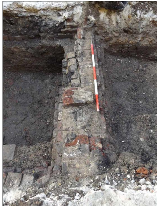
Plate 10: Brick wall [112], facing west, with 1m scale
