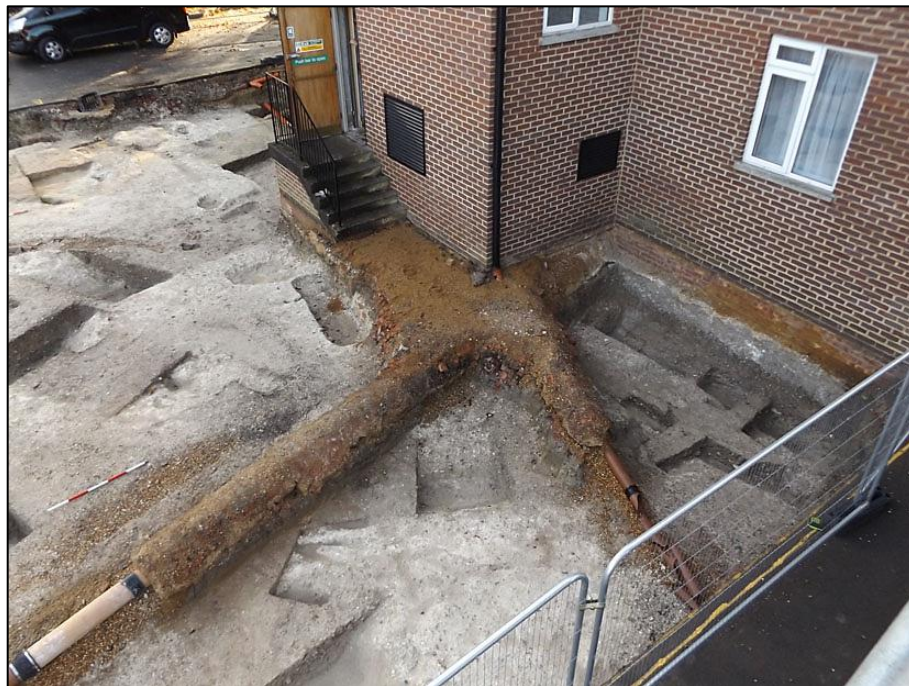
Plate 55: Strip, Map and Sample area, post-excavation, looking SE (1m scale)
