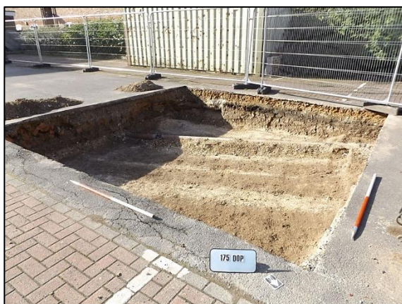
Plate 5: Soakaway, pre-excitation, looking SW (2x1m scale)
