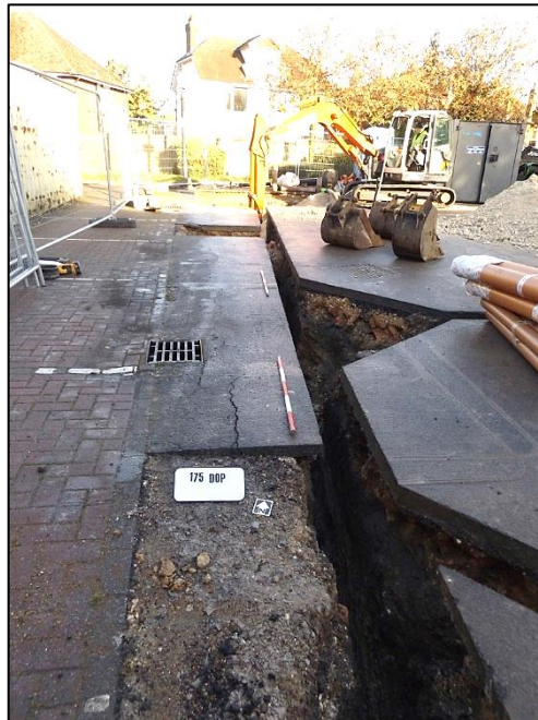
Plate 7: Service trench, looking N (2x1m scale)
