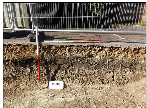
Plate 6: General stratigraphy of soakaway, looking SW (2x1m scale)
