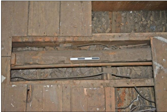
Plate 7: Re-used timber used as a joist in Room F2
