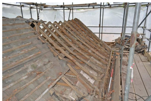
Plate 16: View of the stable roof from the southwest
