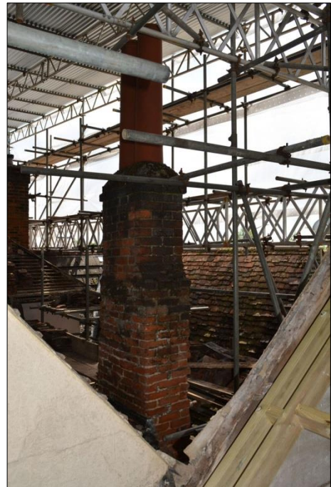
Plate 22: Chimney stack for G6/F8
