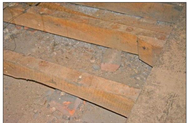
Plate 4: Joists in Room G2
