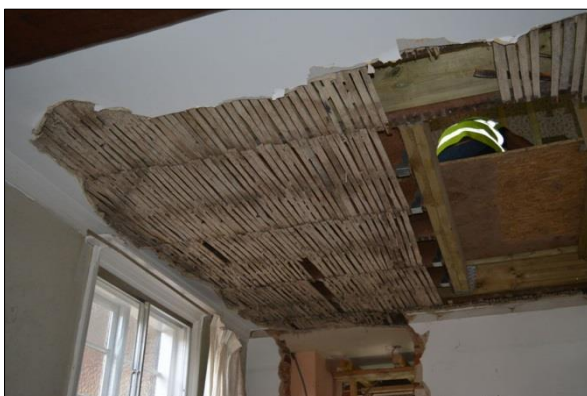
Plate 11: Lath & plaster ceiling in Room G5
