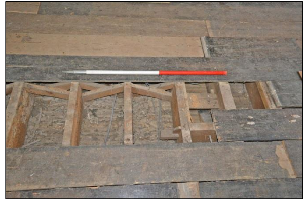
Plate 8: Diagonal bracing and tusk tenon in Room F7
