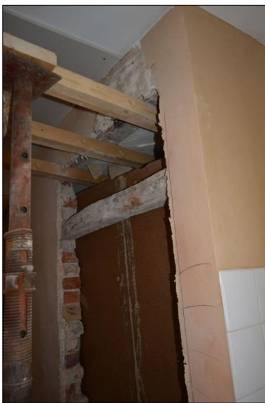
Plate 3: Bonding beam and exposed brickwork in Room F5
