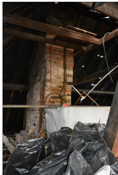
Plate 20: Chimney at the northern end of the main range
