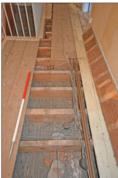
Plate 5: Joists in the landing (F1)
