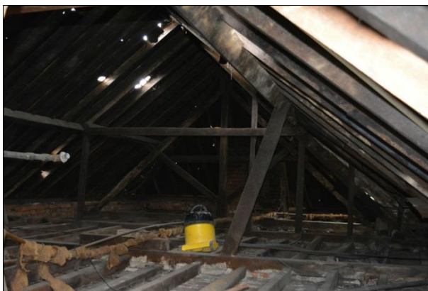
Plate 19: Roof over the main range looking south
