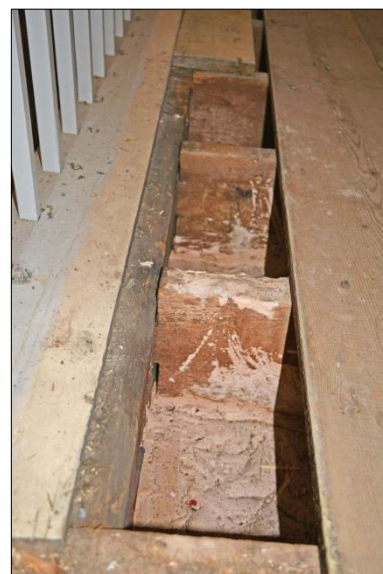
Plate 6: Detail of central tenons
