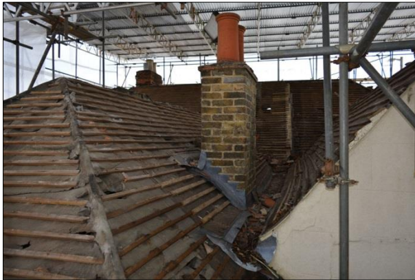
Plate 21: Roof over northern extensions looking east
