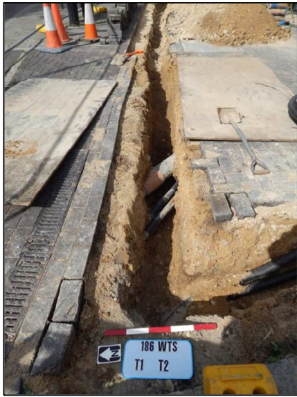
Plate 1: Trench 1, looking east
