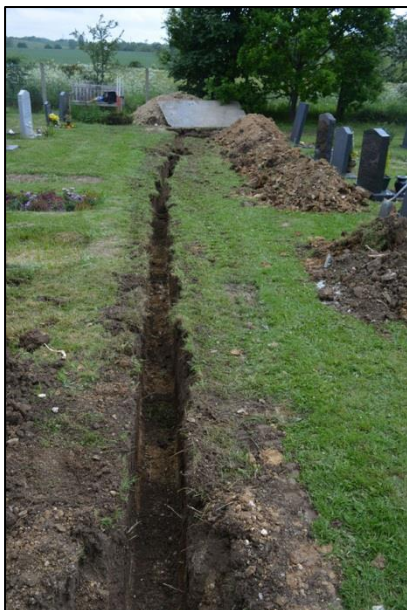
Plate 5: Trench 2, facing NW.
