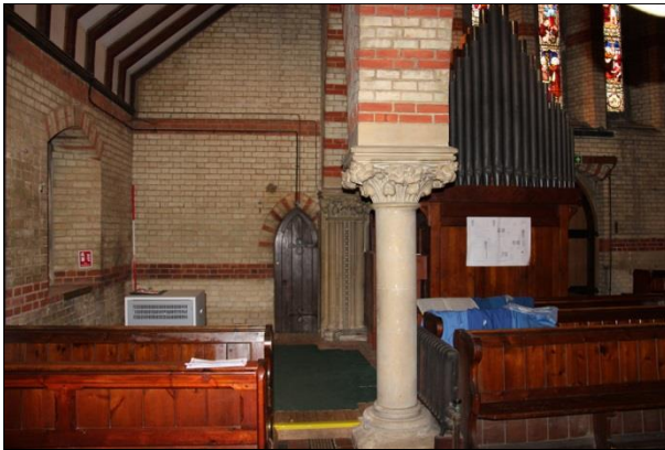
Plate 7: Southwest corner of the nave
