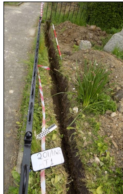
Plate 4: Trench 1 northwest end, facing SE.
