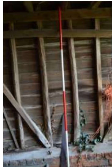
Plate 8: Onion Shed: adzed studs in the east wall
