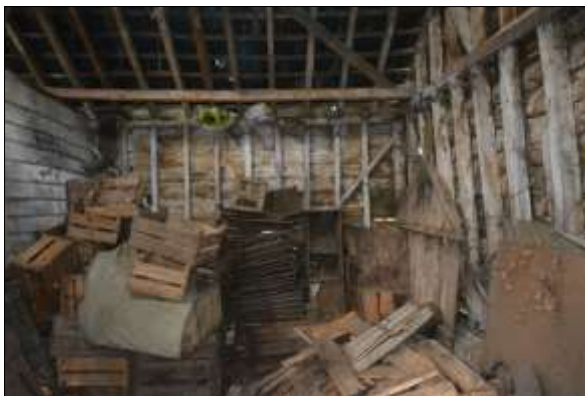
Plate 27: Stable: north wall
