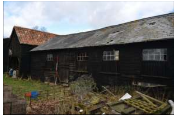
Plate 14: Cowshed: from the southeast
