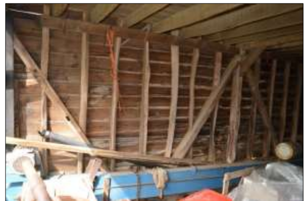
Plate 10: Onion Shed: southern end of west wall
