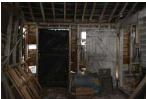
Plate 29: Stable: south wall
