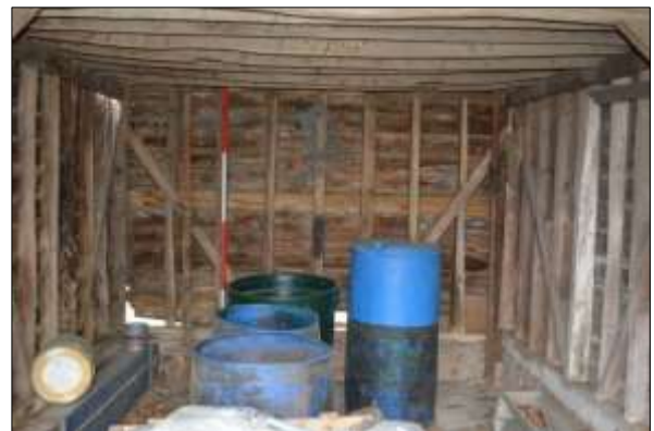
Plate 4: Onion Shed: north wall
