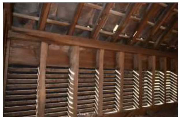
Plate 12: Onion Loft: louvre detail
