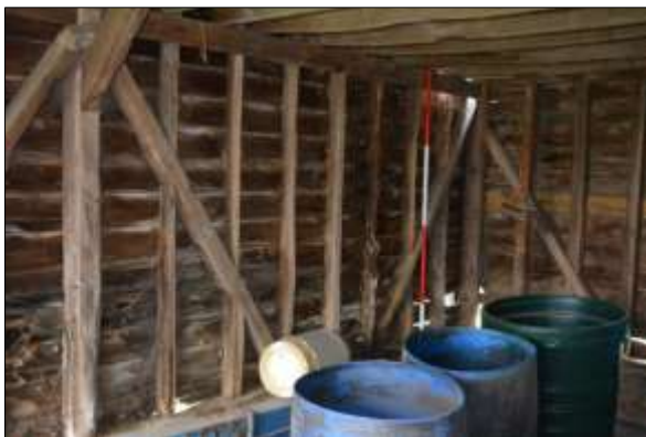
Plate 9: Onion Shed: northwest corner
