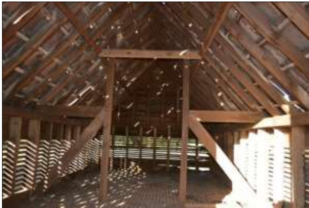
Plate 13: Onion Loft: queen post truss
