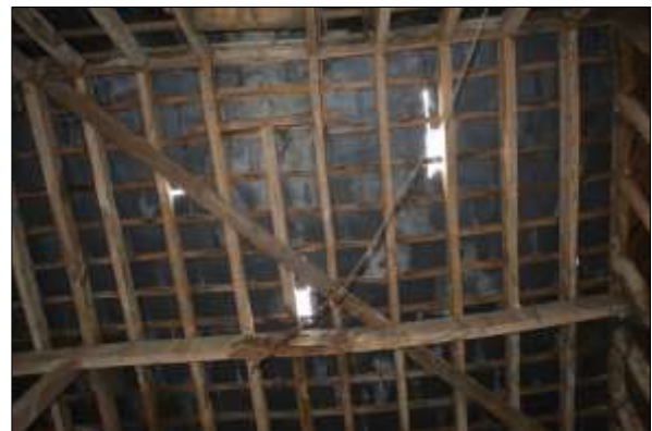
Plate 28: Stable: roof detail
