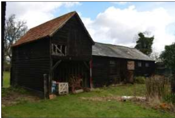
Plate 1: Onion Shed & Cowshed/Stable from the southwest
