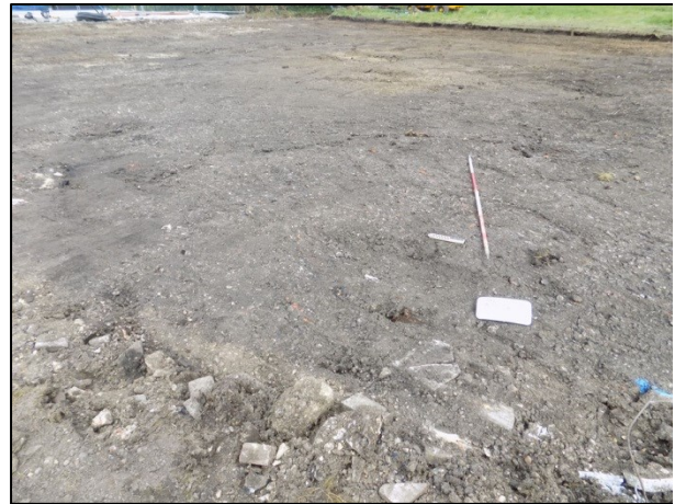
Plate 2: Ground reduction general view facing west (2m scale)
