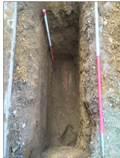
Plate 4: Shot 31. Section of trench showing brick vault.
