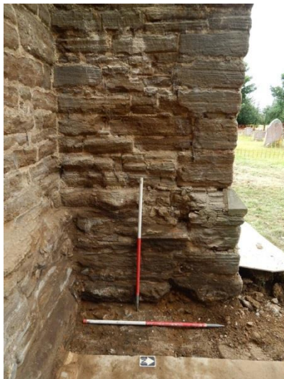
Plate 3: Shot 4. Detail shot of tower buttress repair.
