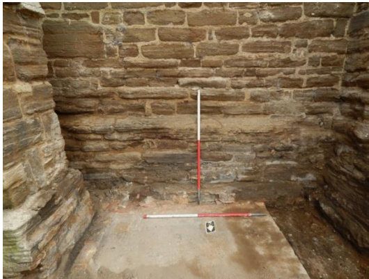
Plate 1: Shot 2. East facing wall of tower following boiler house demolition.
