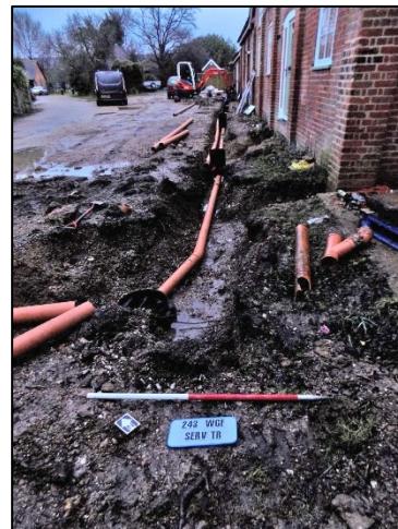
Plate 4: Drainage trench to the south, looking east
