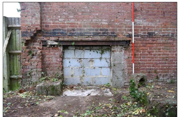
Shot 6: West elevation, bricked up opening
