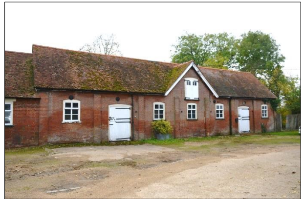
Shot 2: North elevation, building 2
