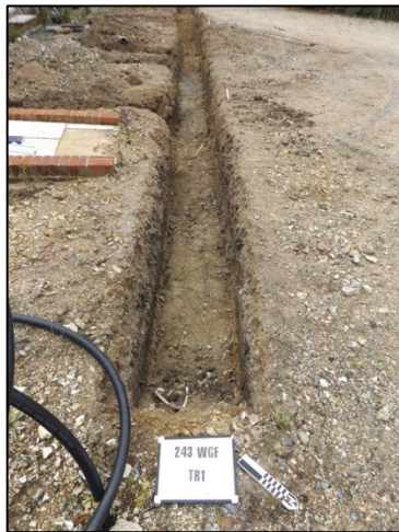
Plate 7: External Service Trench (EST) 1, looking SW
