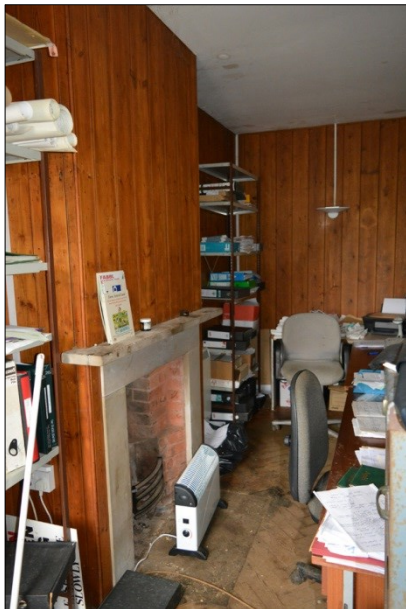
Shot 12: Room 2 looking south
