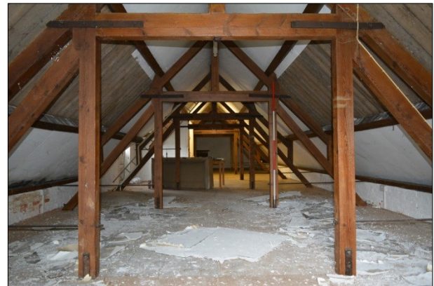
Shot 30: First floor looking east
