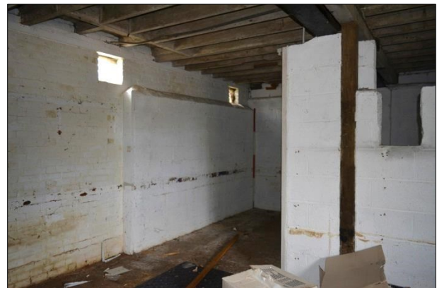
Shot 26: Room 4 south wall
