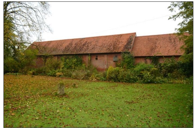
Shot 8: South elevation from the southeast
