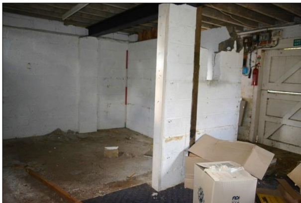
Shot 25: Room 4 northwest corner
