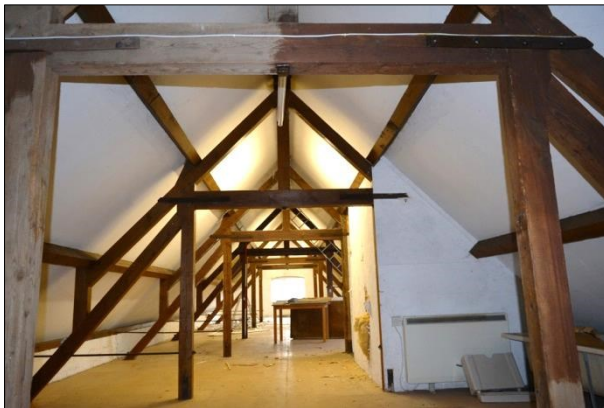
Shot 29: First floor looking west
