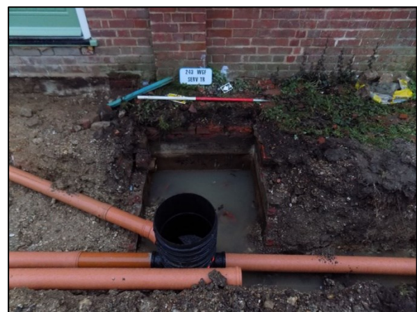
Plate 6: Detail of sump to the south of the building
