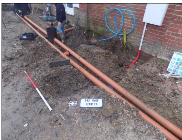
Plate 5: Detail of drainage trench to the south, looking southeast
