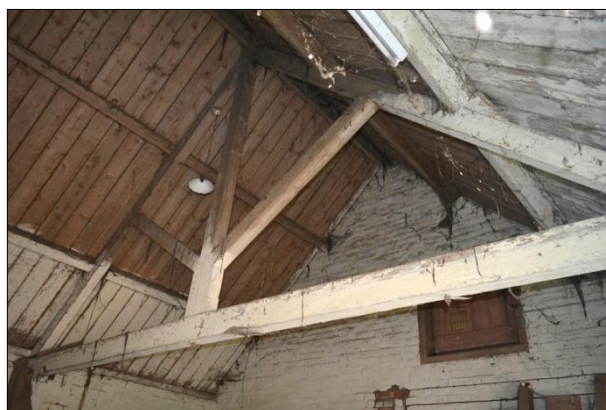
Shot 17: Room 3 roof detail
