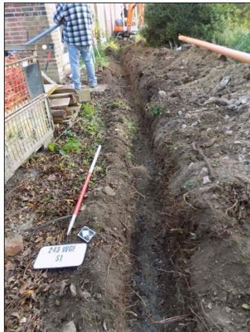
Plate 1: Trench to the rear of the building, view to east
