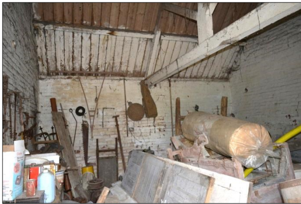
Shot 15: Room 3 southeast view
