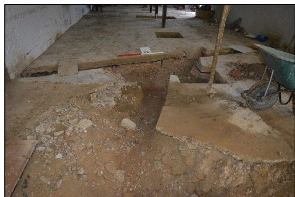
Plate 18: General view of the internal groundworks, looking west
