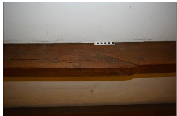
Shot 32: Detail of Trait de Jupiter scarf joint
