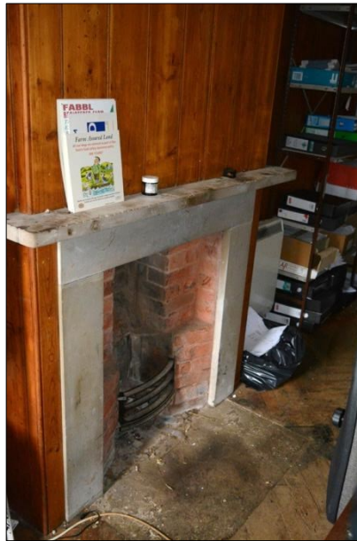
Shot 14: Room 2 fireplace detail
