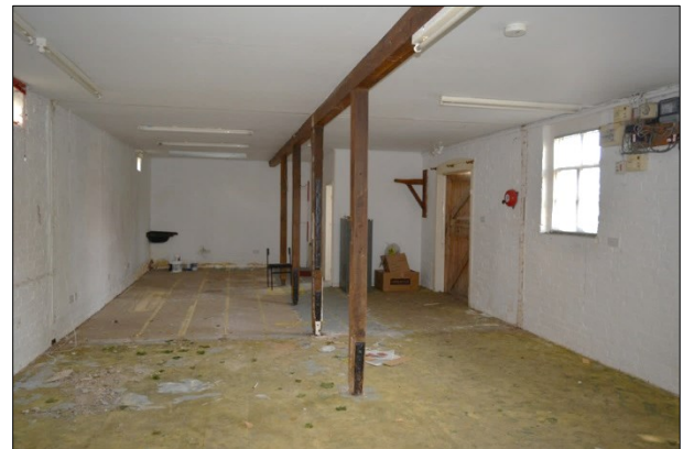
Shot 19: Room 5 looking west
