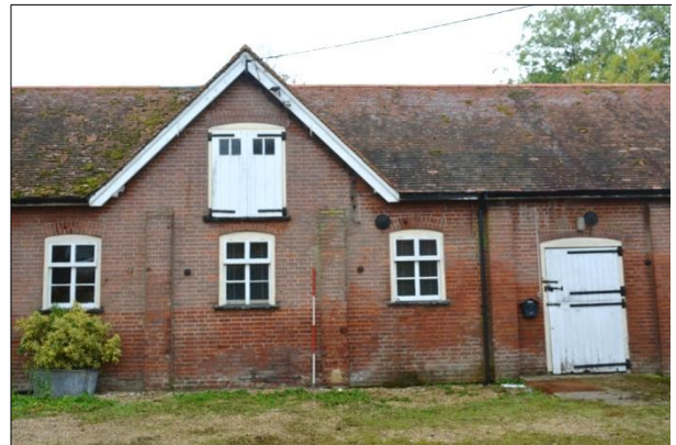
Shot 4: Close up of building 2 gable
