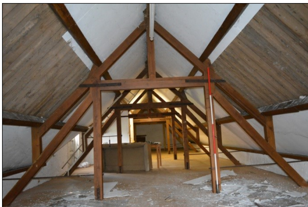
Shot 31: First floor roof structure
