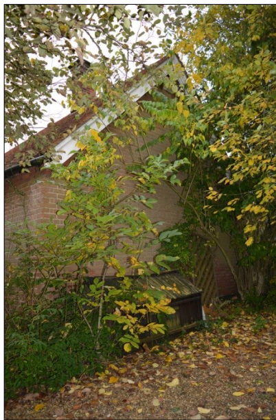
Shot 10: East elevation from the southeast
