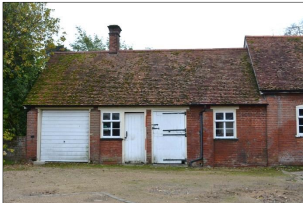
Shot 3: North elevation, building 1
