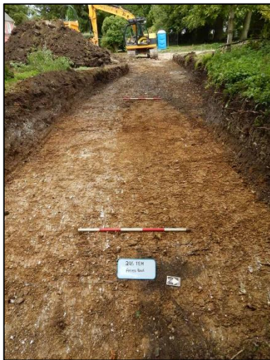
Plate 3: Final access road, looking W (1m scale)
