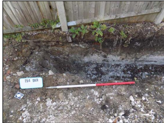
Plate 4: Garage footing trench, stratigraphy, looking SW (1m scale)
