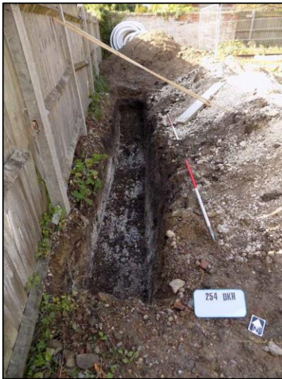
Plate 3: Garage footing trench, looking NNW (2 x 1m scale)
