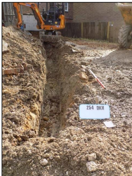
Plate 5: Service trench, looking S (1m scale)
