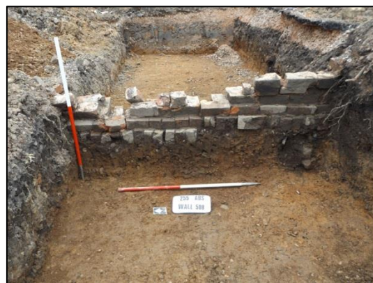
Plate 23: Trench 5, brick wall [508], gully [G527] & pit [522], looking ESE (2x1m scale)
