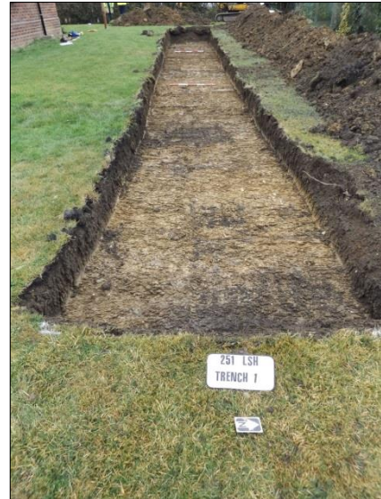
Plate 2: Trench 1: view to west
