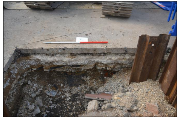
Plate 2: West facing section of the pit prior to shuttering
