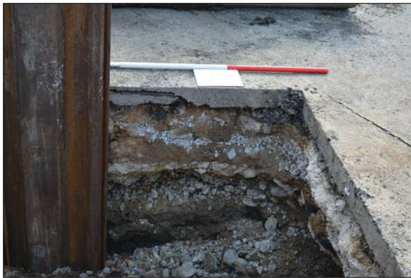
Plate 1: North facing section of the pit prior to shuttering
