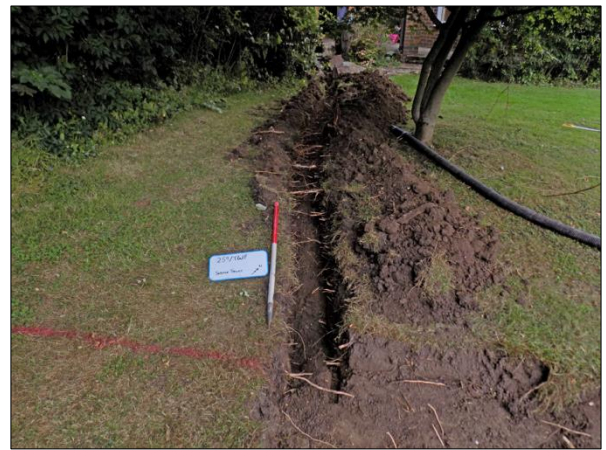
Plate 4: Service trench, facing north
