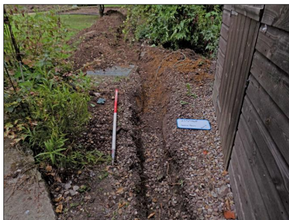
Plate 5: Service trench, facing south
