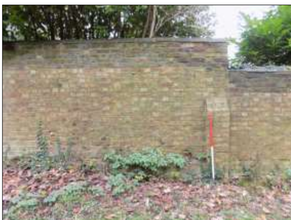
Plate 17: Perimeter wall, location of Test Pit 8
