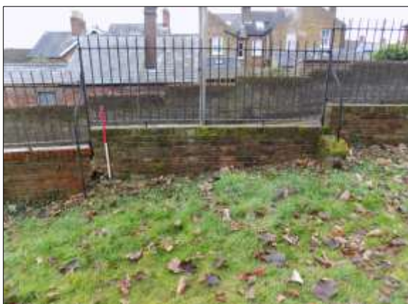
Plate 5: Junction of old and new wall, location of Test Pit 3
