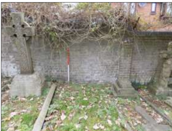
Plate 15: Oldest wall, location of Test Pit 7
