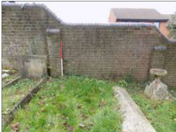
Plate 13: West wall, upper cemetery, location of Test Pit 6
