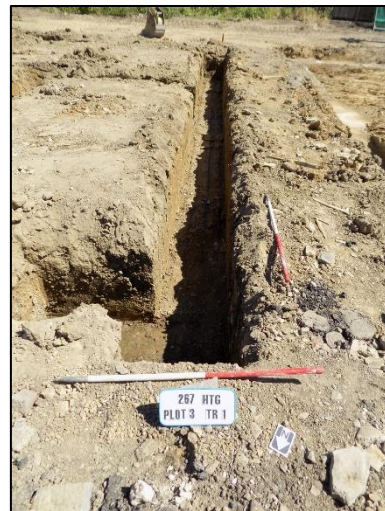
Plate 20: Plot 3, trench 1, looking SSE
