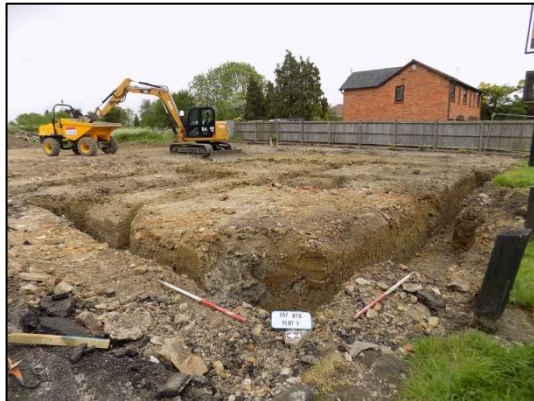
Plate 1: Plot 1 footing trenches, looking E
