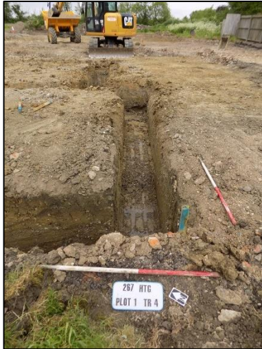
Plate 5: Plot 1, trench 4, looking NE
