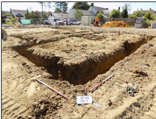
Plate 19: Plot 3, footing trenches, looking W
