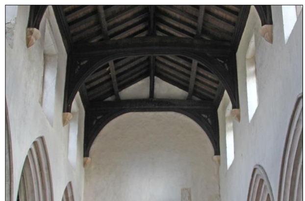
Plate 14: Nave roof, view east
