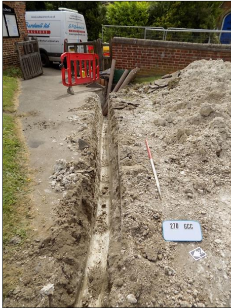
Plate 22: Man-hole and service trench underlying church pathway, view SE
