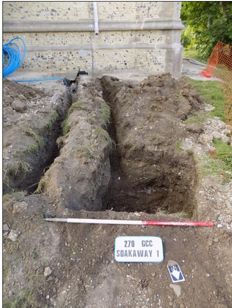
Plate 30: Soakaway 1, view SSW
