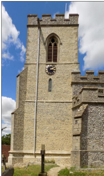
Plate 3: South side of tower after works, view north
