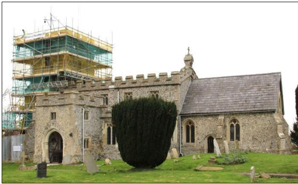
Plate 1: Tower and south side during works, view north-northeast
