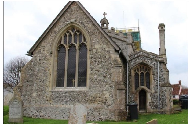
Plate 4: East front of the church and vestry, view west
