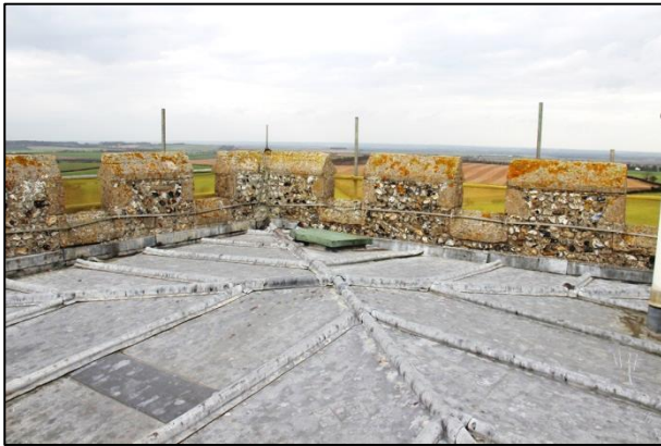
Plate 7: Tower roof and parapets, view northwest
