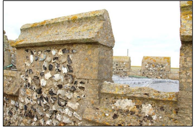
Plate 8: Tower parapets, view north
