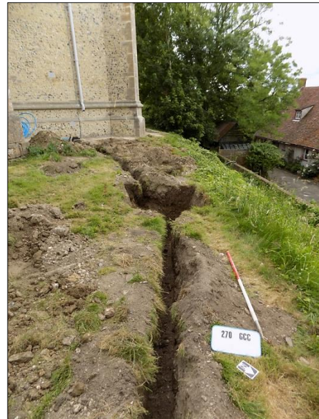
Plate 27: Service trench through churchyard, view SW (pump trench also shown)
