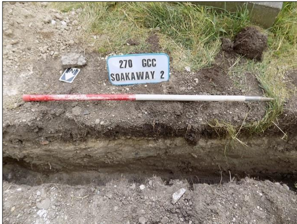
Plate 34: Pipe trench for Soakaway 2, view SSE
