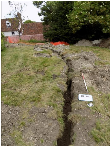
Plate 26: Service trench through churchyard, view NW
