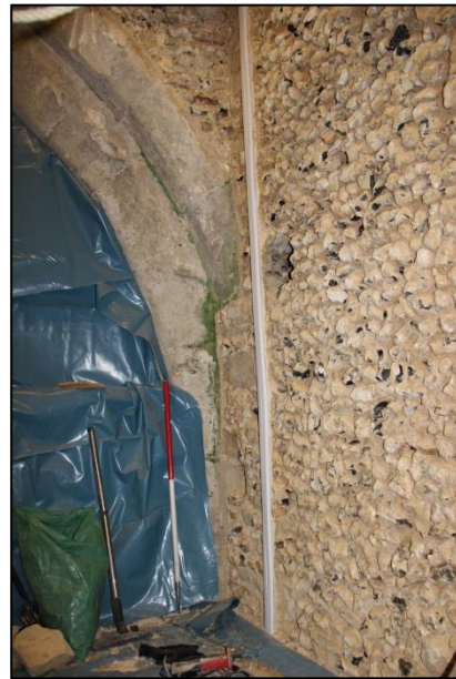
Plate 16: Tower: internal flint wall, view southeast
