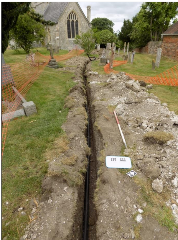
Plate 24: Service trench through churchyard, view NW
