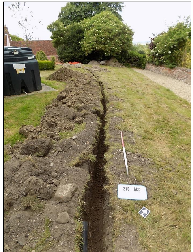
Plate 25: Service trench through churchyard, view NW
