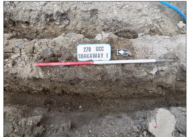
Plate 31: General stratigraphy of pipe trench for Soakaway 1, view E
