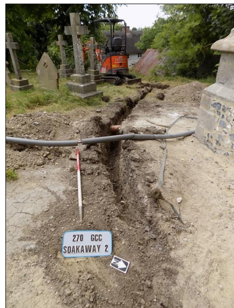
Plate 33: Soakaway 2, view WSW
