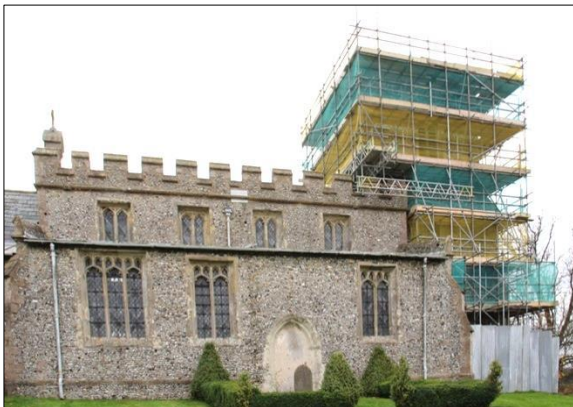
Plate 5: Tower and south side during works, view south
