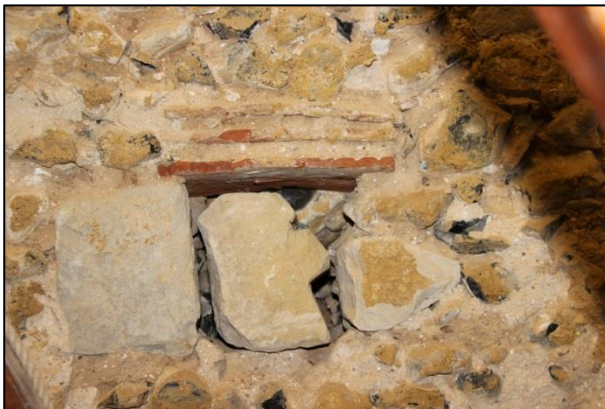
Plate 17: Tower: put-log hole, view north
