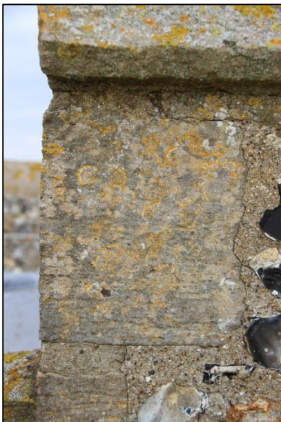
Plate 9: Tower parapet detail, view north
