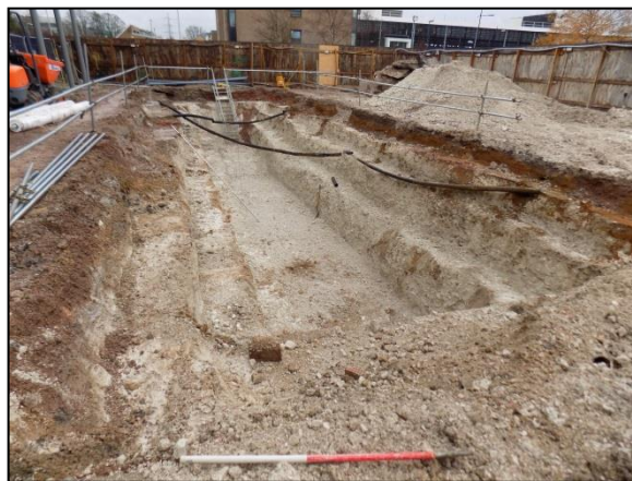
Plate 8: Attenuation tank, looking northeast
