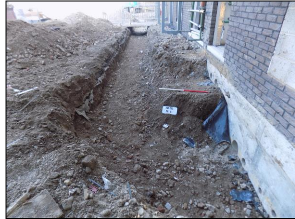
Plate 7: Service trench to the northwest of the new building, looking northeast
