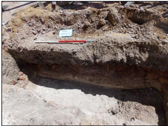
Plate 6: Percolation test pit
