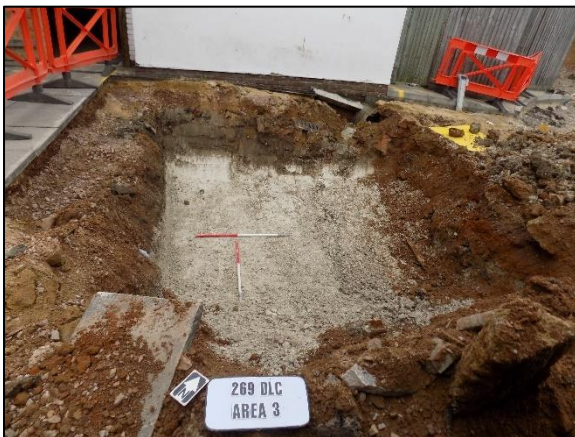
Plate 3: Area 3, looking northwest
