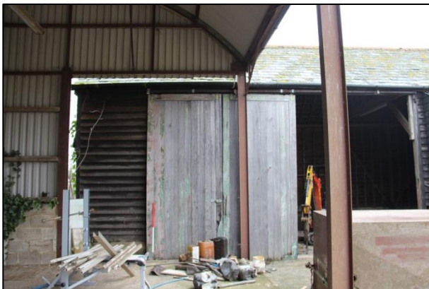
Plate 5: West elevation, northern end
