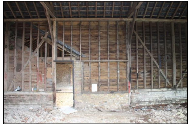
Plate 14: East wall, Bay 2
