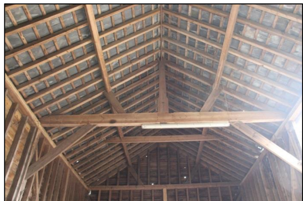
Plate 24: Barn roof detail, facing south
