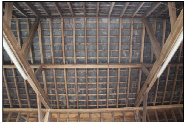
Plate 20: Barn roof detail, facing east
