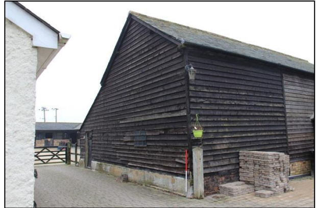
Plate 10: South elevation, facing northwest
