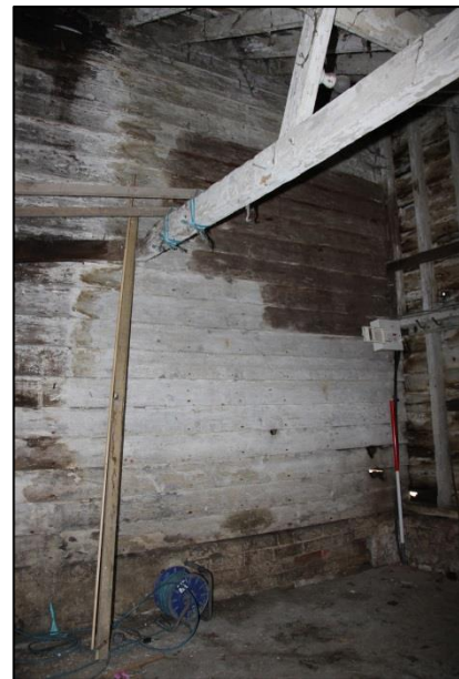
Plate 28: Workshop, southeast corner
