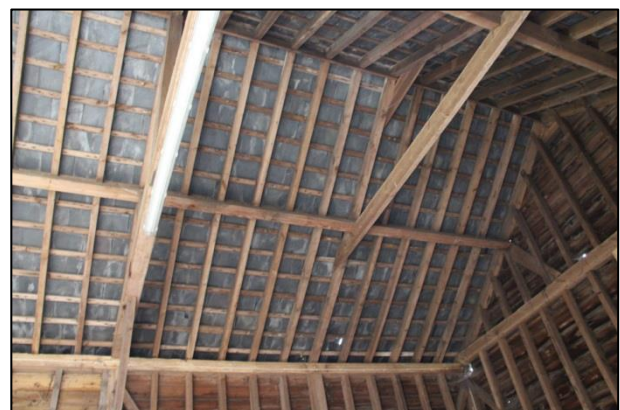
Plate 18: Barn roof detail, facing southeast
