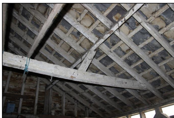
Plate 33: Workshop roof detail, facing south
