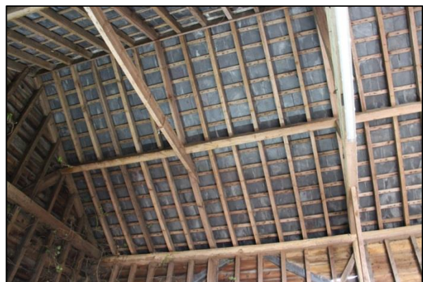
Plate 22: Barn roof detail, facing northeast
