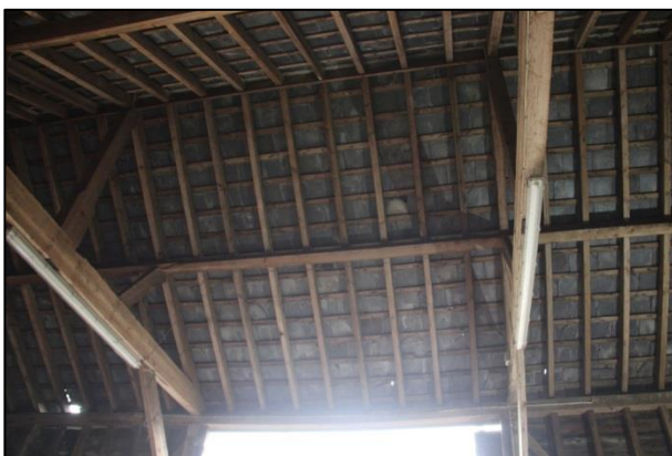
Plate 21: Barn roof detail, facing west
