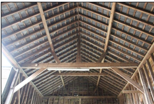
Plate 23: Barn roof detail, facing north
