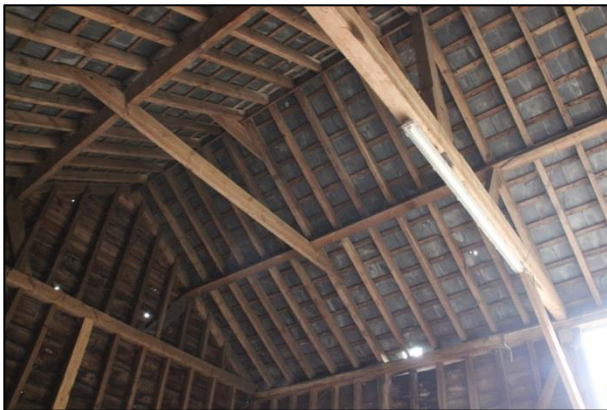
Plate 19: Barn roof detail, facing southwest
