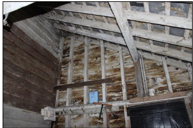
Plate 30: Workshop roof detail, facing southeast
