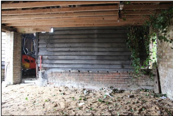
Plate 3: East elevation inside car port
